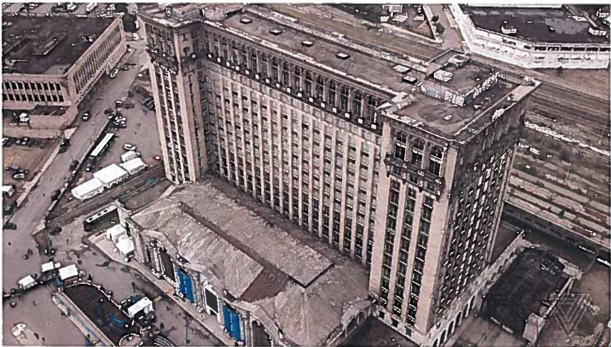
Aerial view of the Michigan Central Station 45
