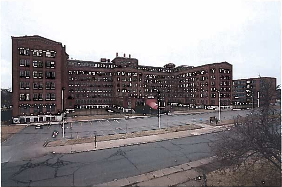
Herman Kiefer Hospital complex
