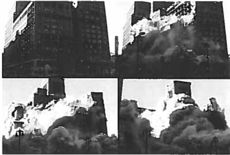
Controlled demolition of the Hudson's Department store at 5:45 p.m. on Oct. 24, 1998 23
