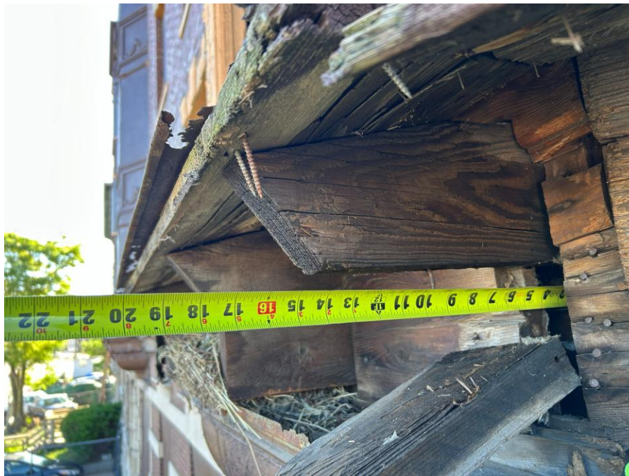
Typical Window Bay Framing Condition at Manhattan Building
