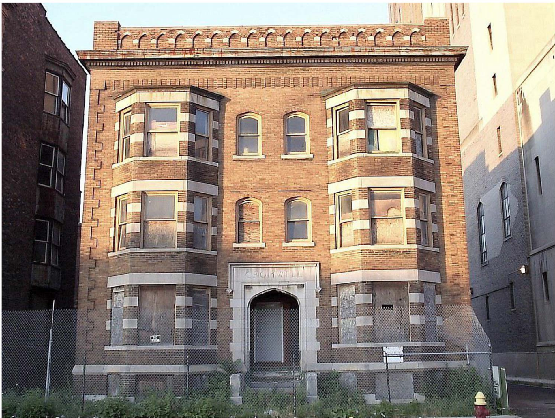
CROMWELL WEST (2ND AVENUE) FACADE *PRE-BOARDING OF WINDOWS
