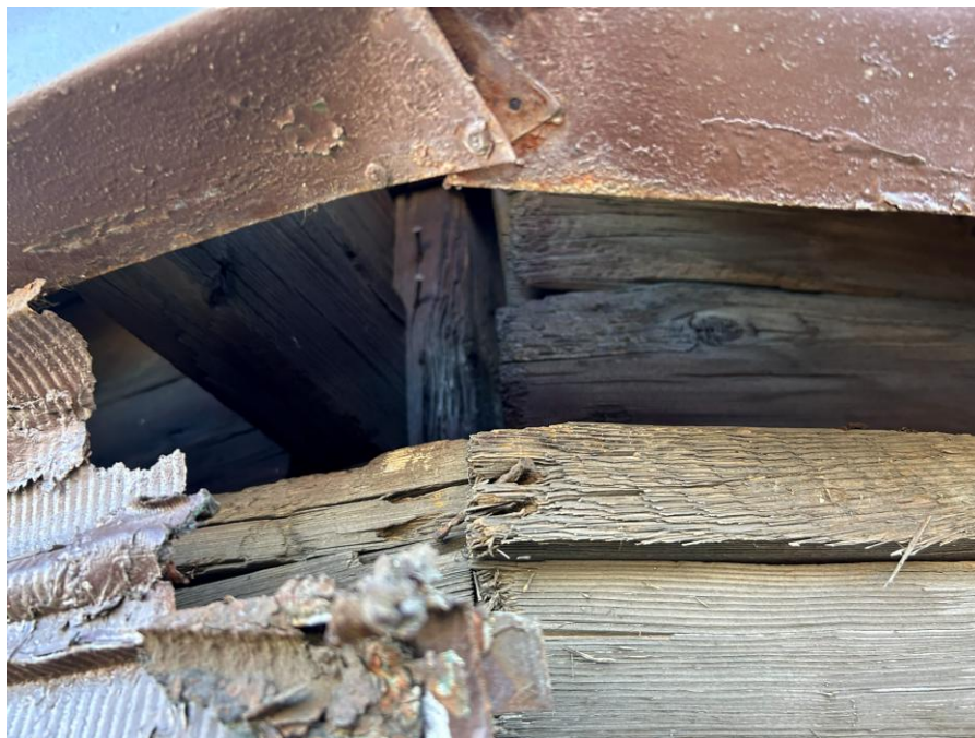
Typical Window Bay Framing Condition at Altadena Building
