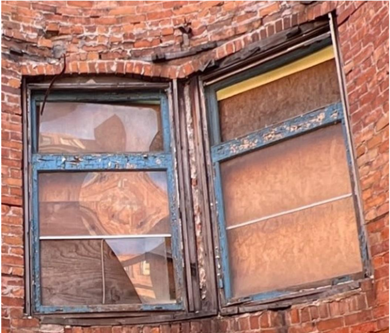
EXISTING WINDOWS 3418 JOHN R
