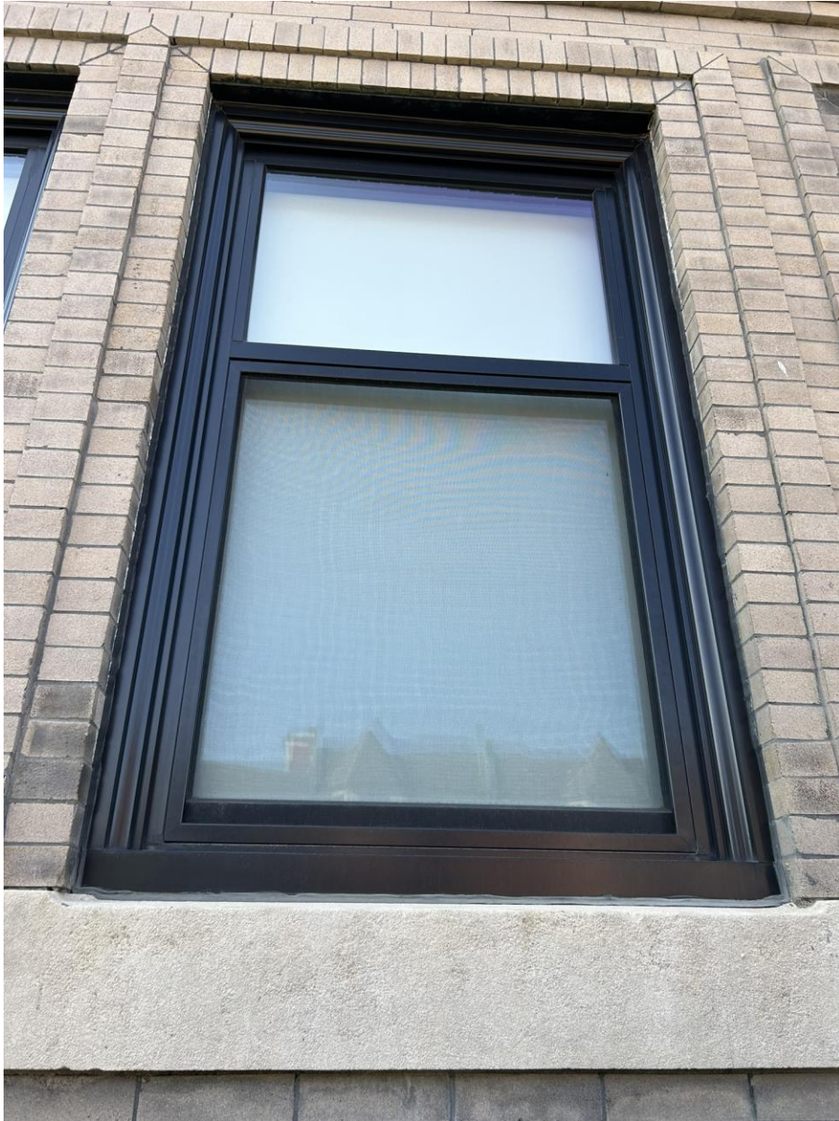
TYPICAL COTTAGE STYLE DOUBLE HUNG ALUMINIUM WINDOW
