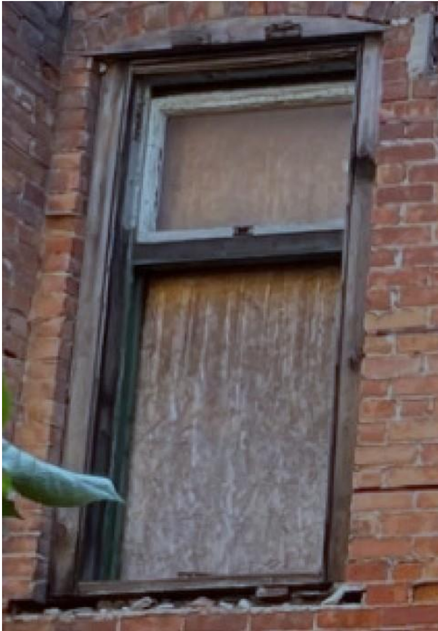
EXISTING WINDOW 3418 JOHN R
