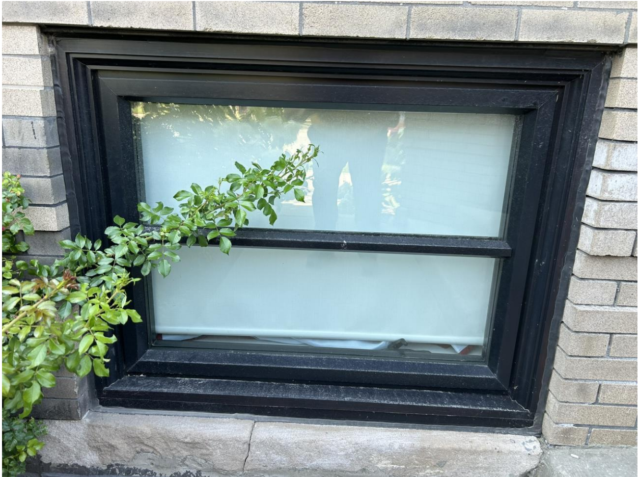
TYPICAL DOUBLE HUNG WINDOW LOCATED IN LOWER LEVEL
