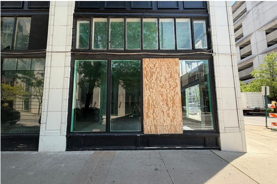
6. Storefront F, North Façade, Looking South.
