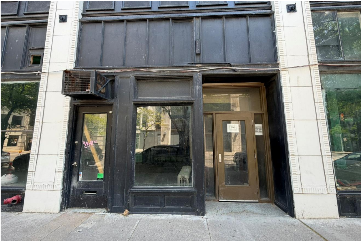
4. Storefront D, North Façade, Looking South.
