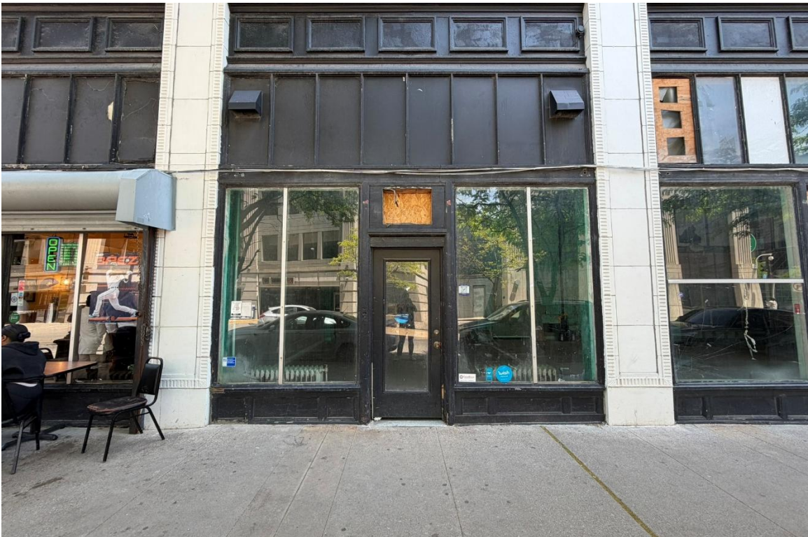
2. Storefront B, North Façade, Looking South.
