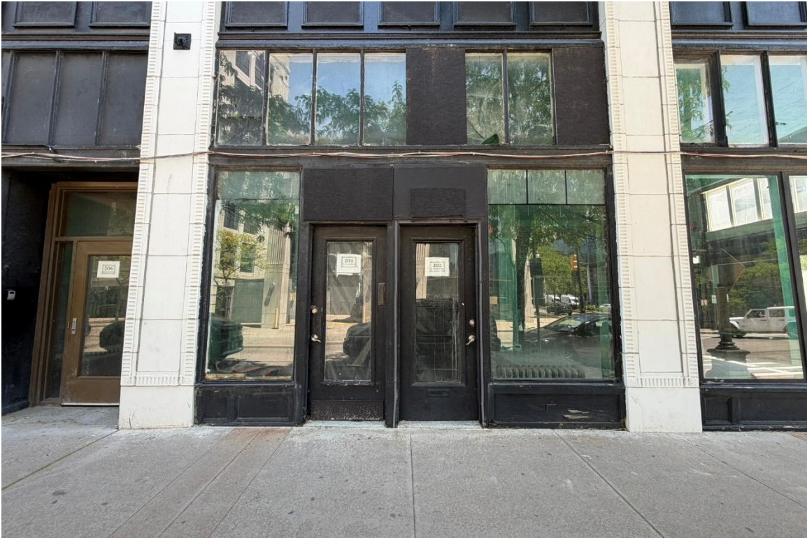
5. Storefront E, North Façade, Looking South.
