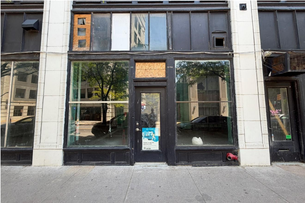
3. Storefront C, North Façade, Looking South.
