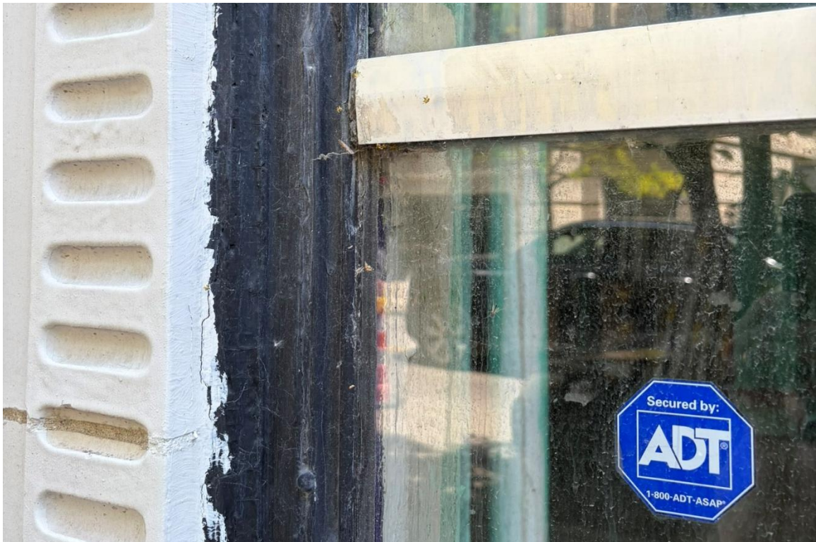
10. Storefront C reglazed, North Façade, Looking South.
