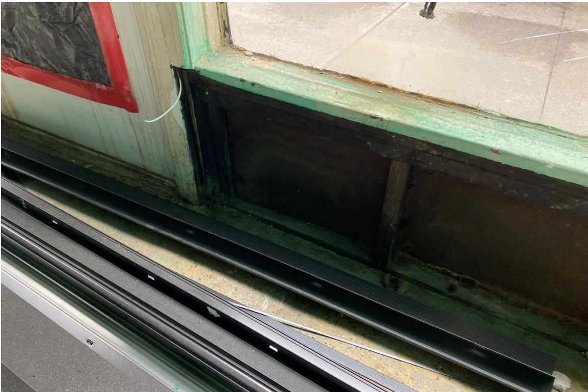
28. . Interior wood structure of storefront, North Façade, Looking North.
