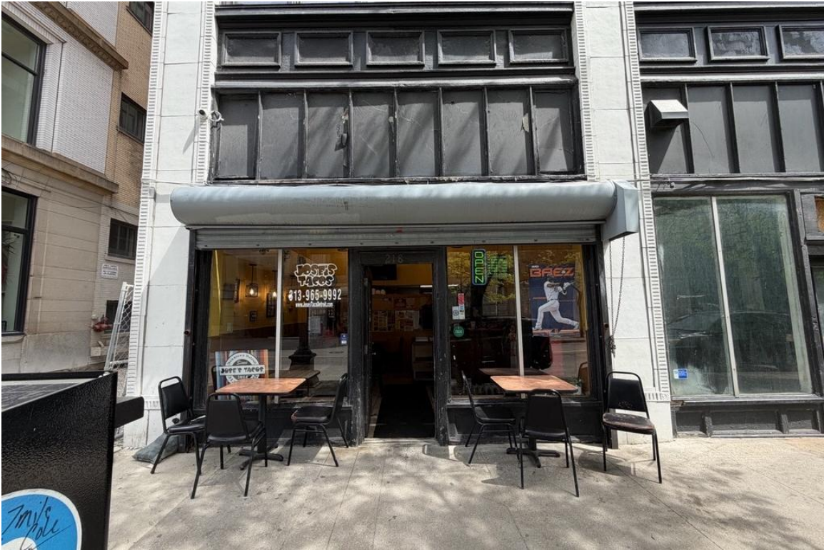
1. Storefront A, North Façade, Looking South.
