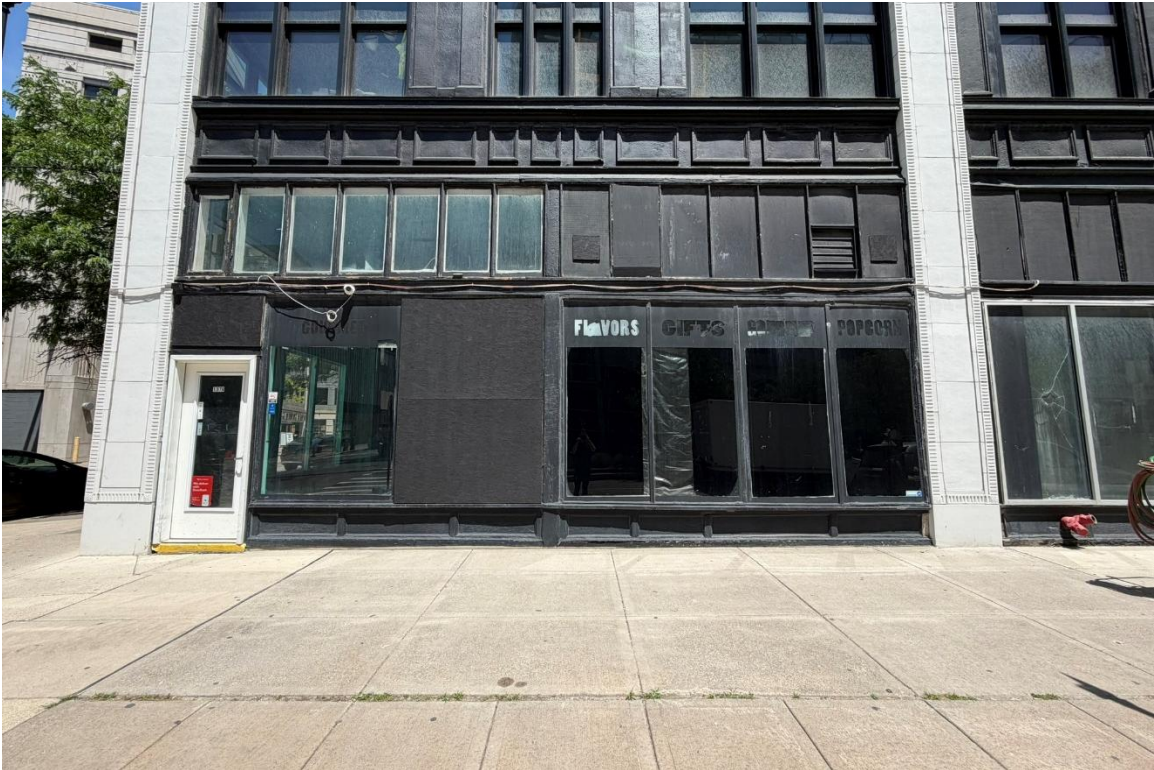
7. Storefront G, West Façade, Looking East.
