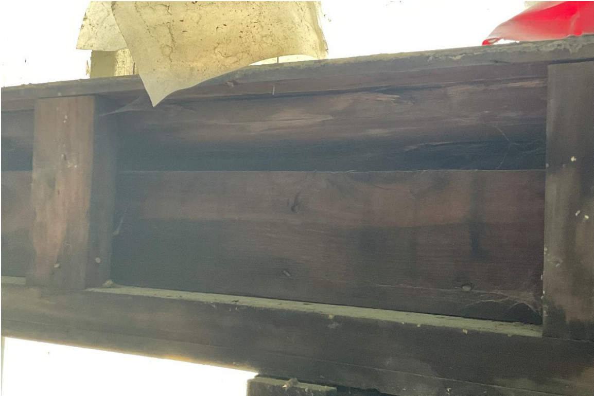
27. Interior wood structure of storefront, North Façade, Looking North.
