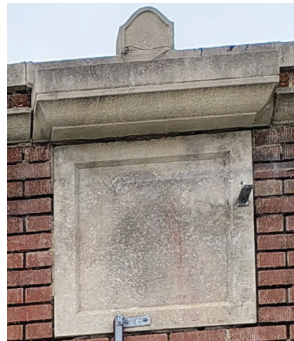
12526 EXISTING STONE TO BE RECLAIMED
