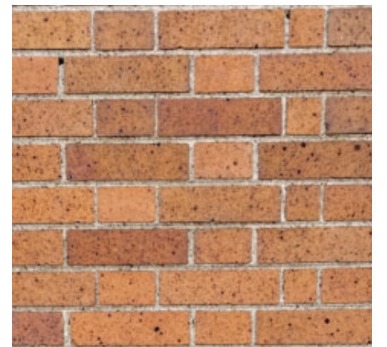
12546 EXISTING BRICK TO REMAIN
