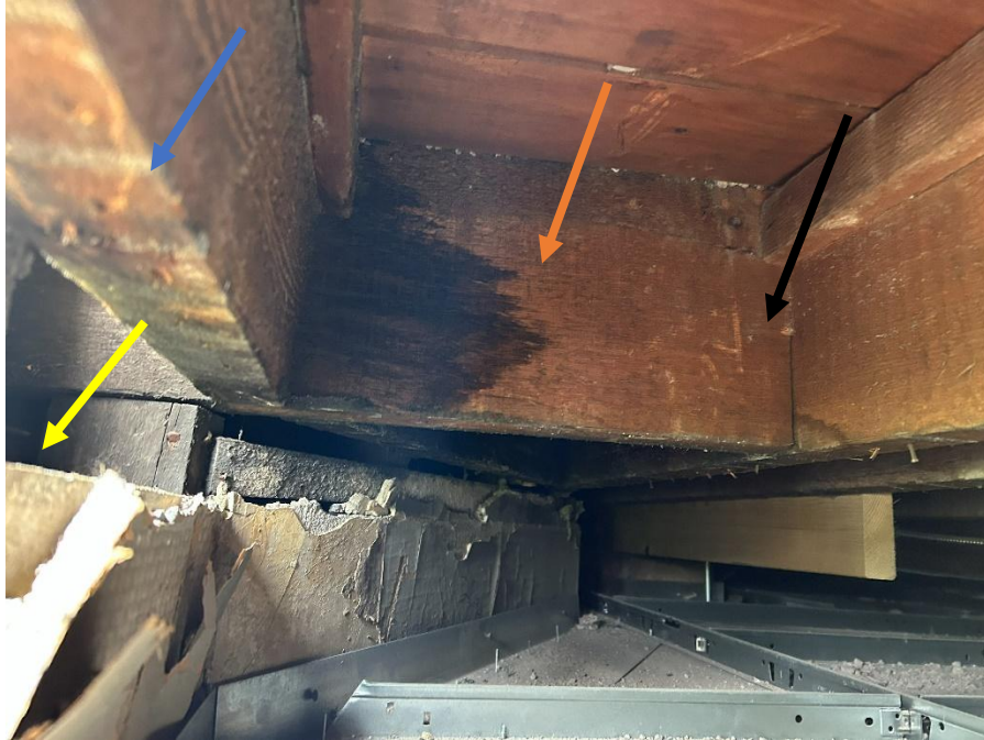
Photo 4: Connection of the north end of the cross-joist member (indicated by the blue arrow) and the perpendicular member (indicated with orange arrow). Member shown with the blue arrow within this photo matches member shown with a blue arrow in Photo 2.
