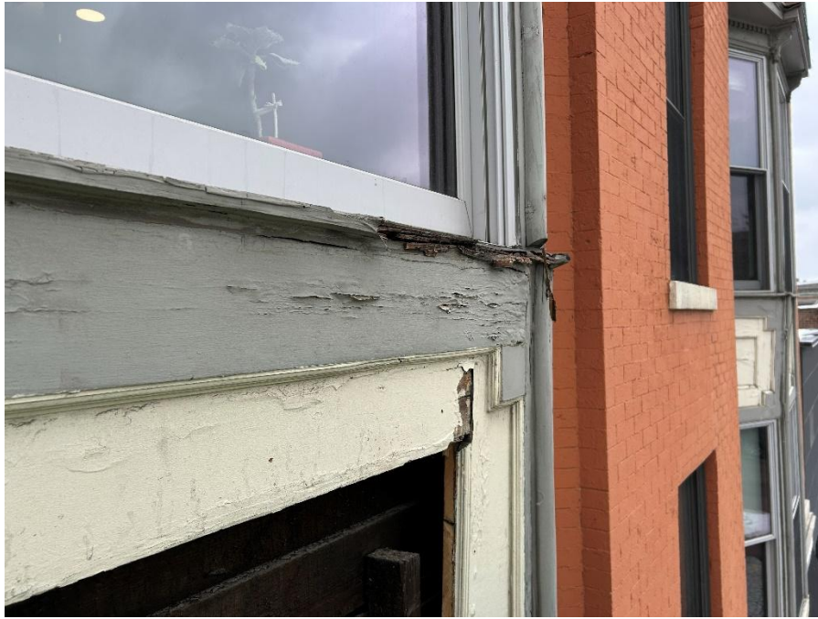
Photo 5: Typical wood paneling condition.
