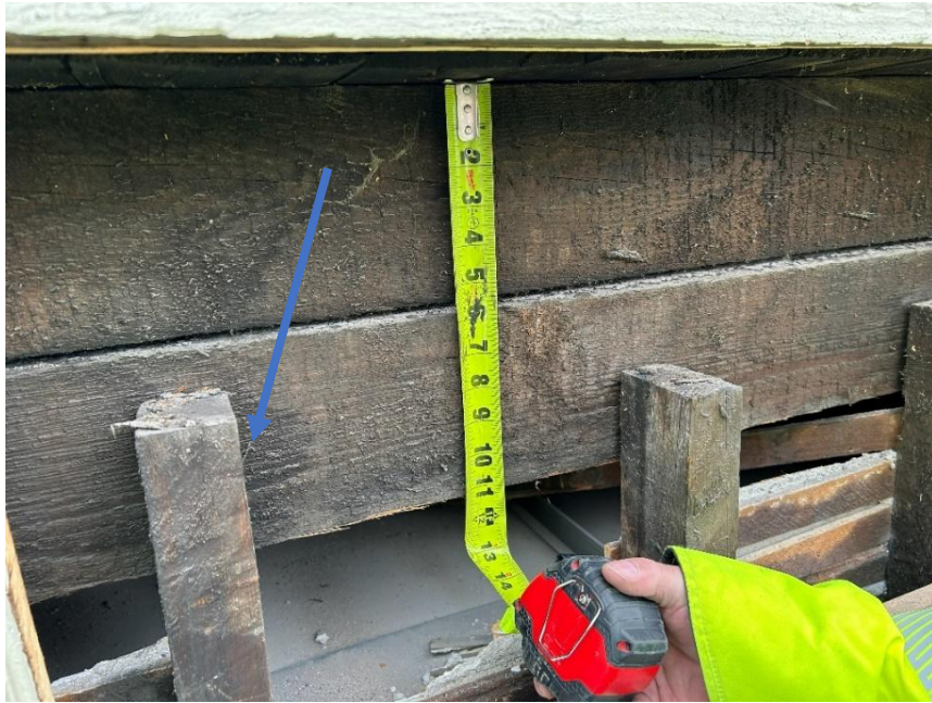
Photo 2: Support lumber members below third level bay window. Member indicated with a blue arrow matches member in Photo 4.
