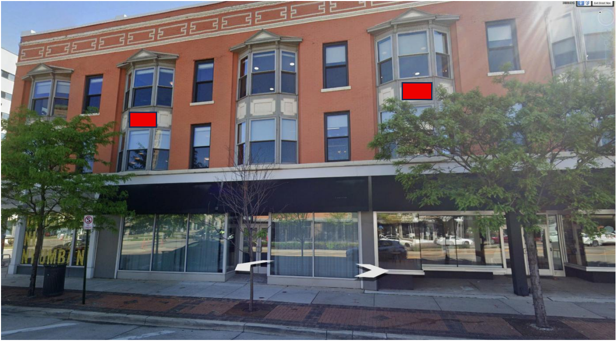
Photo 1: Observation opening locations (indicated with red boxes).
