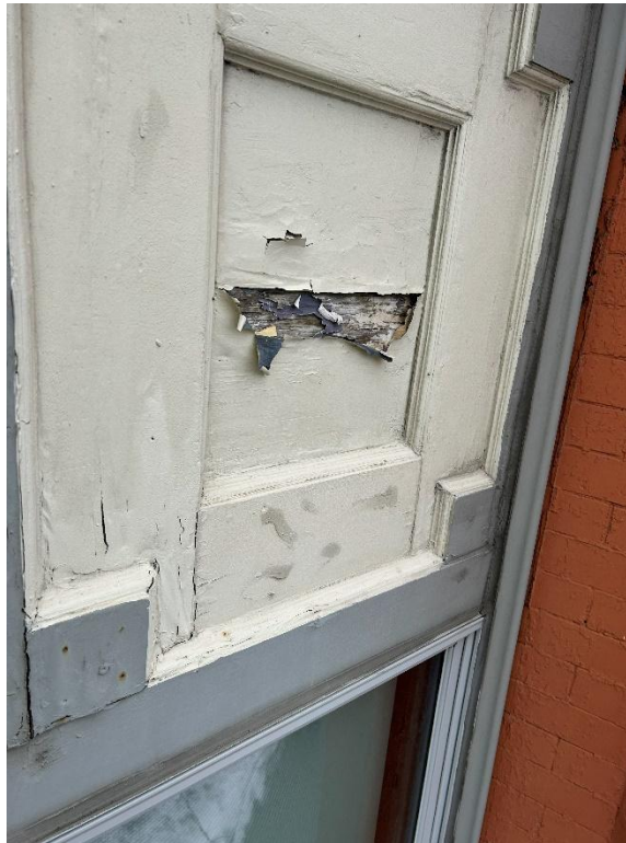
Photo 6: Typical wood paneling condition.
