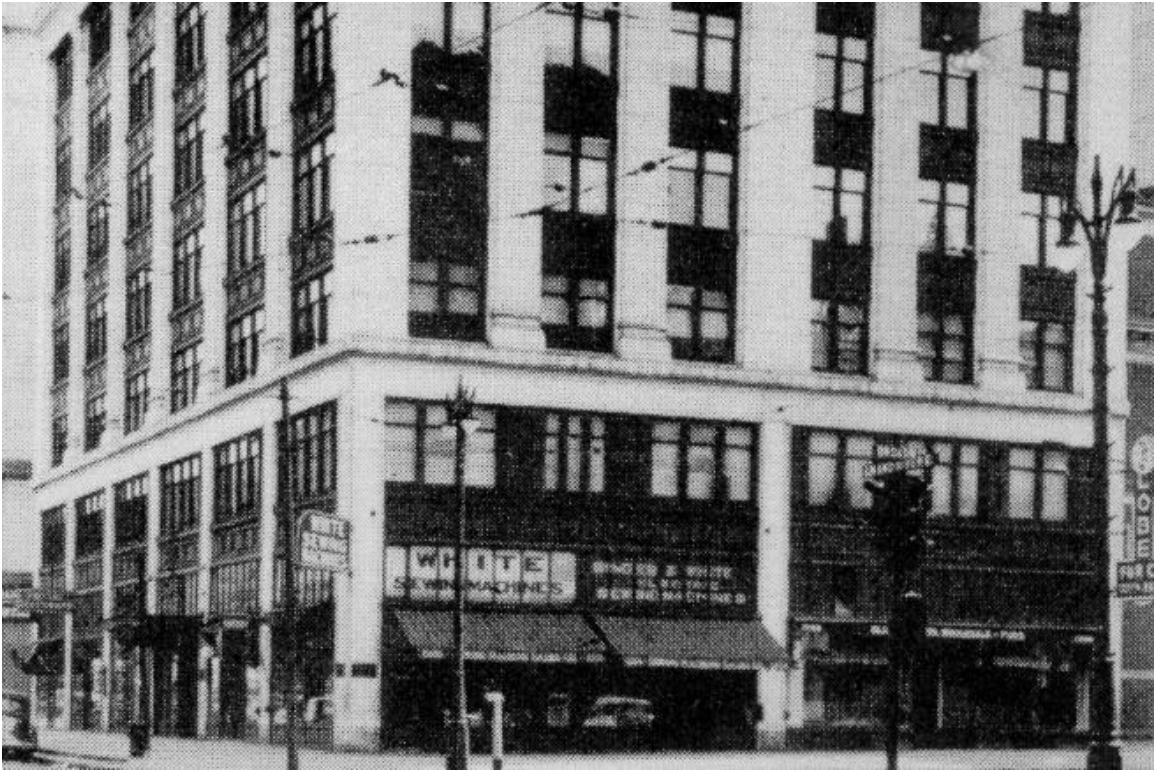
1. Historic Precedents of Grand River Canopy and Signage, Looking East. 1941.
