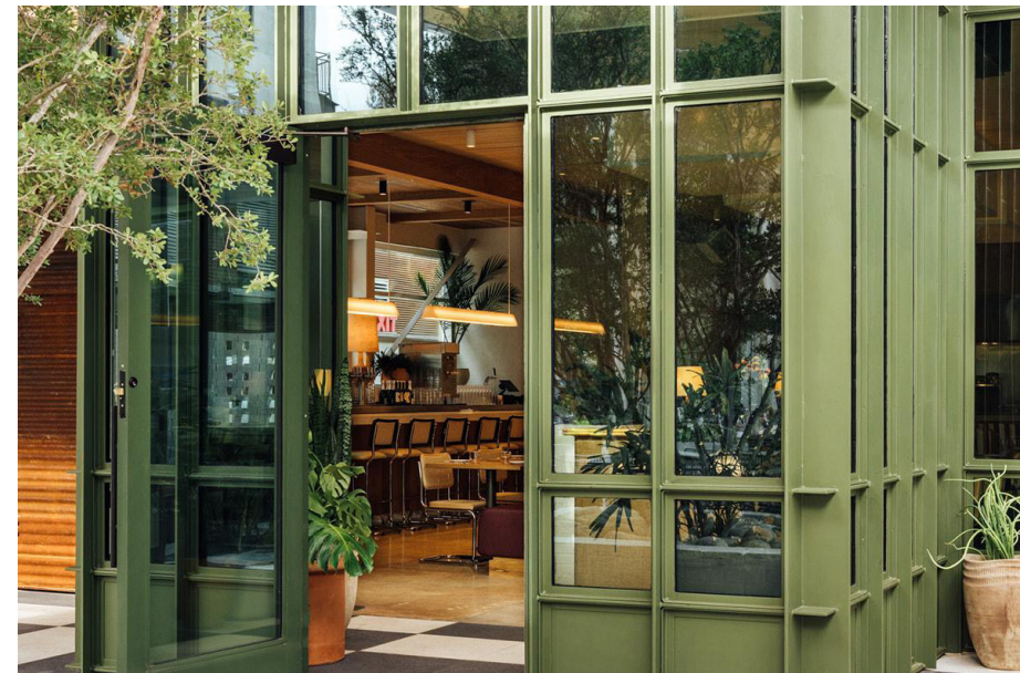
Glass Wall System and Muntins – ID Precedent (Rohe) Glass and Green Aluminum
