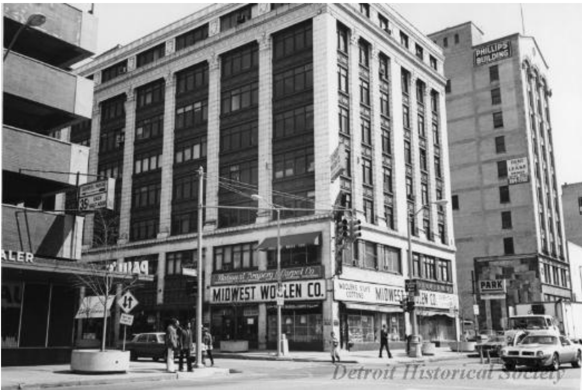
4. Historic Precedents of Corner Signage, Looking Southeast.
