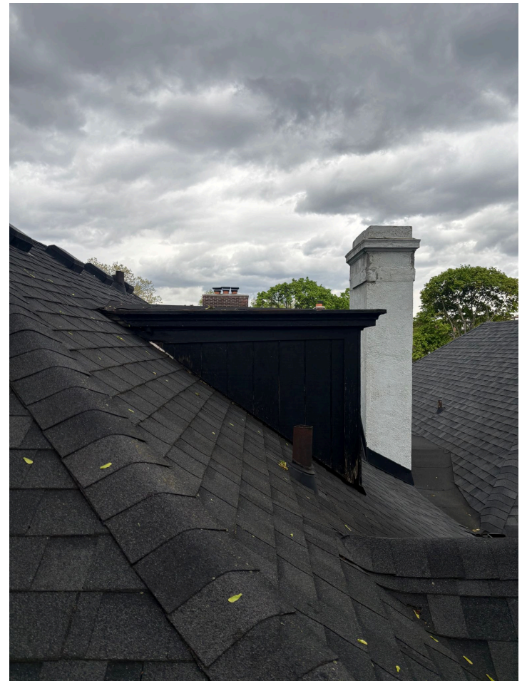
East Facing Dormer(side profile)
