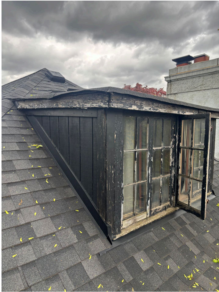
South Facing Dormer(sideyard)
