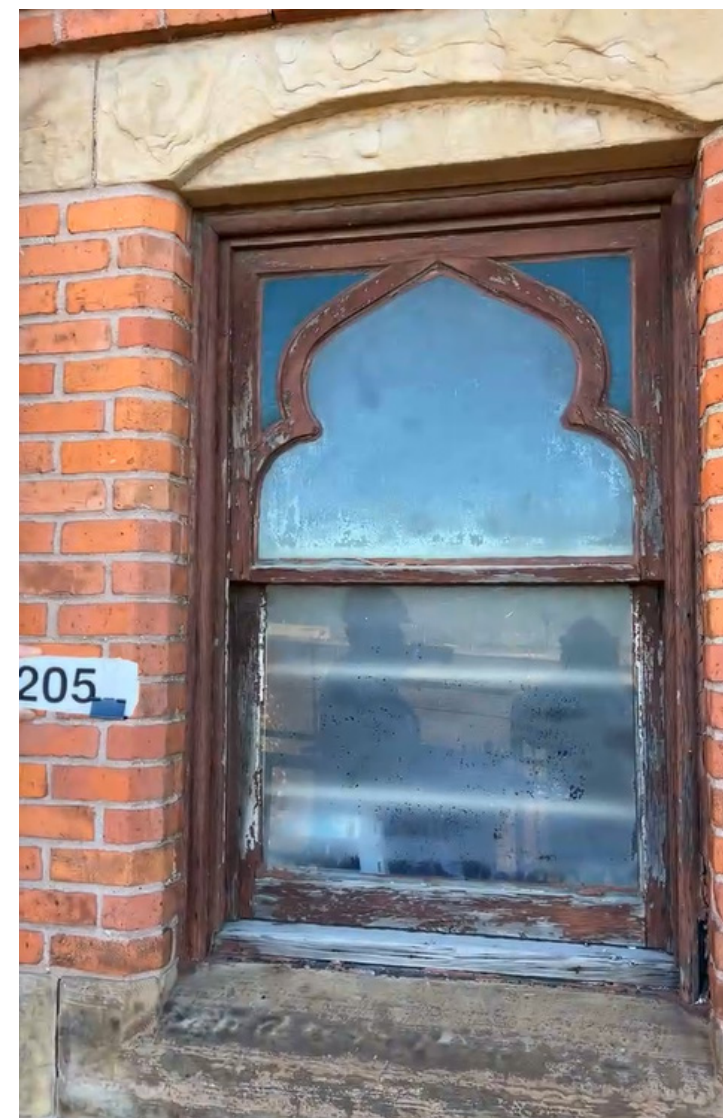
View of existing historic wood window #205 at Basilica (sacristy), 2nd floor, west elevation.
