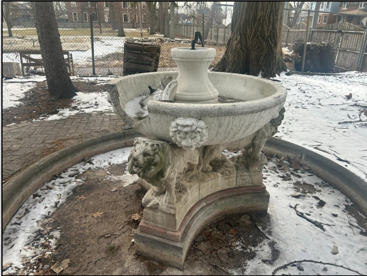
North Fountain base is historic. The bowl is not historic. The basin is in disrepair.
