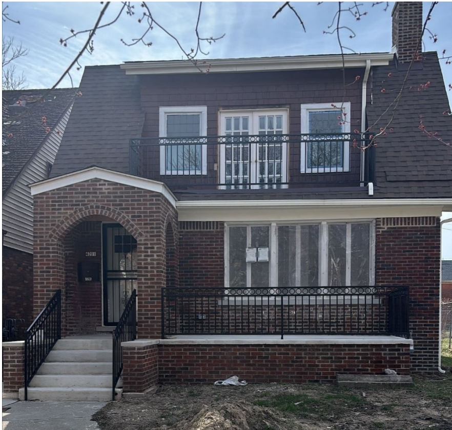
2026 – Window and Door restoration complete on front facade
