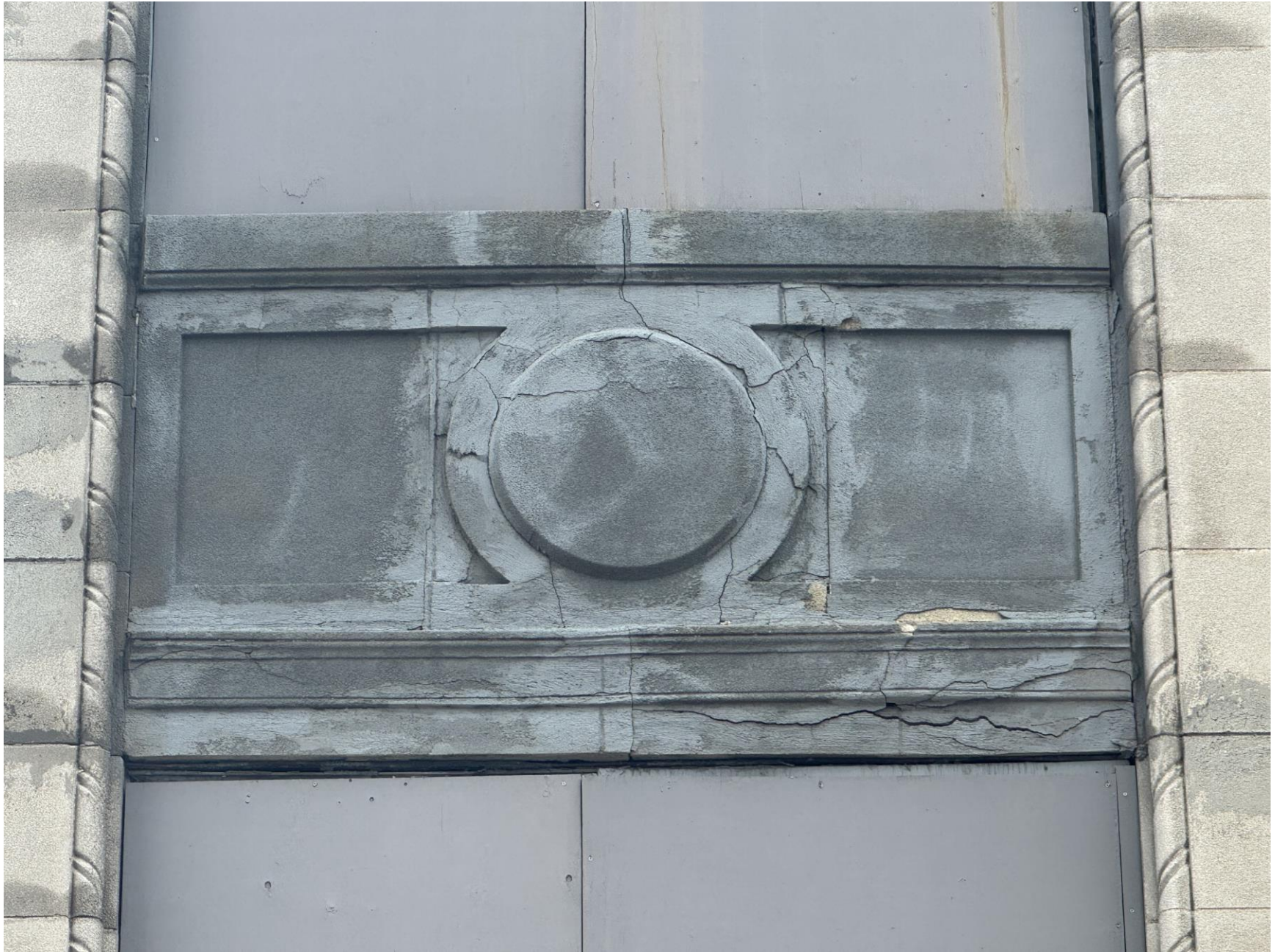
Photo S1 (West Elevation – Between Column Lines A & B)
