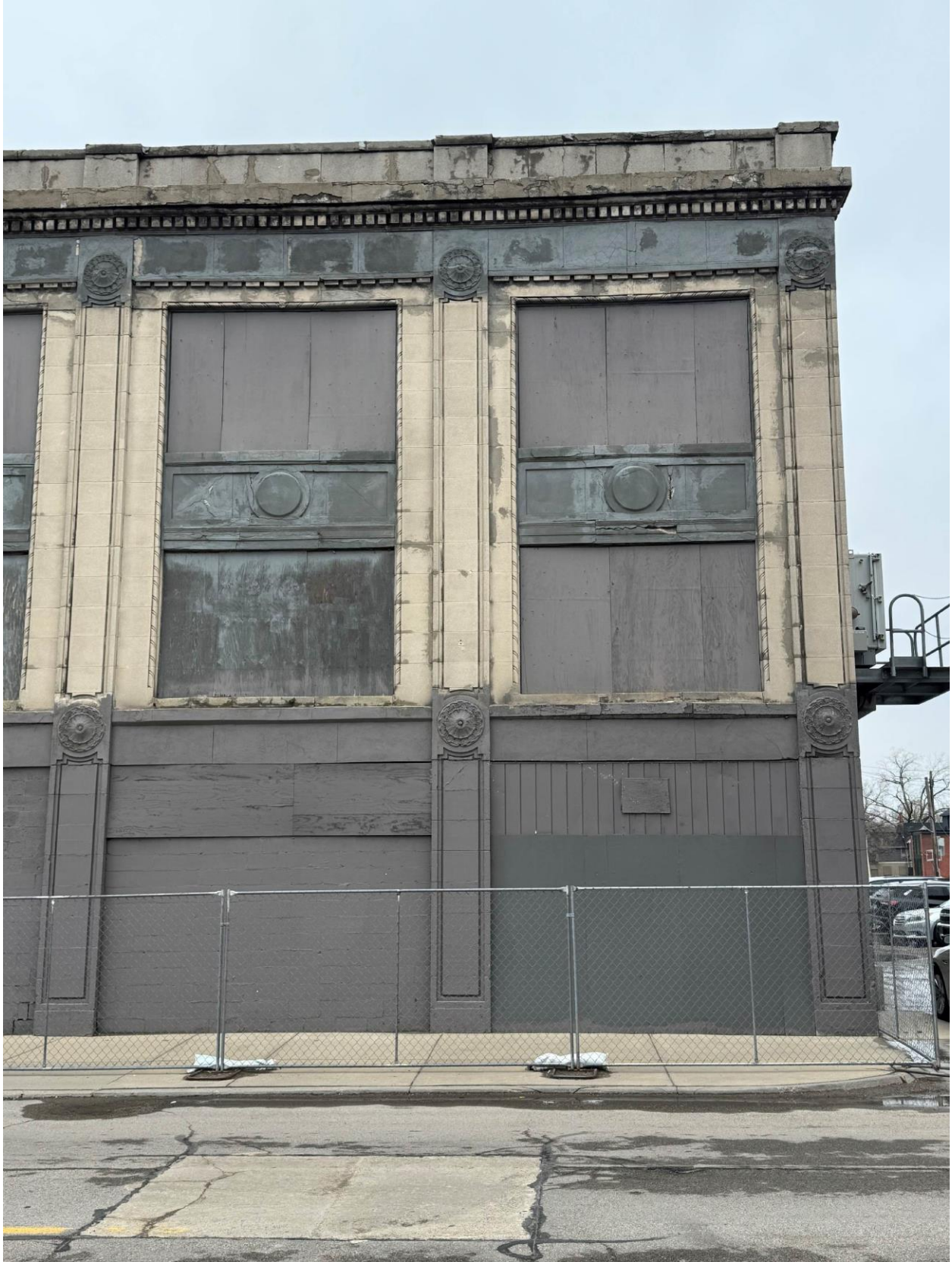
Photo F5 (Partial South Elevation – Column Lines 6, 7 & 8)
