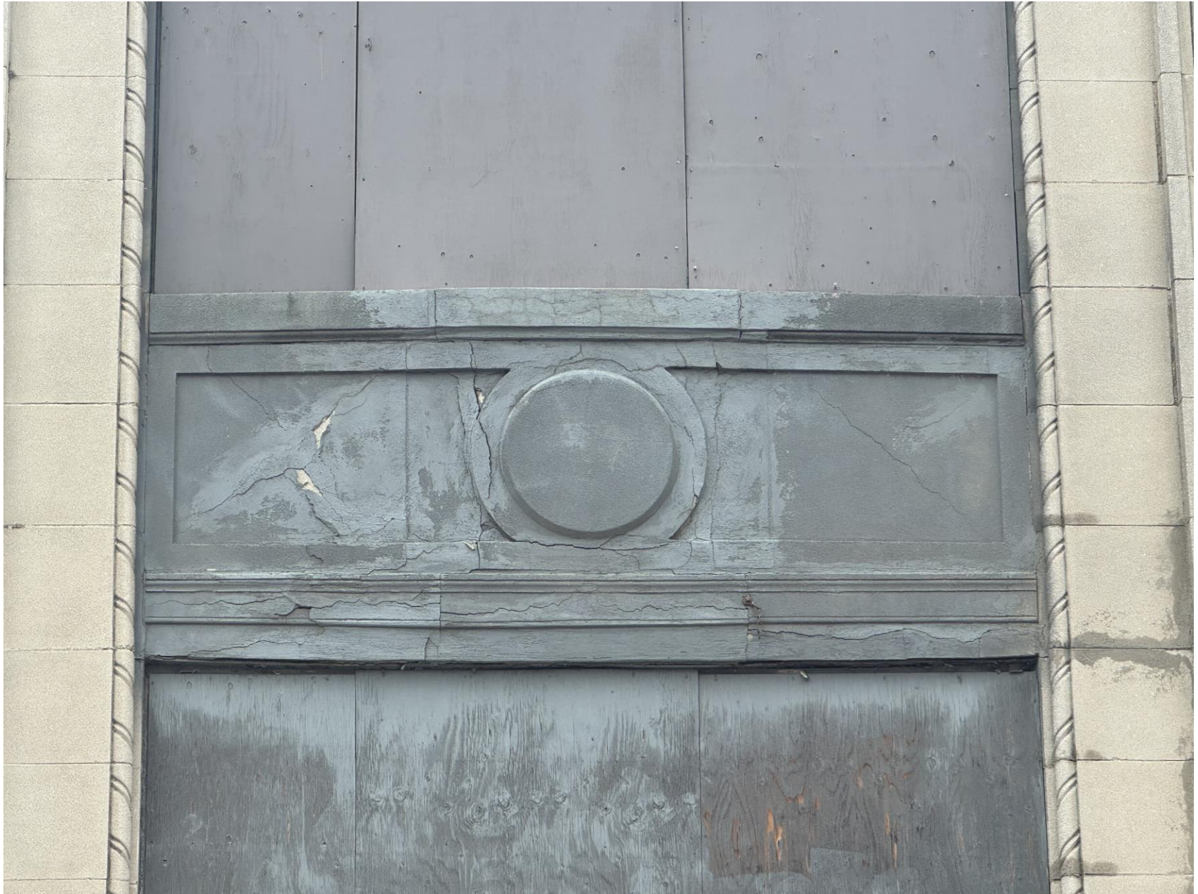
Photo S8 (South Elevation – Between Column Lines 6 & 7)
