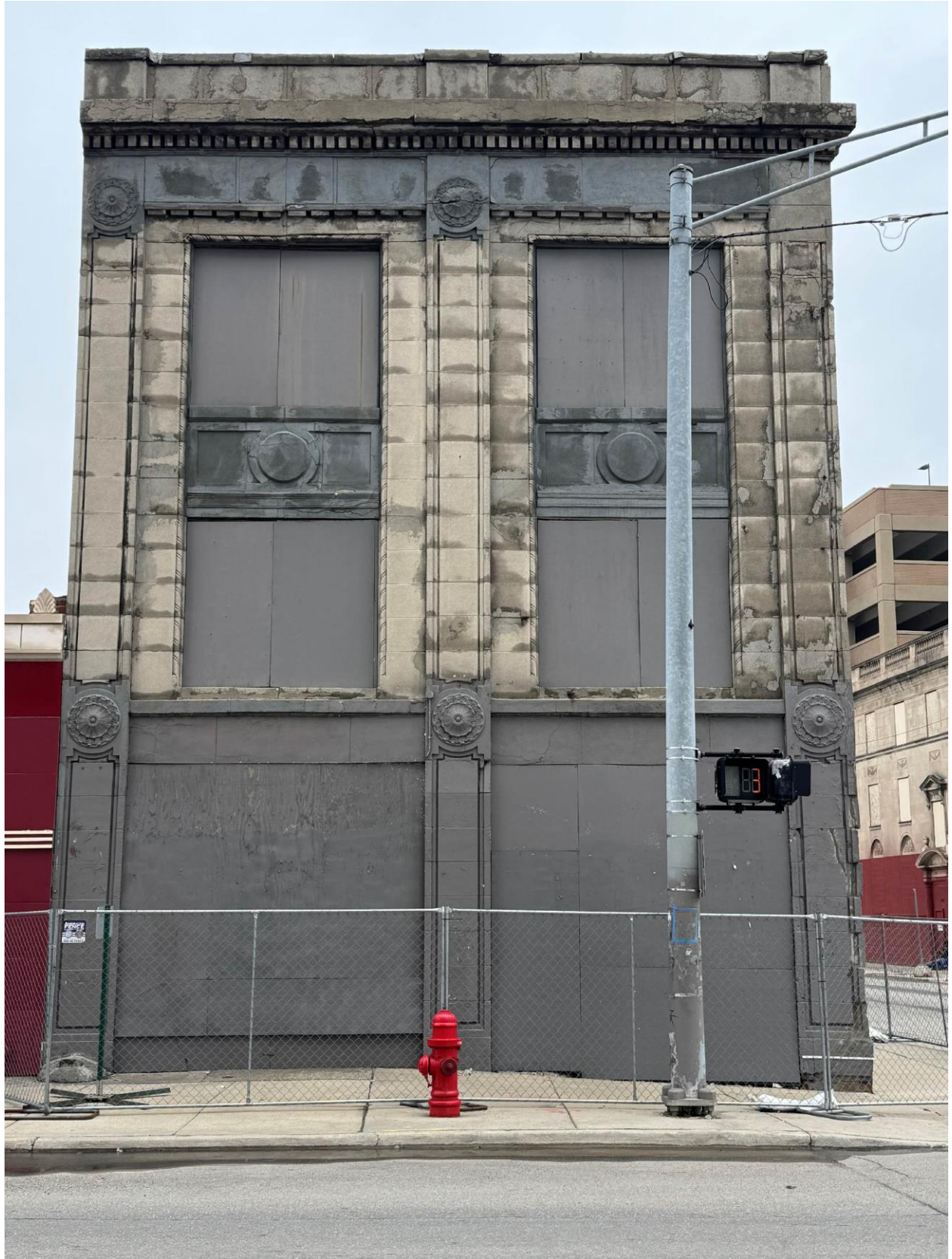
Photo F1 (West Elevation – Column Lines A, B & C)
