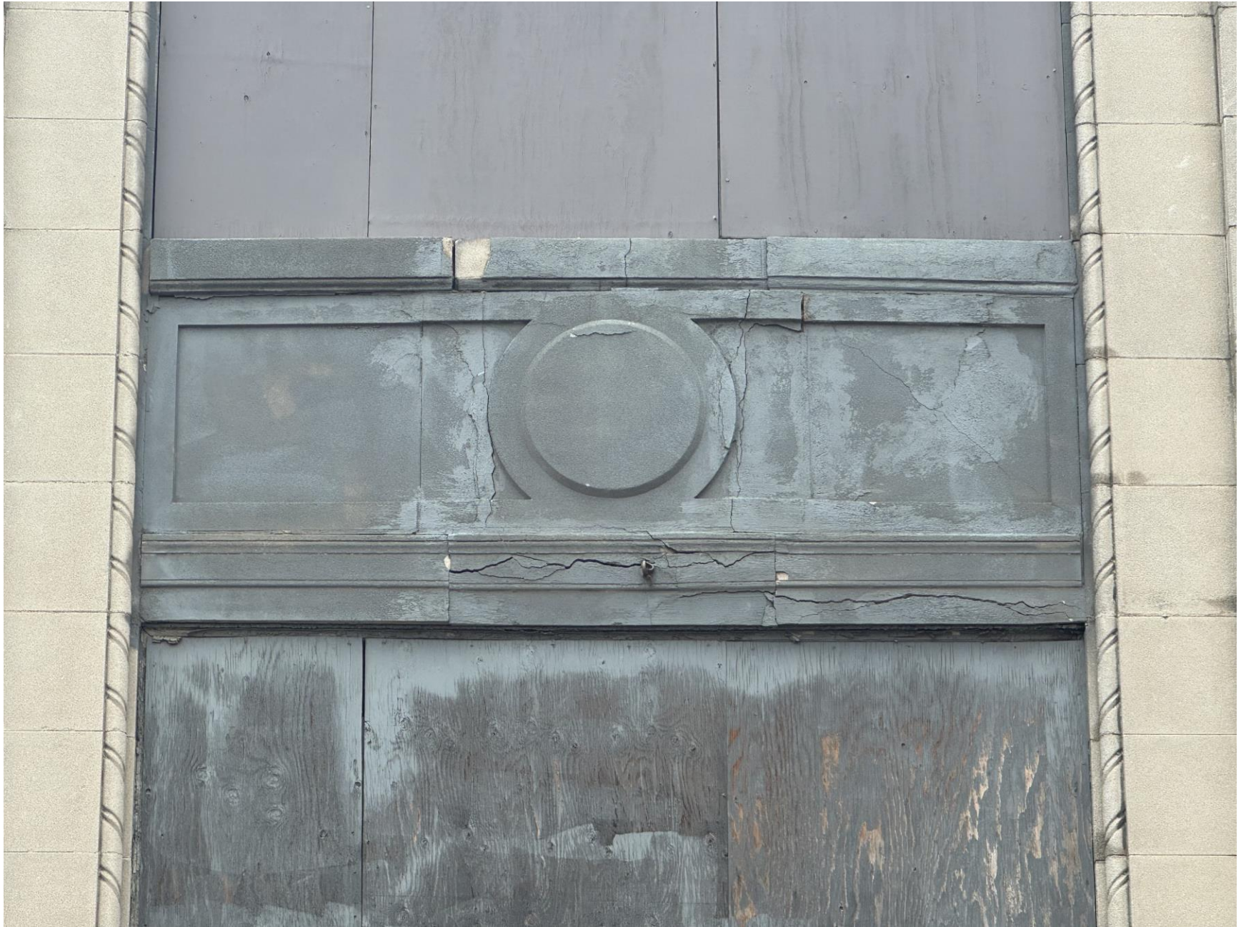
Photo S7 (South Elevation – Between Column Lines 5 & 6)
