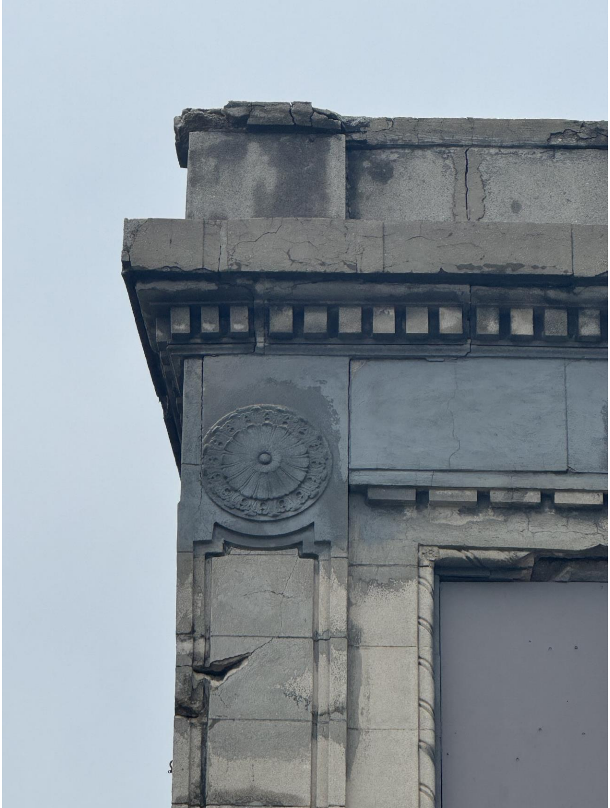
Photo M3 (South Elevation – Column Line 1)
