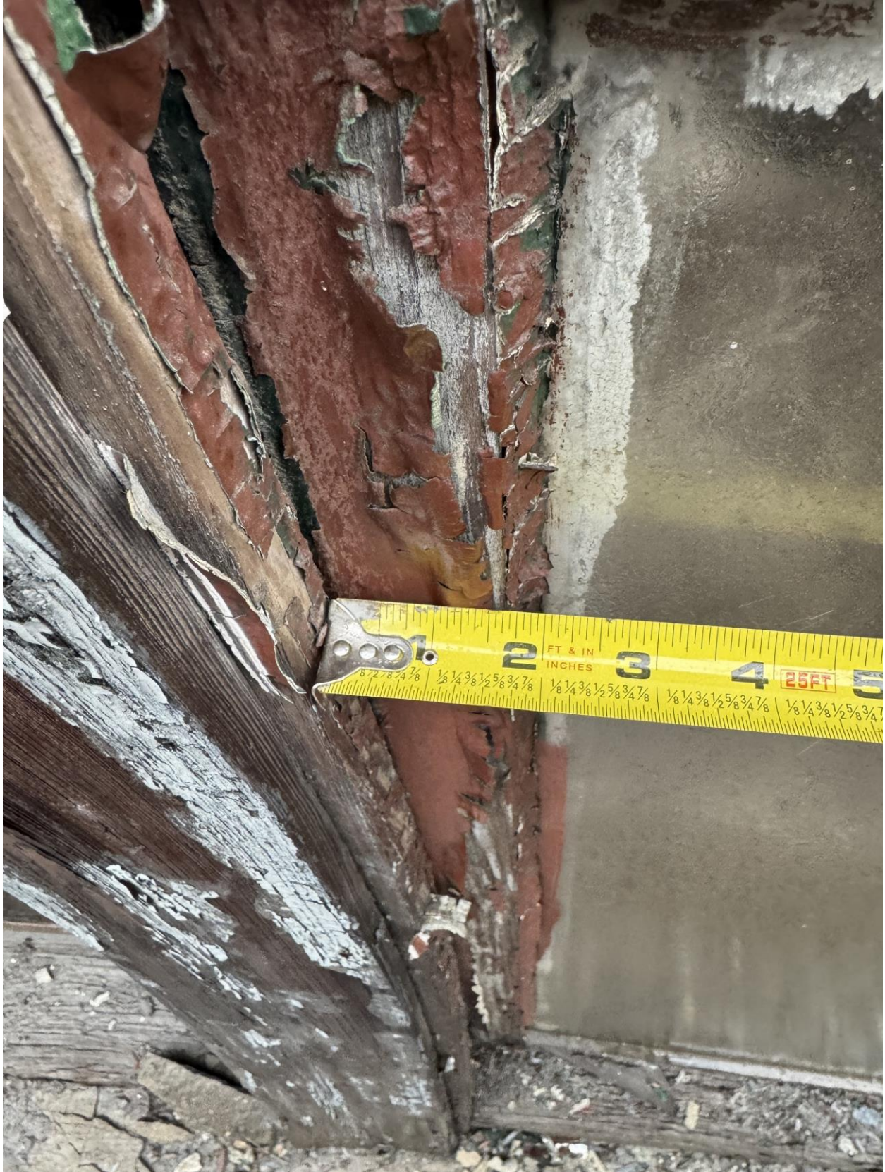
Photo W12 (Mull & Sash Stile)
