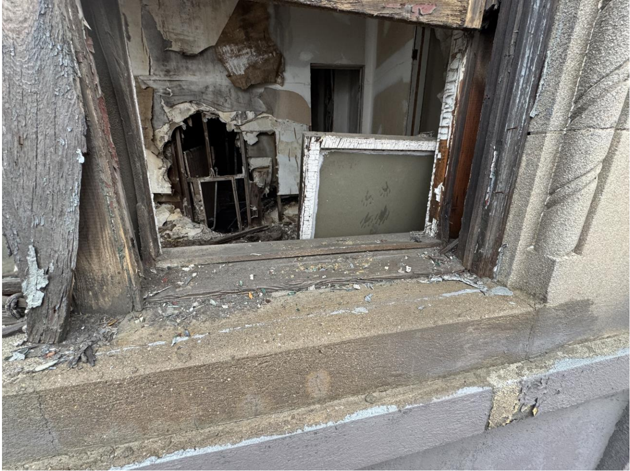
Photo W3 (Right Window – Sill & Lower Sash Opening)
