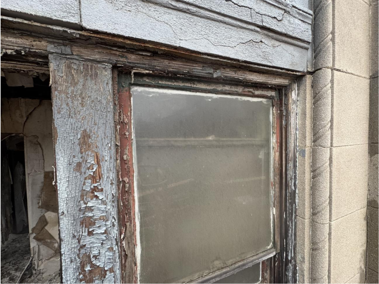
Photo W6 (Right Window – Upper Sash, Mull, & Head)
