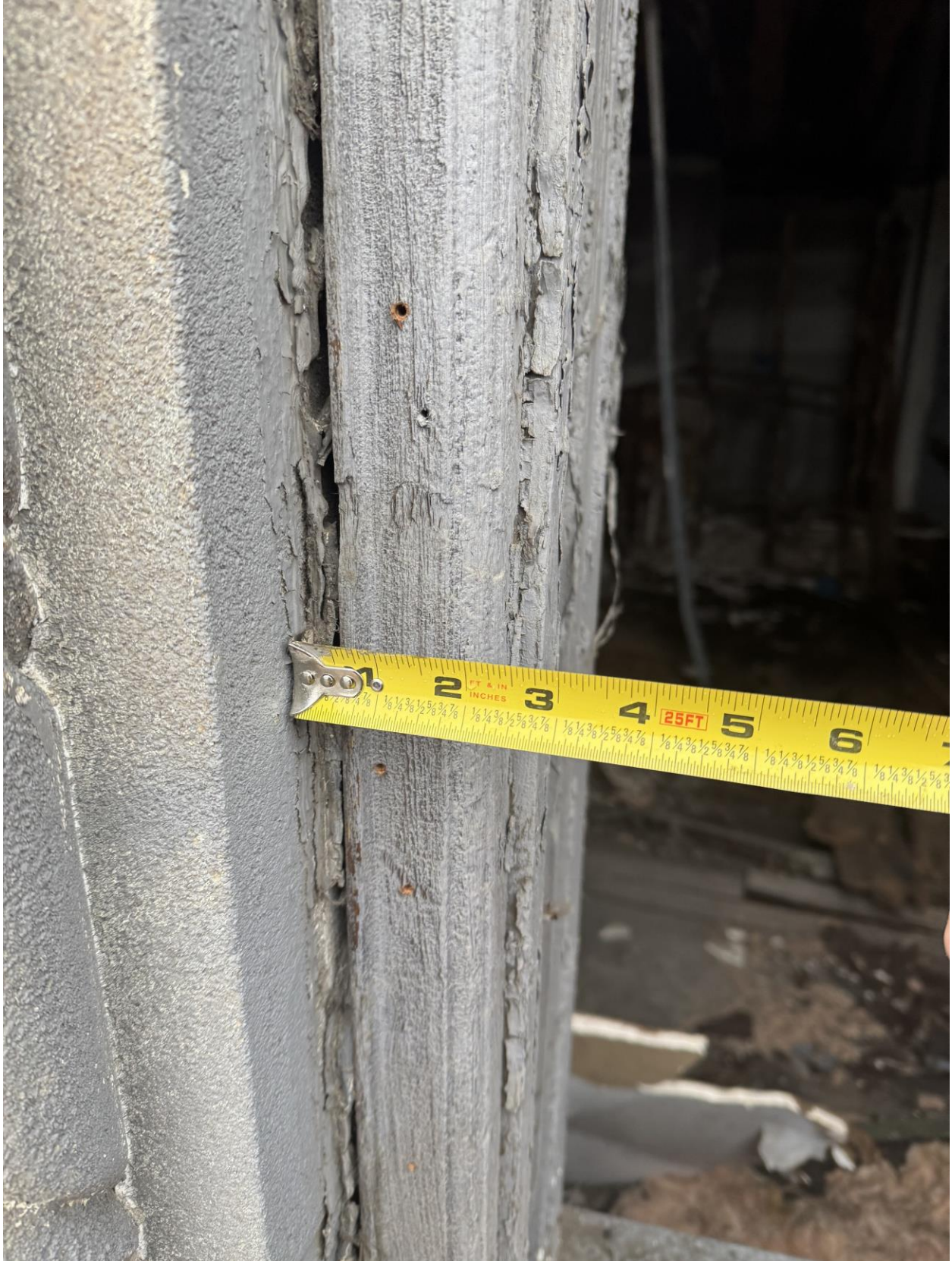
Photo W8 (Brick Molding)
