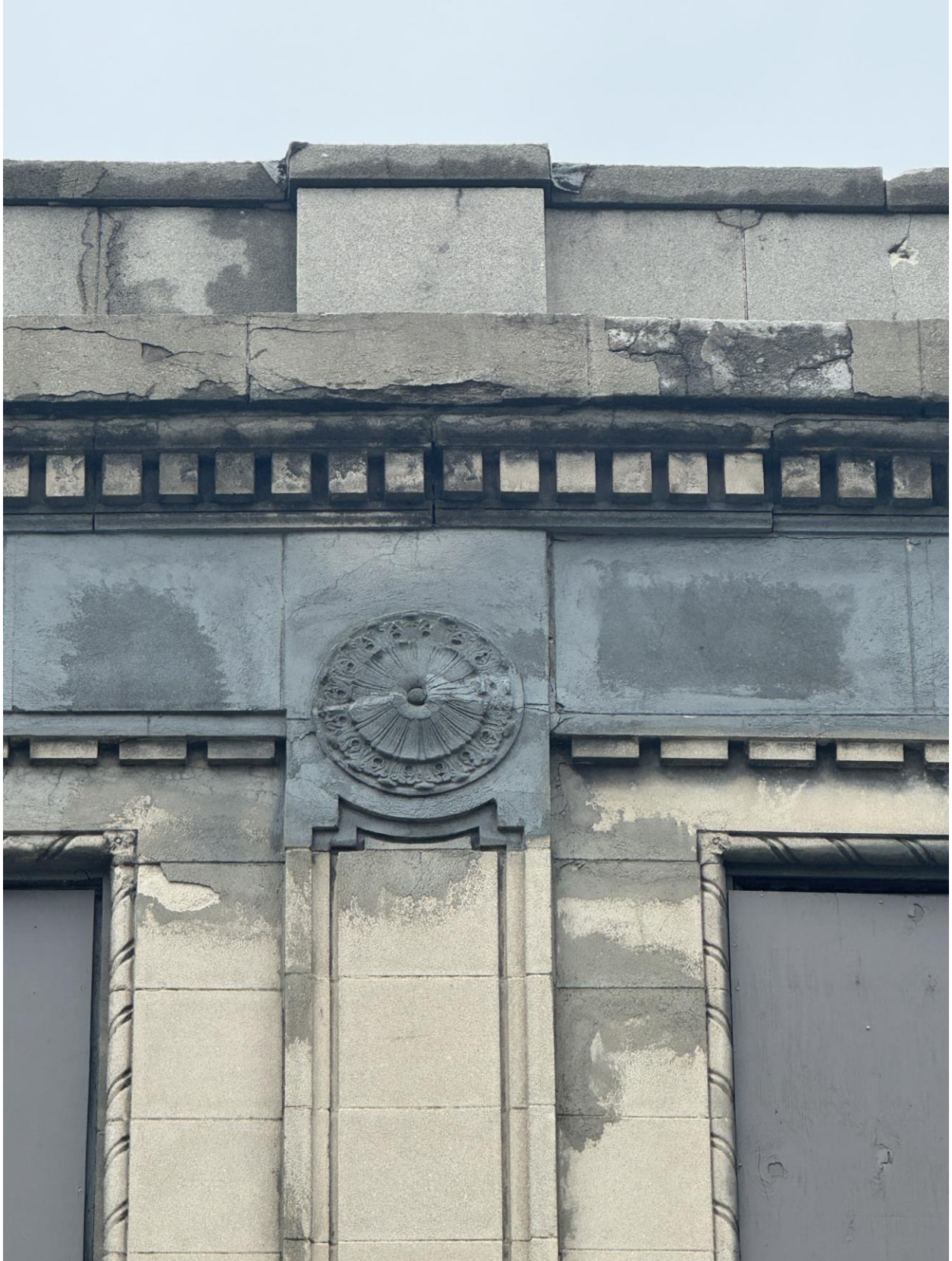
Photo M5 (South Elevation – Column Line 3)
