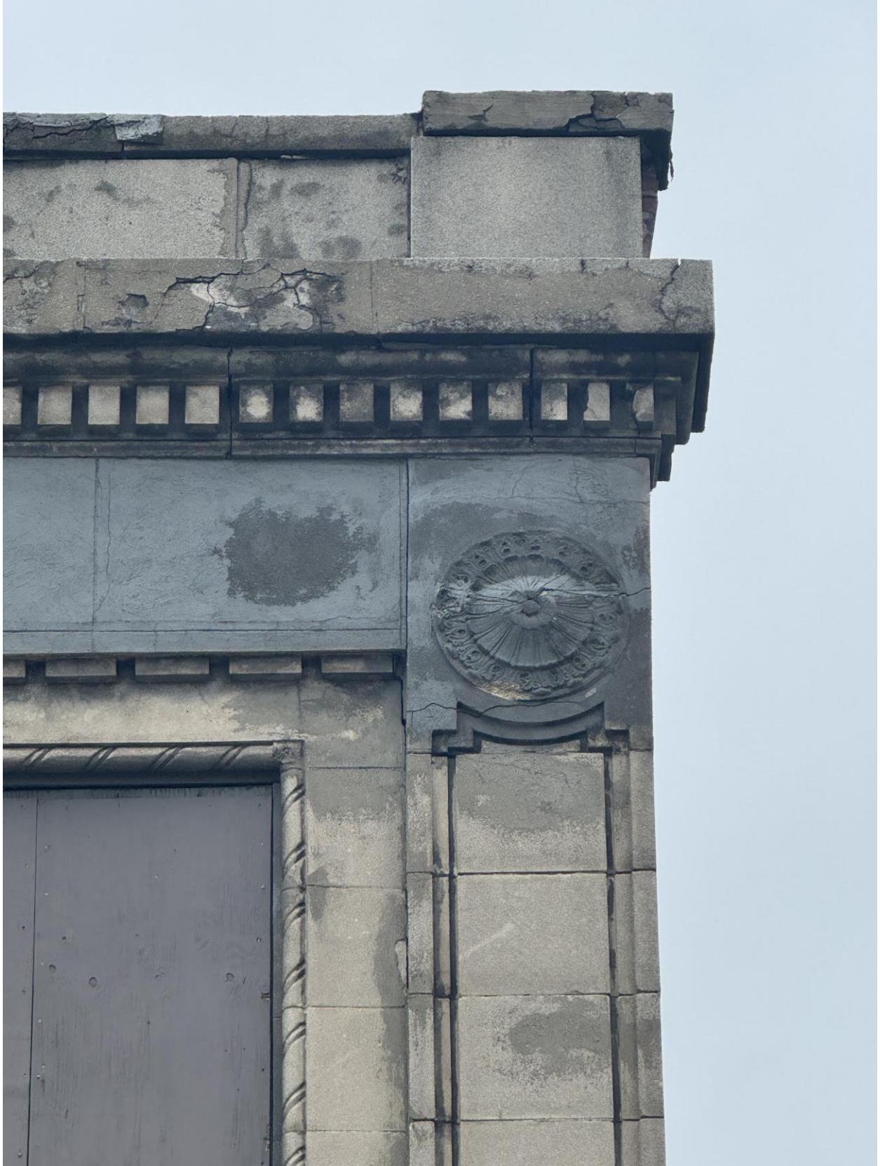
Photo M10 (South Elevation – Column Line 8)
