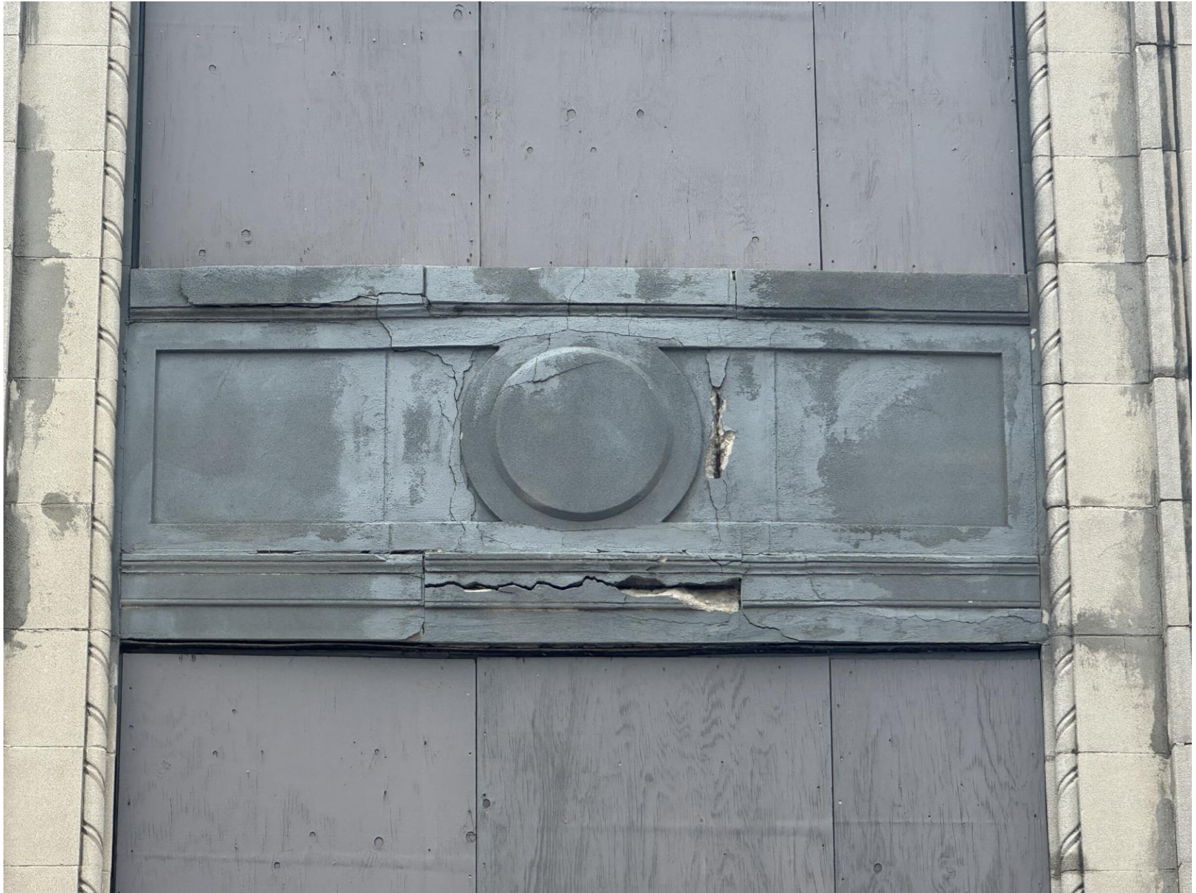
Photo S9 (South Elevation – Between Column Lines 7 & 8)
