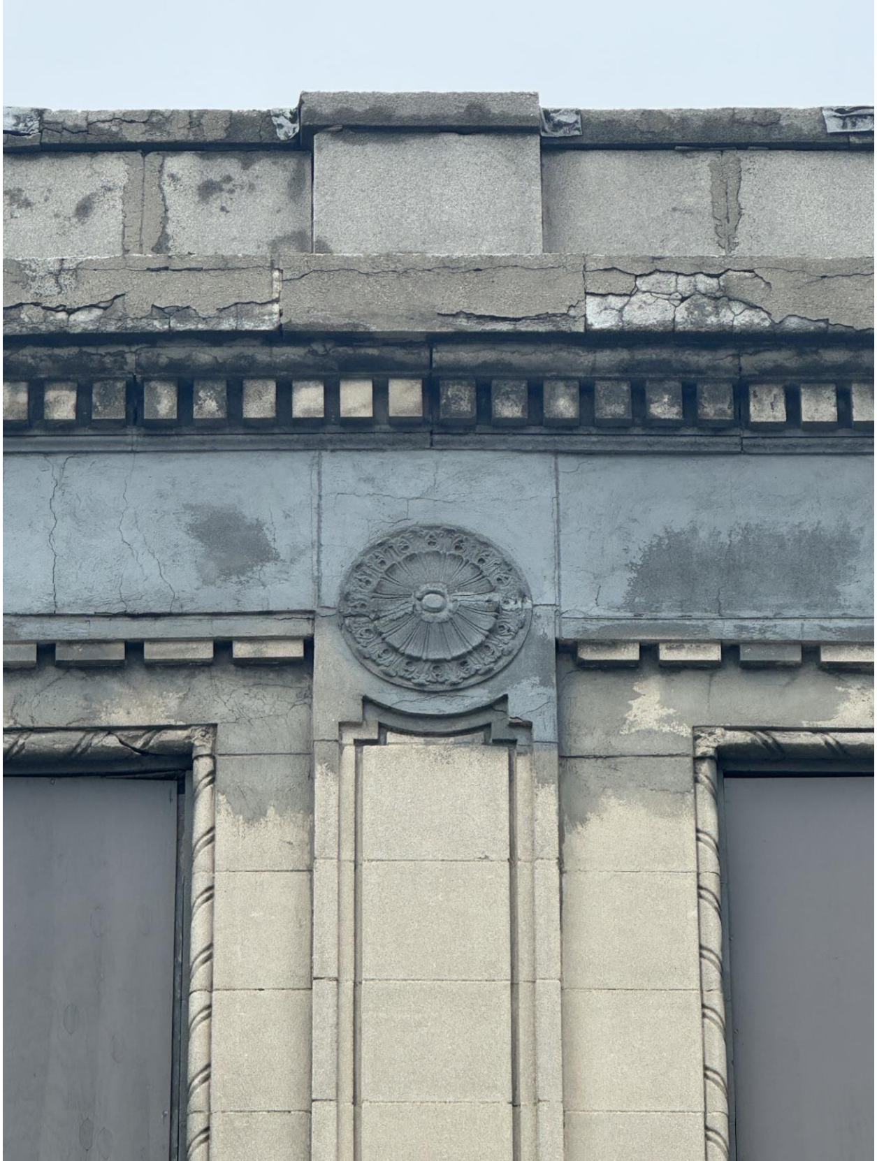
Photo M4 (South Elevation – Column Line 2)
