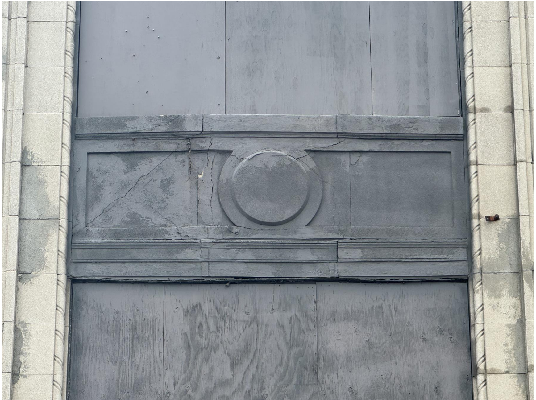
Photo S3 (South Elevation – Between Column Lines 1 & 2)
