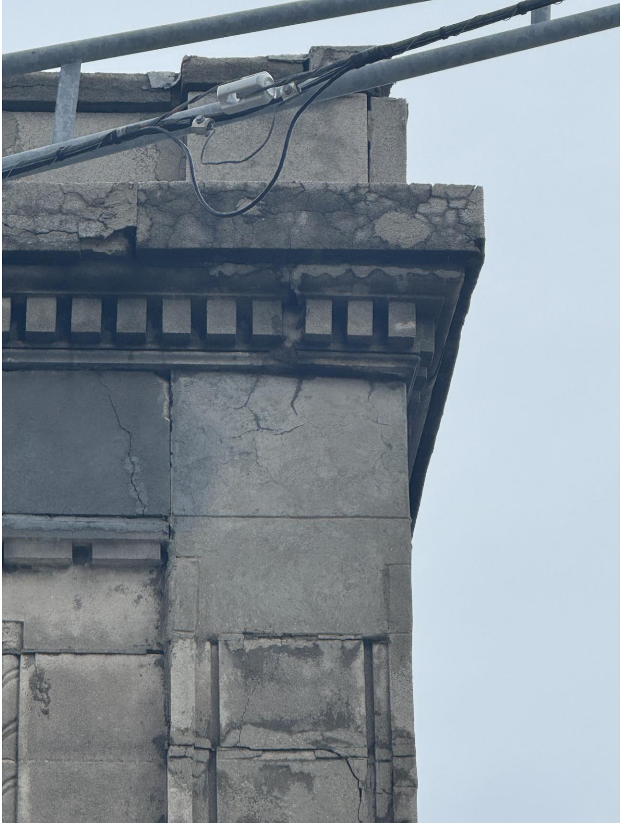
Photo M2 (West Elevation – Column Line C)
