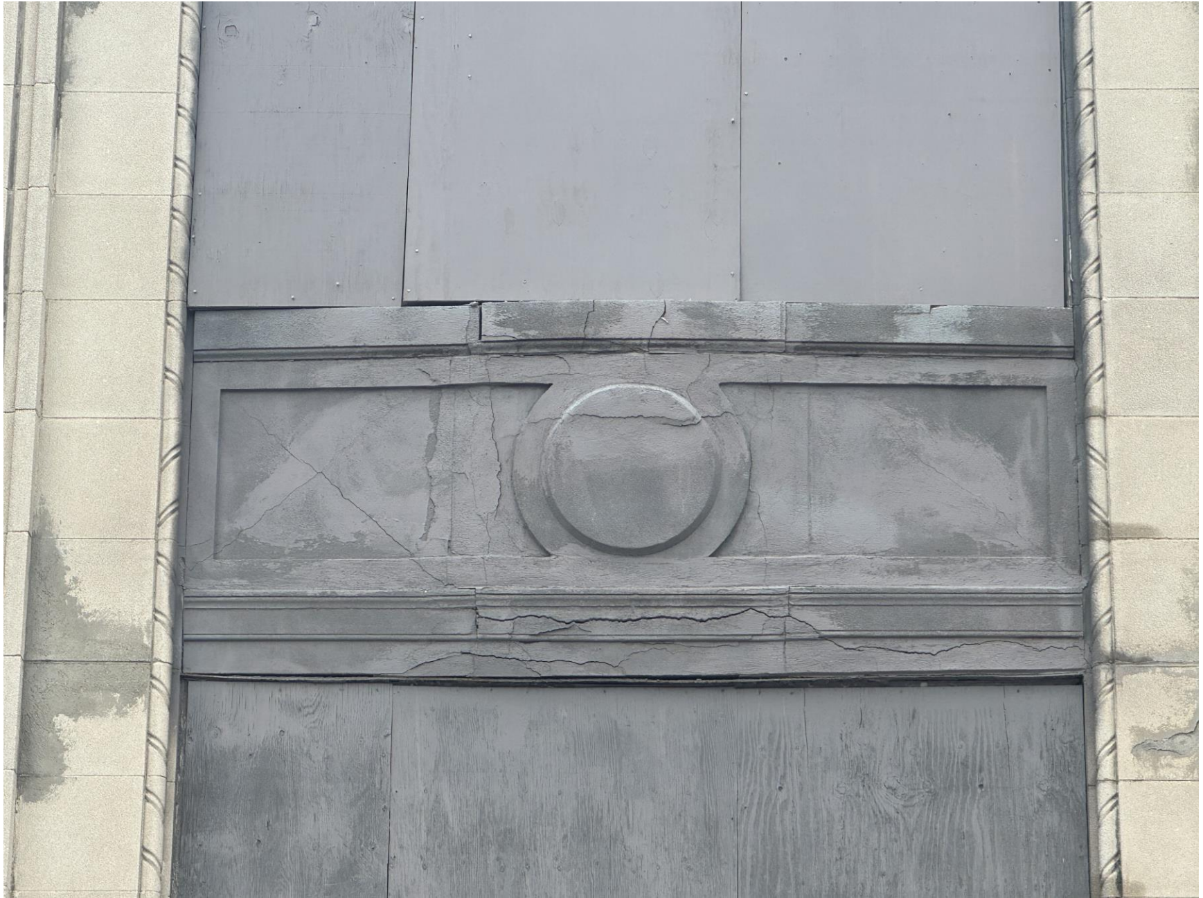
Photo S5 (South Elevation – Between Column Lines 3 & 4)
