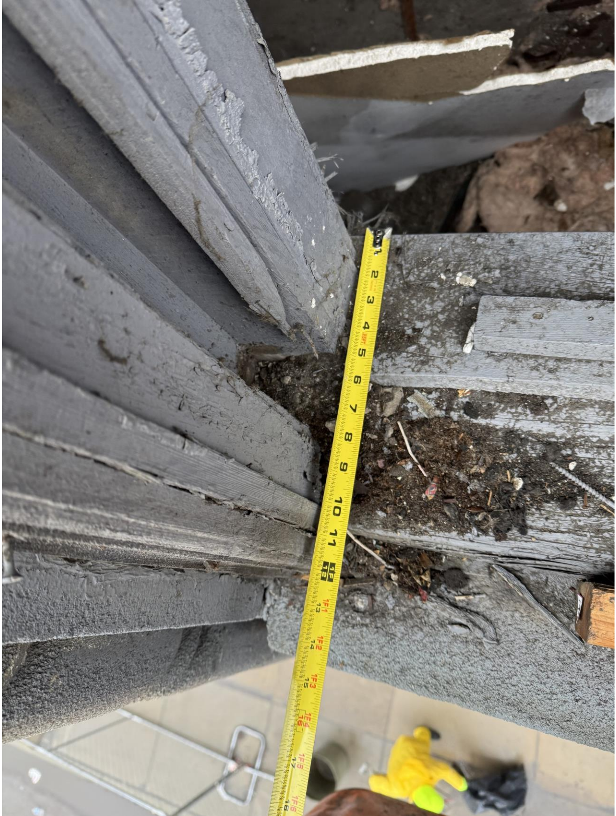
Photo W10 (Sill @ Spandrel)
