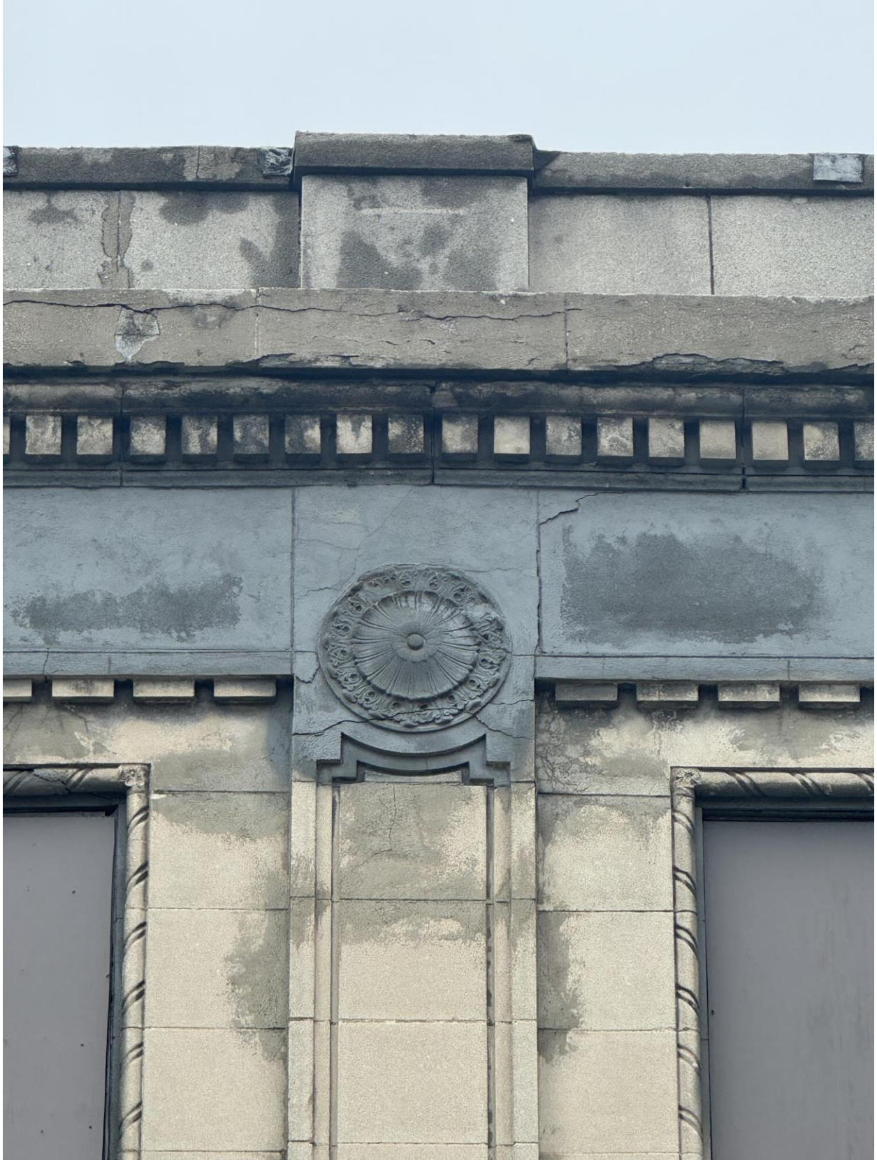
Photo M6 (South Elevation – Column Line 4)
