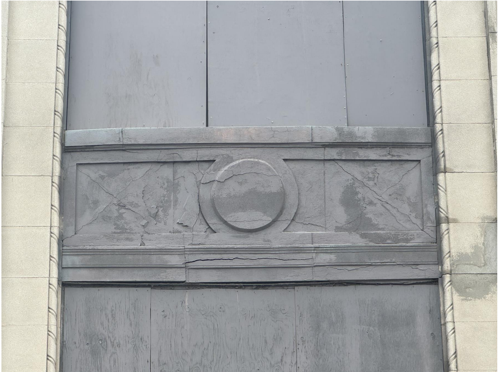
Photo S4 (South Elevation – Between Column Lines 2 & 3)
