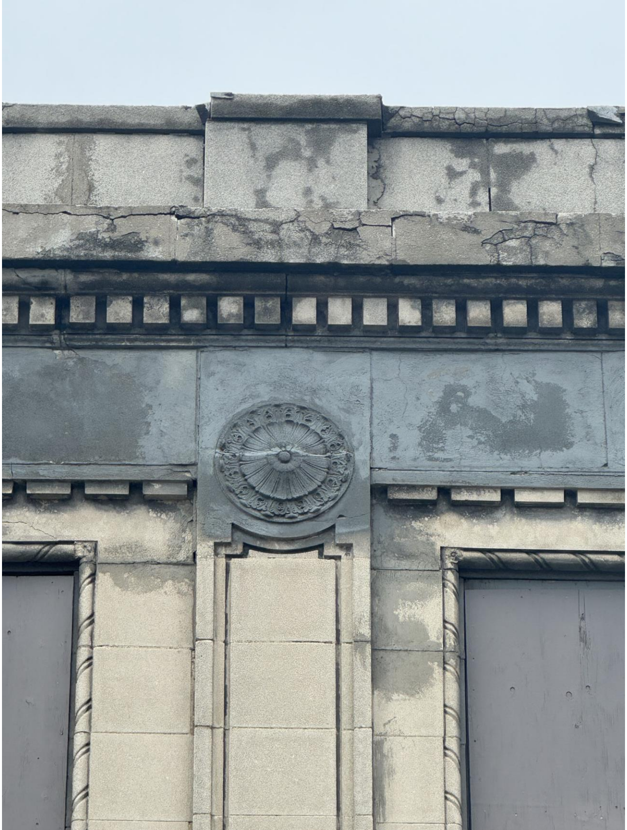
Photo M9 (South Elevation – Column Line 7)
