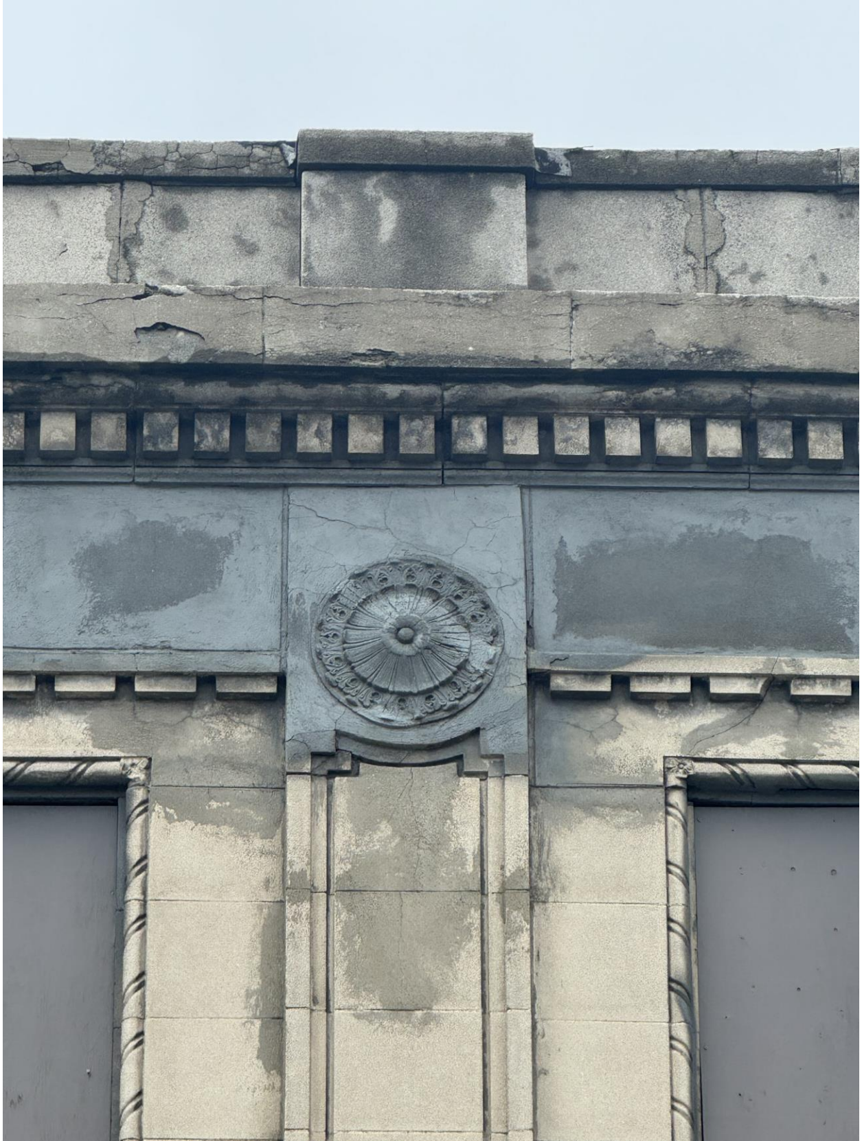
Photo M7 (South Elevation – Column Line 5)
