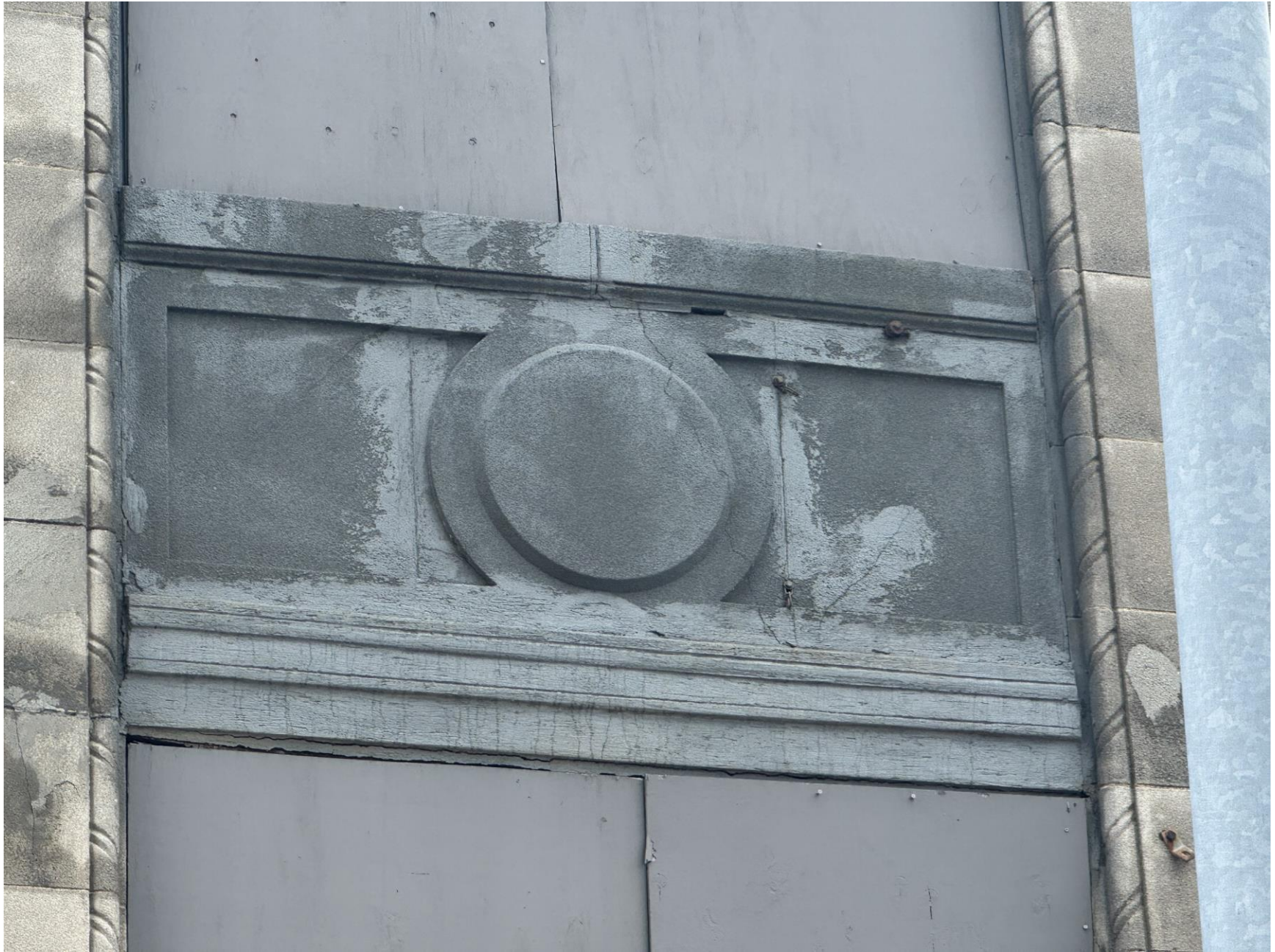
Photo S2 (West Elevation – Between Column Lines B & C)
