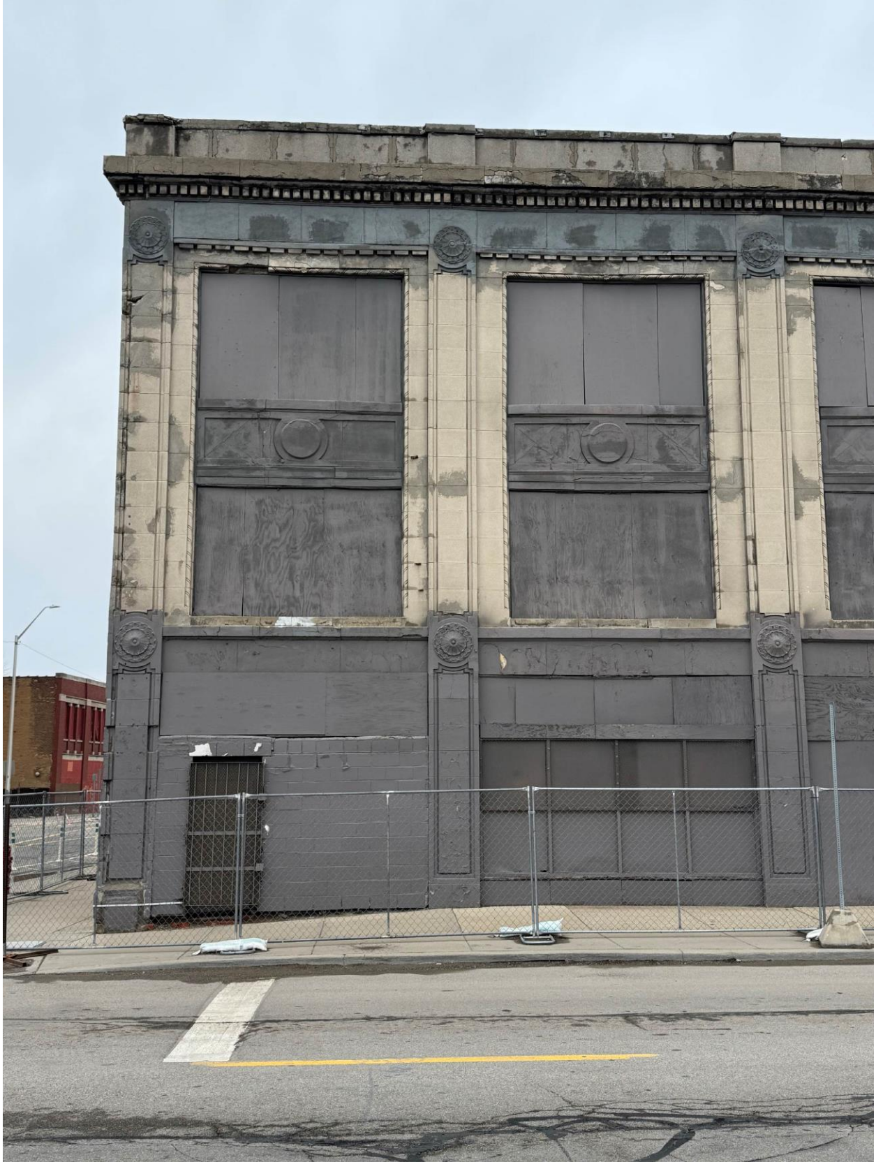
Photo F2 (Partial South Elevation – Column Lines 1, 2 & 3)
