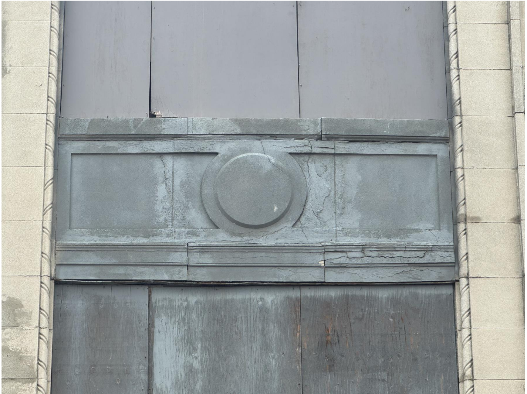
Photo S6 (South Elevation – Between Column Lines 4 & 5)
