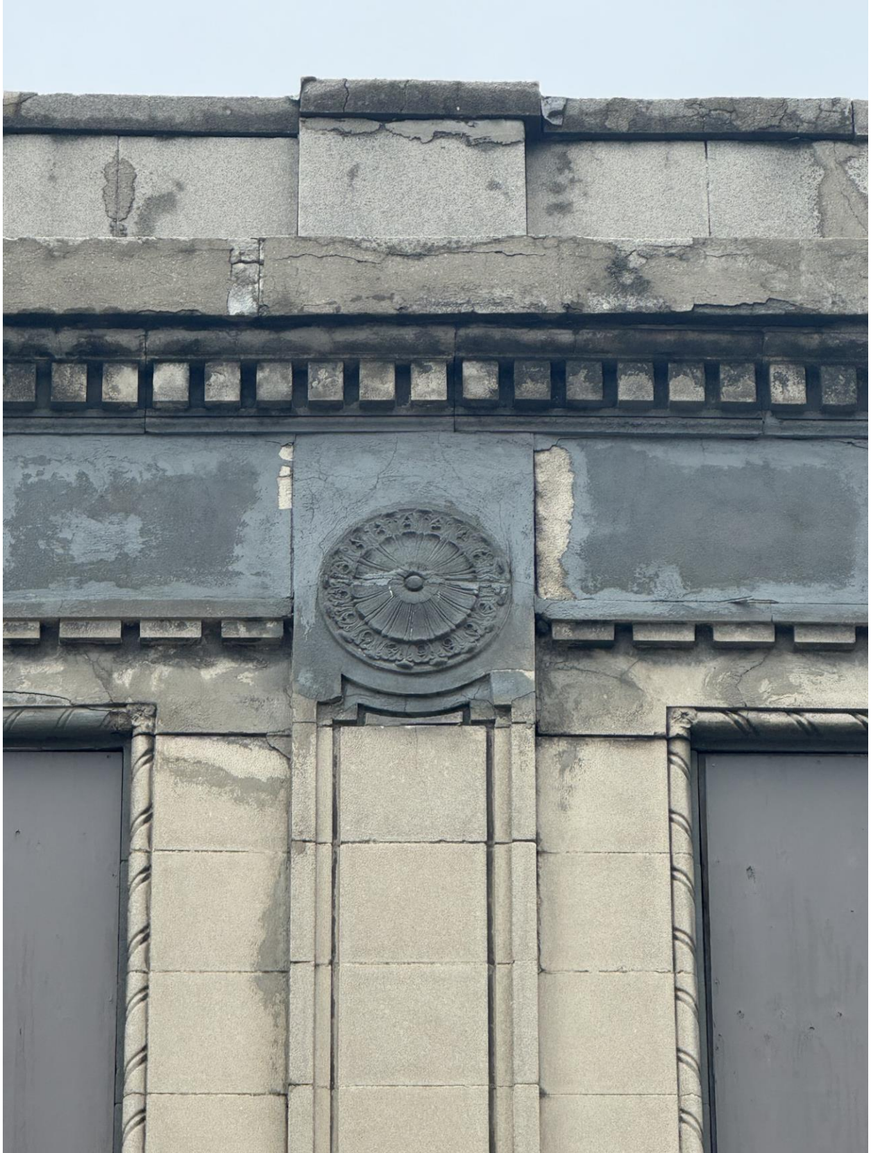
Photo M8 (South Elevation – Column Line 6)
