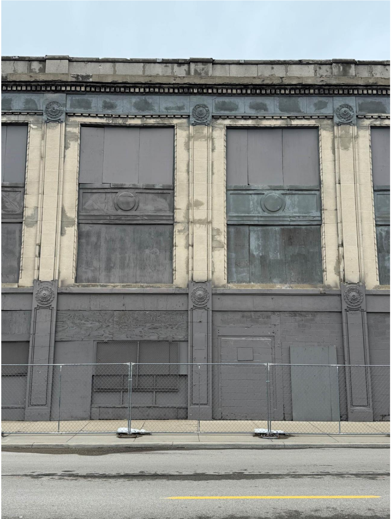
Photo F3 (Partial South Elevation Column Lines 3, 4 & 5)
