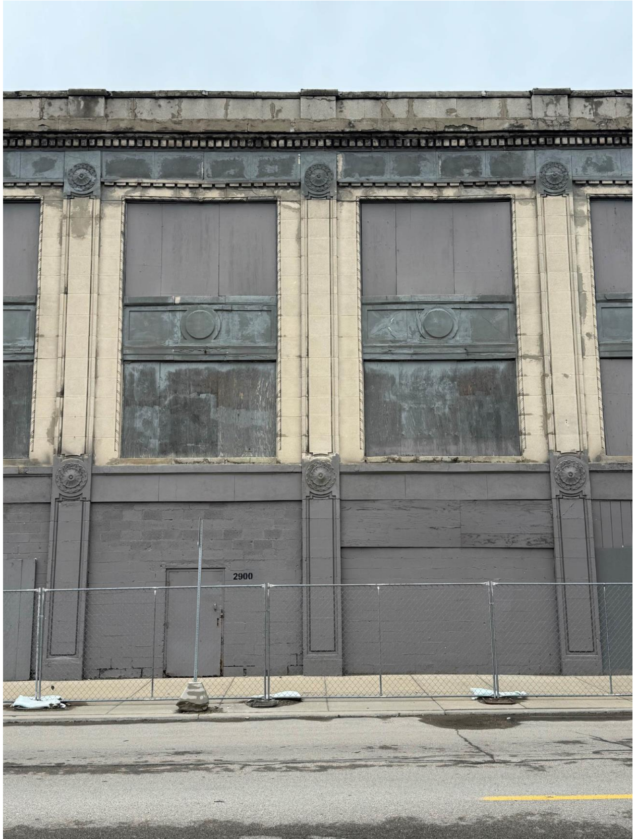
Photo F4 (Partial South Elevation – Column Lines 5, 6 & 7)
