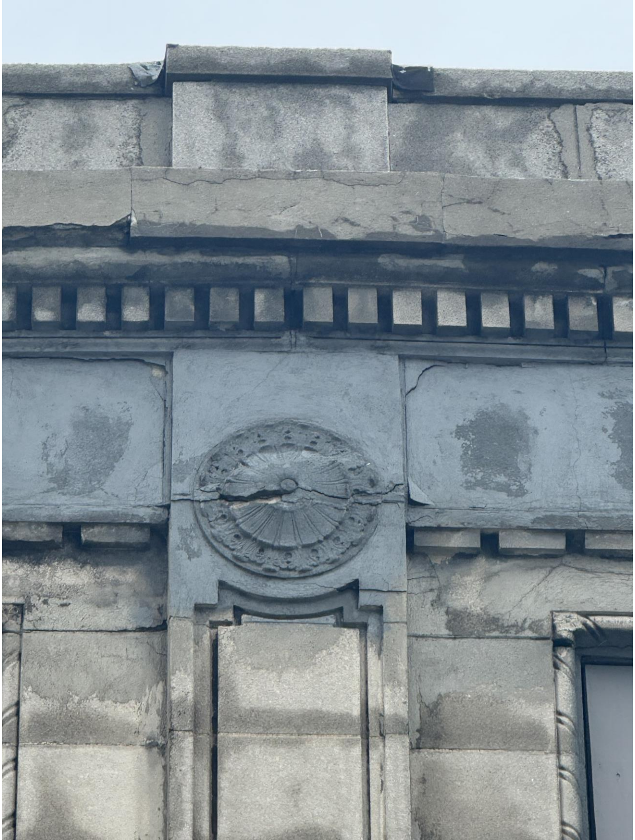
Photo M1 (West Elevation – Column Line B)
