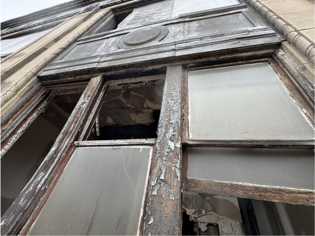
Photo W5 (Upper Sash & Spandrel)
