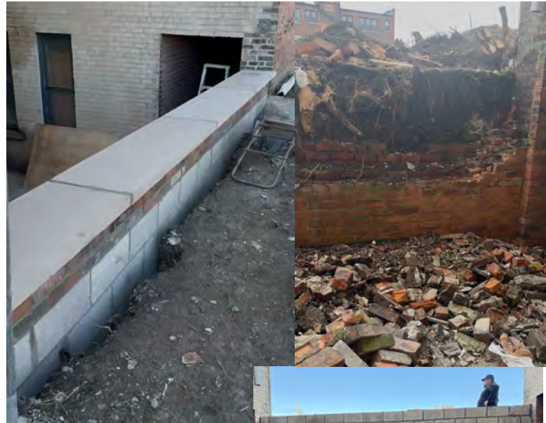
3 images below showing repaired wall and New limestone cap
