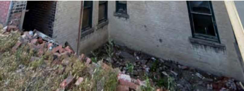
2 images below Showing original retaining wall
