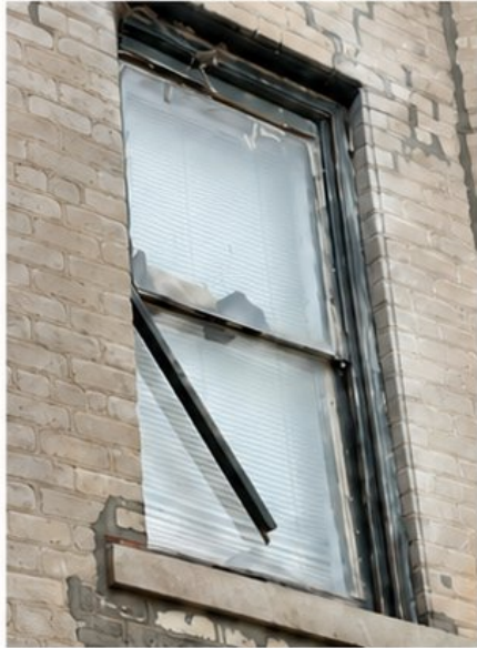
Existing Wood Window
