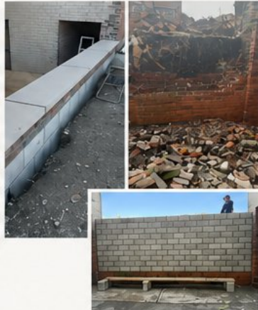
3 IMAGES – REPAIRED WALL & NEW LIMESTONE CAP
