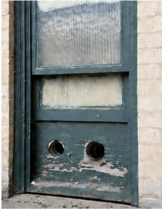
Existing Wood Window
