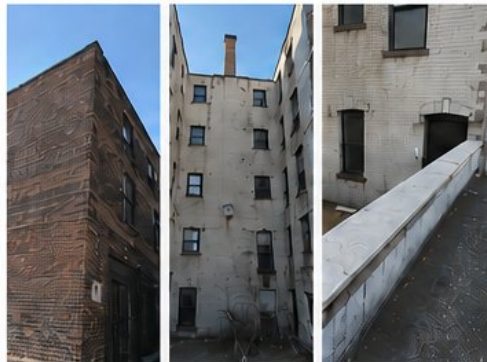
MURALS WILL UNIFY MISMATCHED BRICK AND CMU INFILL AREAS AND REDUCE VISUAL PROMINENCE OF ALTERATIONS.
