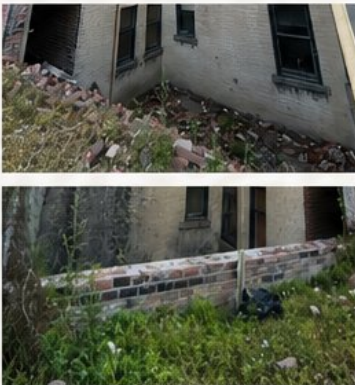
2 IMAGES – ORIGINAL RETAINING WALL
