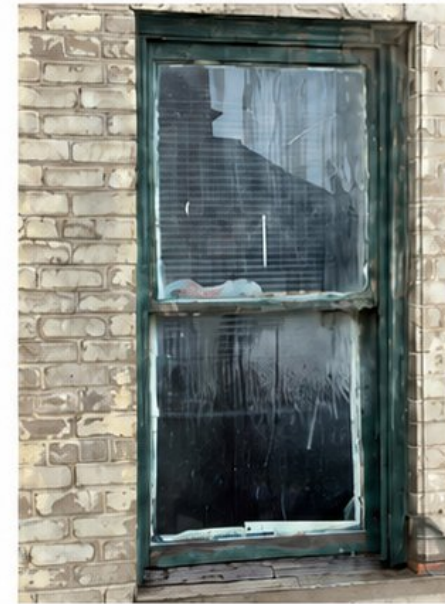
Existing Wood Window
