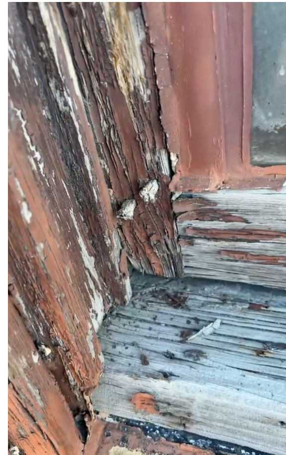
Detail view of existing historic wood sill, frame, and lower sash components, typical condition.
