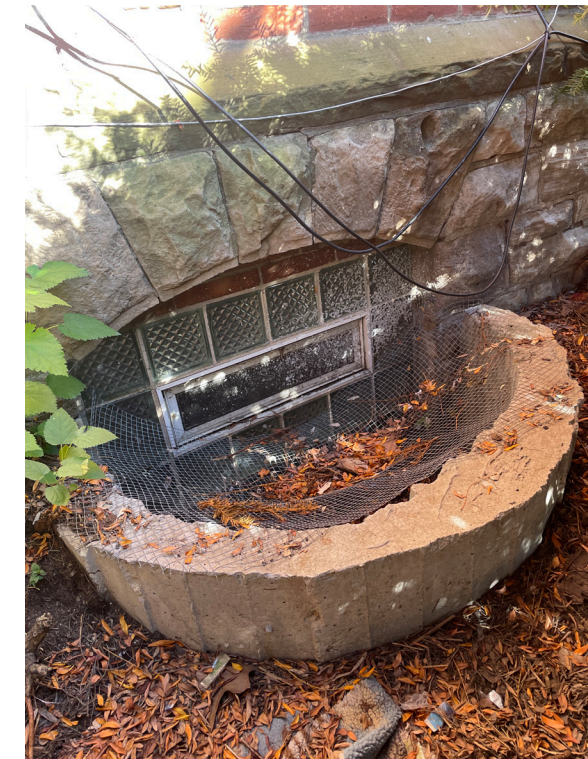
View of existing historic masonry opening #003 at Rectory, south elevation.
