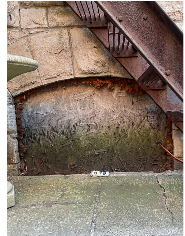
View of existing historic masonry opening #019 at Rectory, north elevation.
