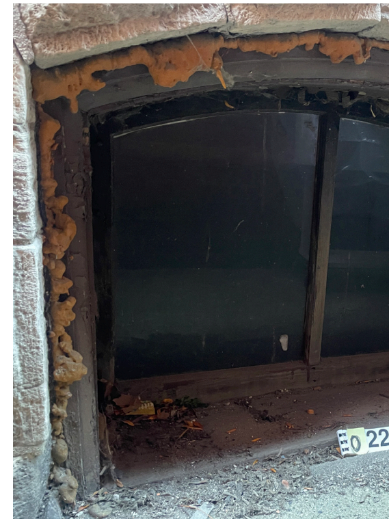
View of existing historic masonry opening #022 at Rectory, north elevation.
