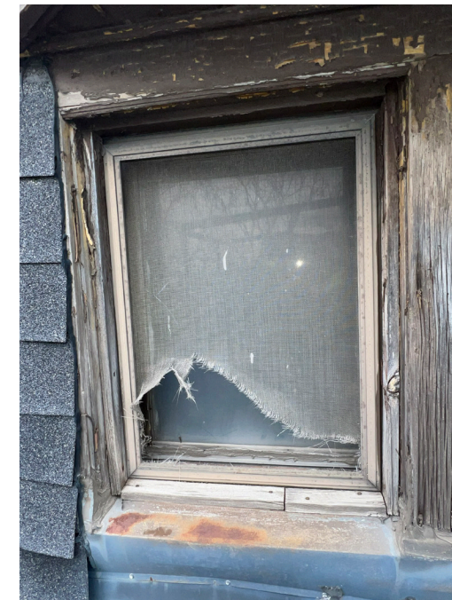
Detail view of existing historic wood window #400A.
