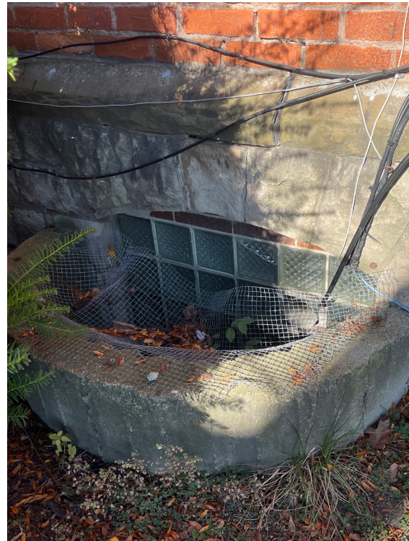
View of existing historic masonry opening #004 at Rectory, south elevation.
