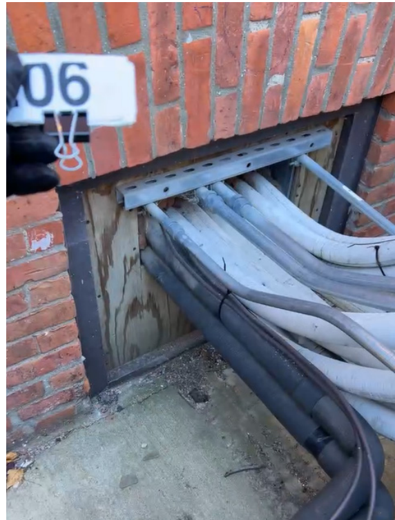
View of existing historic masonry opening #006 at Wellness Center/Convent, north elevation.
