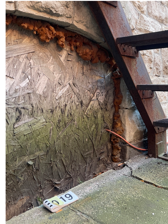
View of existing historic masonry opening #019 at Rectory, north elevation.
