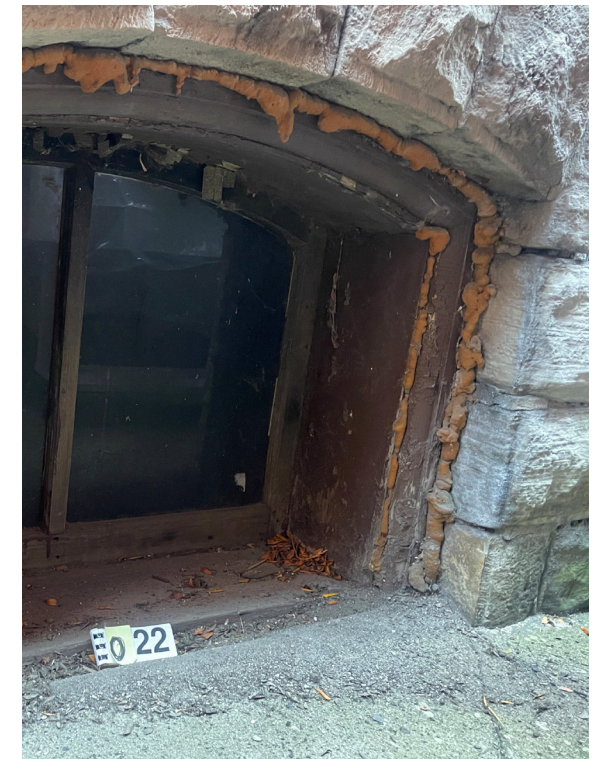
View of existing historic masonry opening #022 at Rectory, south elevation.
