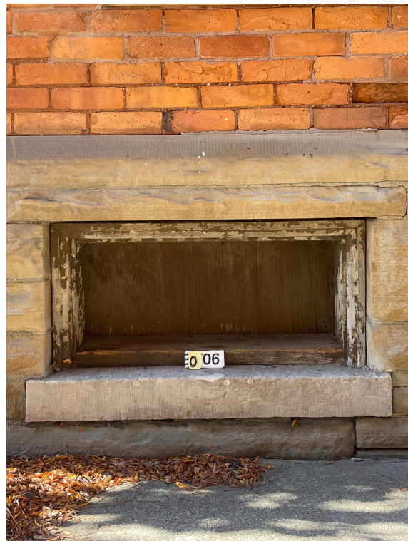
View of existing historic masonry opening #006 at Rectory, south elevation.
