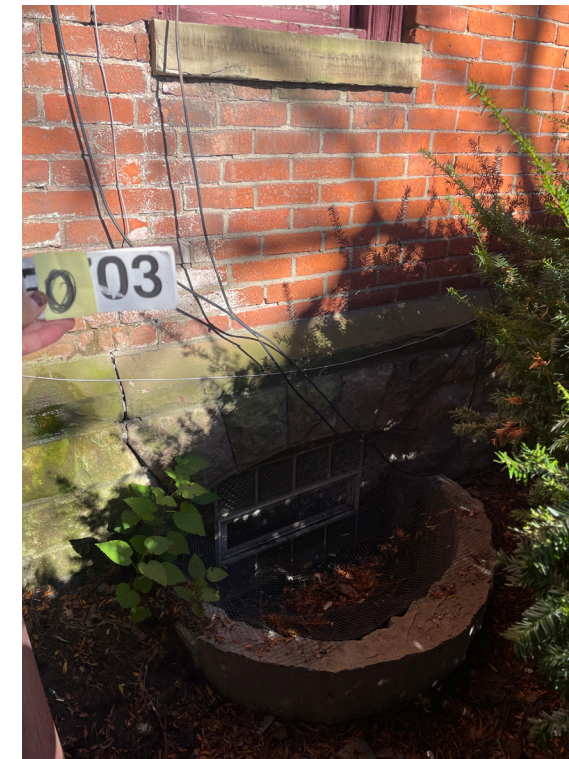
View of existing historic masonry opening #003 at Rectory, south elevation.
