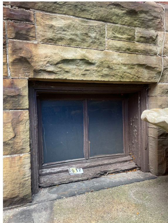
View of existing historic masonry opening #017 at Rectory/connector, west elevation.
