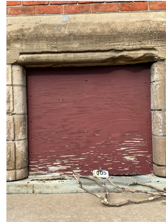
View of existing historic masonry opening #005 at Basilica/chapel, west elevation.
