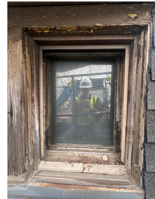
Detail view of existing historic wood window #400B.
