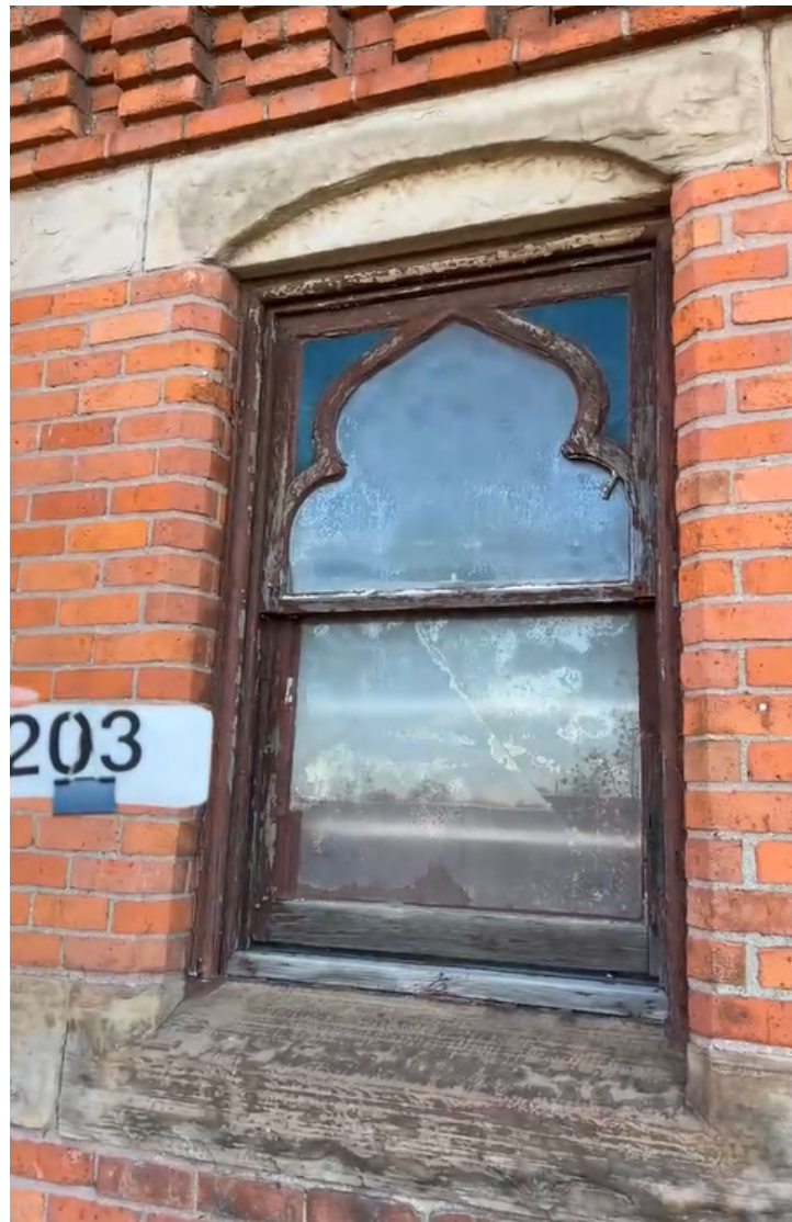
View of existing historic wood window #203 at Basilica (sacristy), 2nd floor, west elevation.
