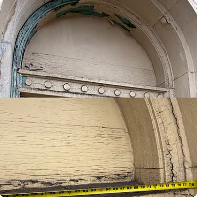
Existing conditions documentation revealed severe deterioration of original wood window assemblies beyond feasible repair.
