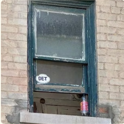
Existing conditions documentation revealed severe deterioration of original wood window assemblies beyond feasible repair.
