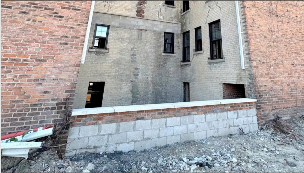
EXISTING CONDITIONS — Exposed retaining wall
