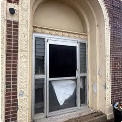
Existing conditions documentation revealed severe deterioration of original wood window assemblies beyond feasible repair.
