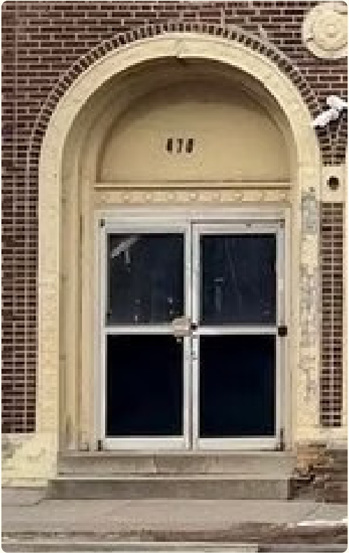
EXISTING CONDITIONS — Original entry doors
