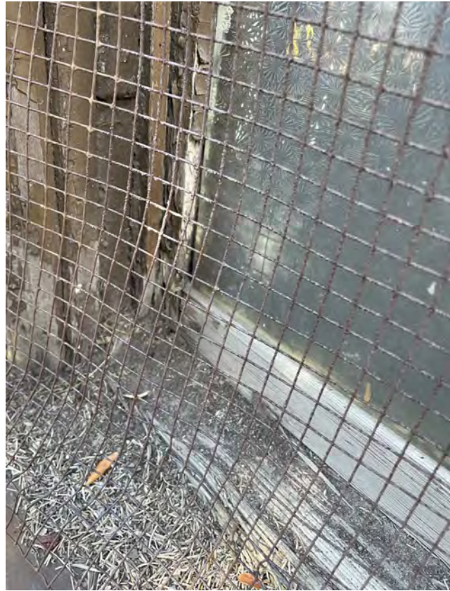
Photo: Window 004, exterior weight pocket detail. Typ. inherent flaw condition at historic wood dbl-hung units.
