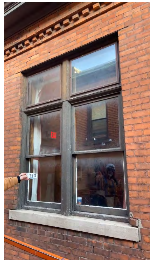
Photo: Window 113 (ABCD), exterior view.
