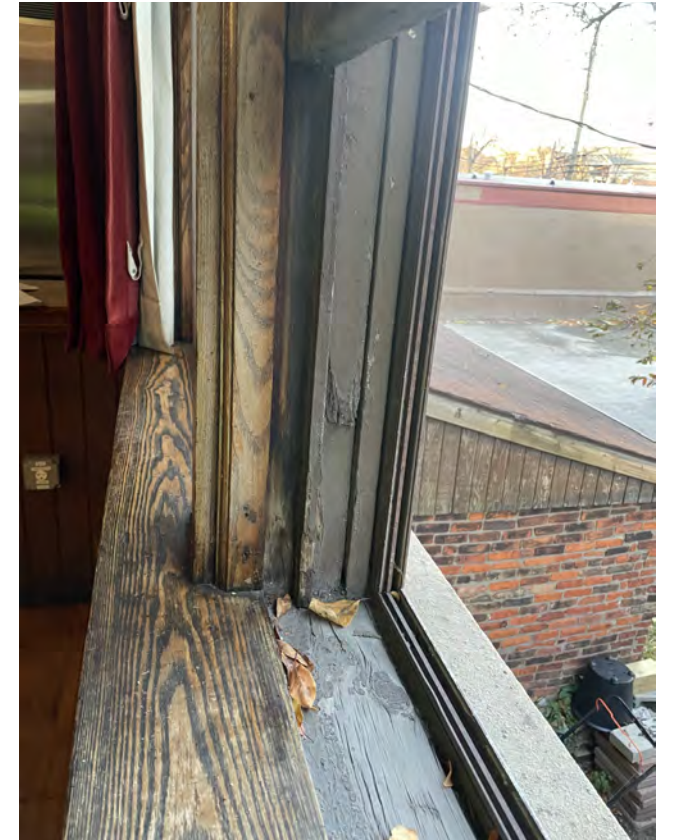
Photo: Window 107 (C), exterior weight pocket detail. Typ. inherent flaw condition at historic wood dbl-hung units.
