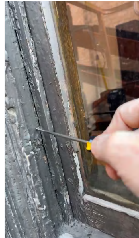
Photo: Window 112 (C), exterior weight pocket detail. Typ. inherent flaw condition at historic wood dbl-hung units.
