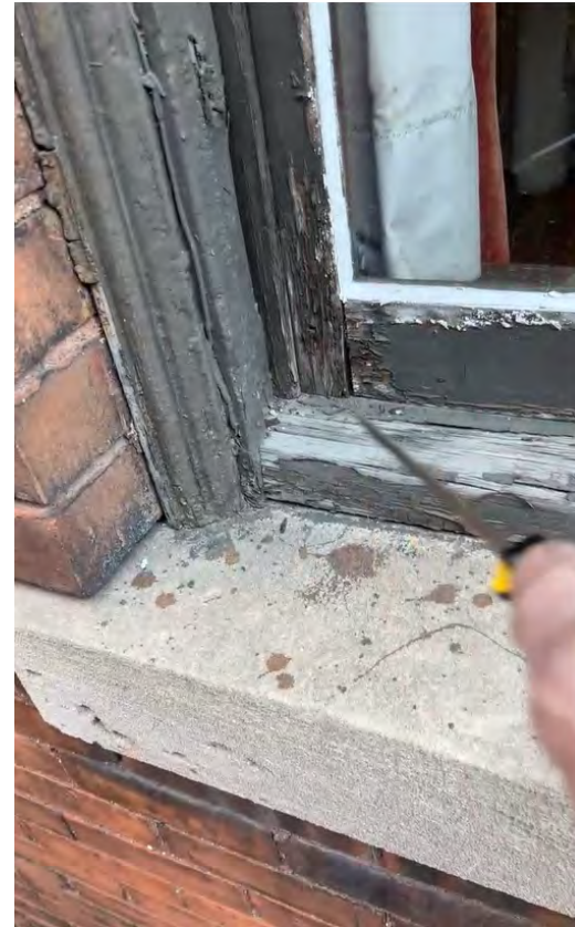
Photo: Window 113 (C), exterior weight pocket detail. Typ. inherent flaw condition at historic wood dbl-hung units.
