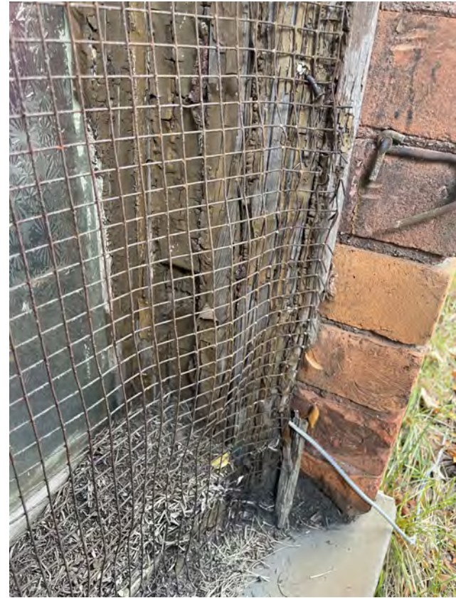
Photo: Window 004, exterior weight pocket detail. Typ. inherent flaw condition at historic wood dbl-hung units.
