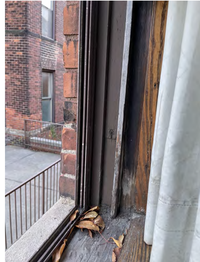
Photo: Window 107 (C), exterior weight pocket detail. Typ. inherent flaw condition at historic wood dbl-hung units.
