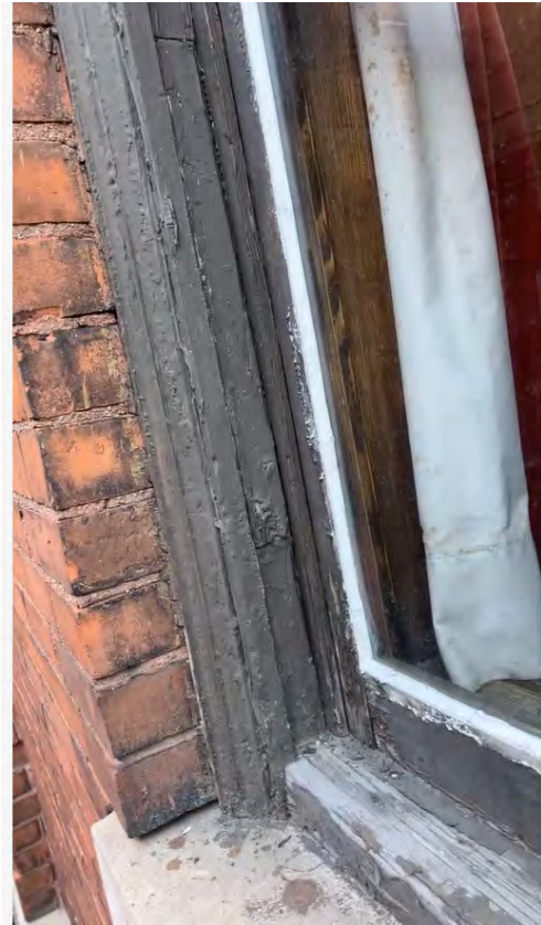
Photo: Window 113 (C), exterior weight pocket detail. Typ. inherent flaw condition at historic wood dbl-hung units.
