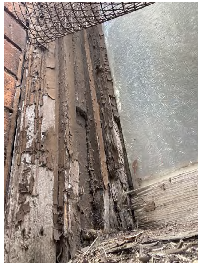
Photo: Window 004, exterior weight pocket detail. Typ. inherent flaw condition at historic wood dbl-hung units.
