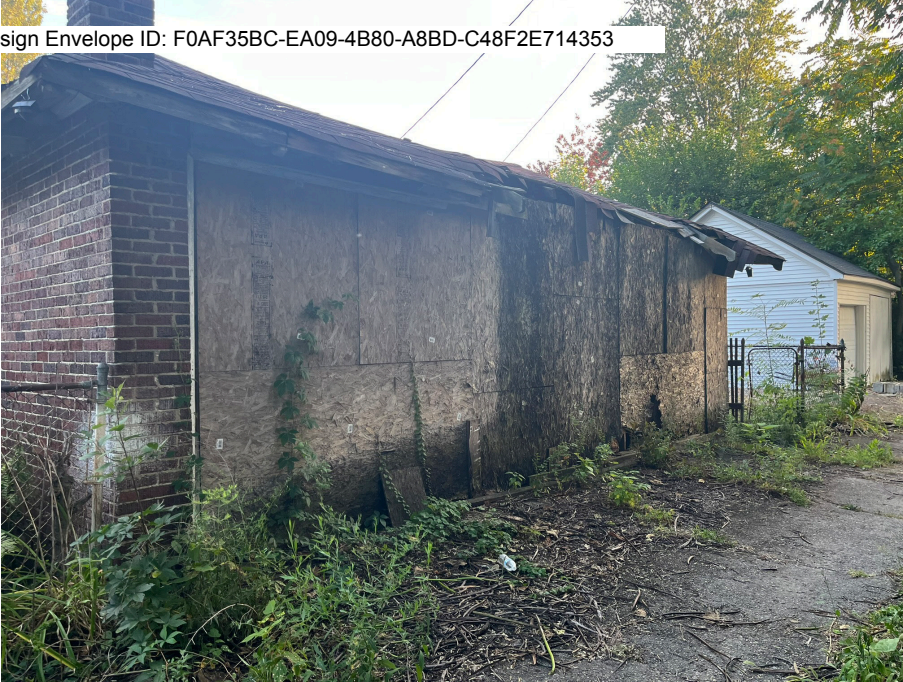
IMAGE 07: NORTH ELEVATION EVIDENCE OF DOOR ALONG ALLEY SIDE OF GARAGE
