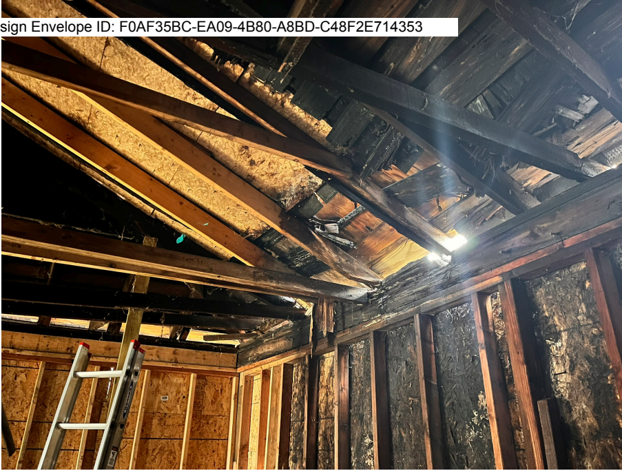
IMAGE 16: PLYWOOD TO SECURE PROPERTY AND STRUCTURE - WATER DAMAGE ON SOME PLYWOOD ELEMENTS DUE TO HOLE IN ROOF - MULTIPLE UNCONNECTED SUPPORT ELEMENTS
