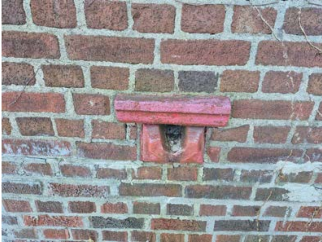
Porch drainage spout (typ. condition)
