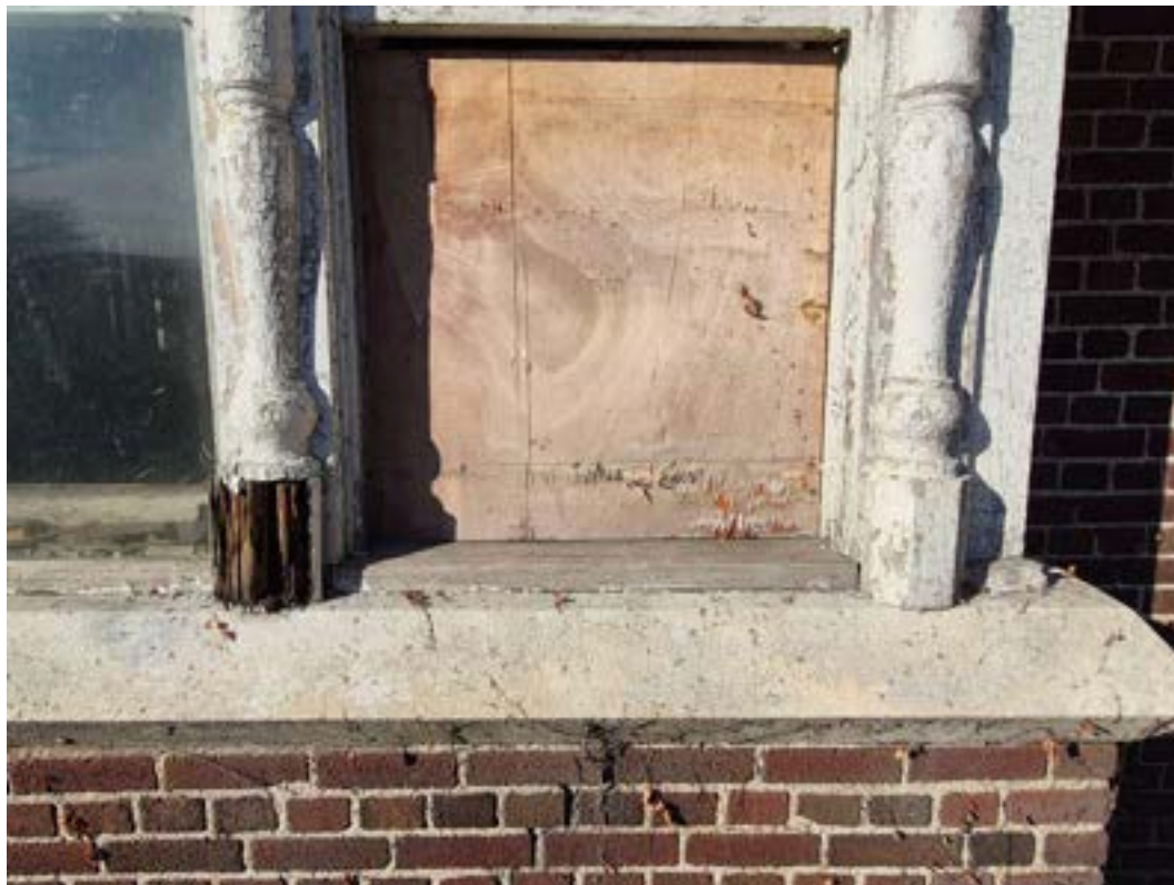
Damage to front window trim; missing partial window frame
