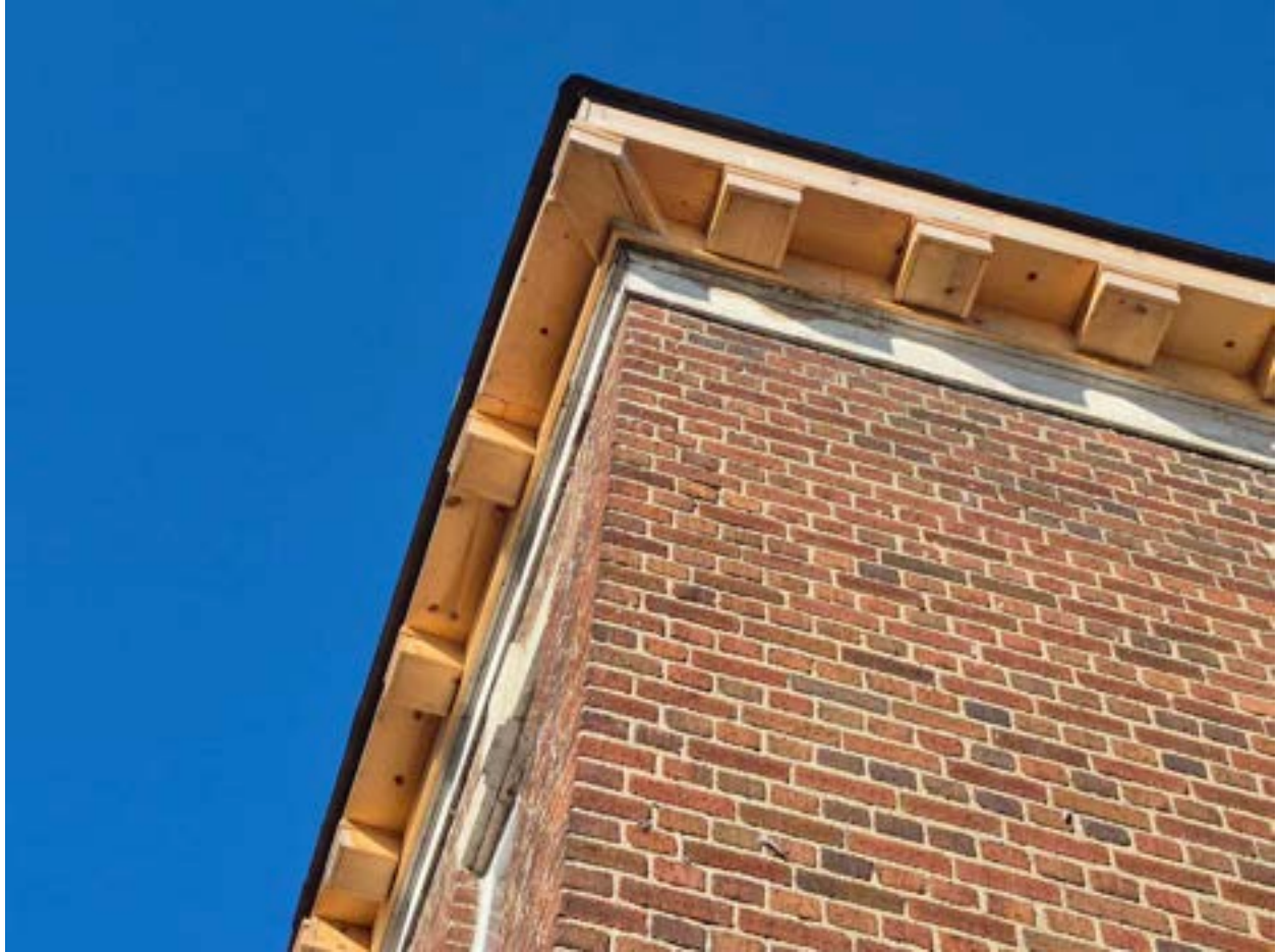
Soffit detail, southwest corner; note new dentil spacing at front
