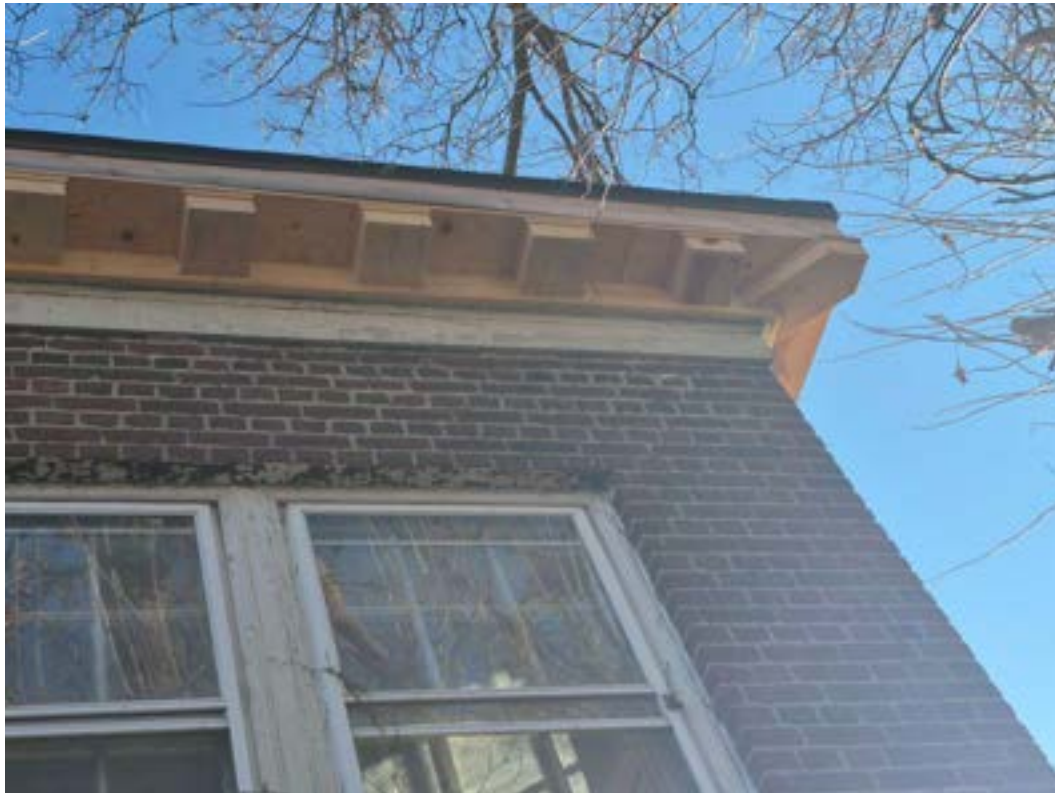
Rear soffit and dentiling
