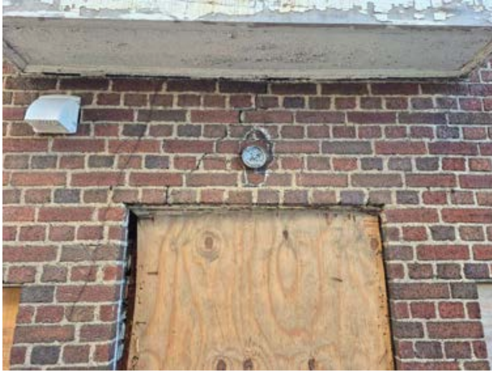
East side entry door: note cracks in masonry joints
