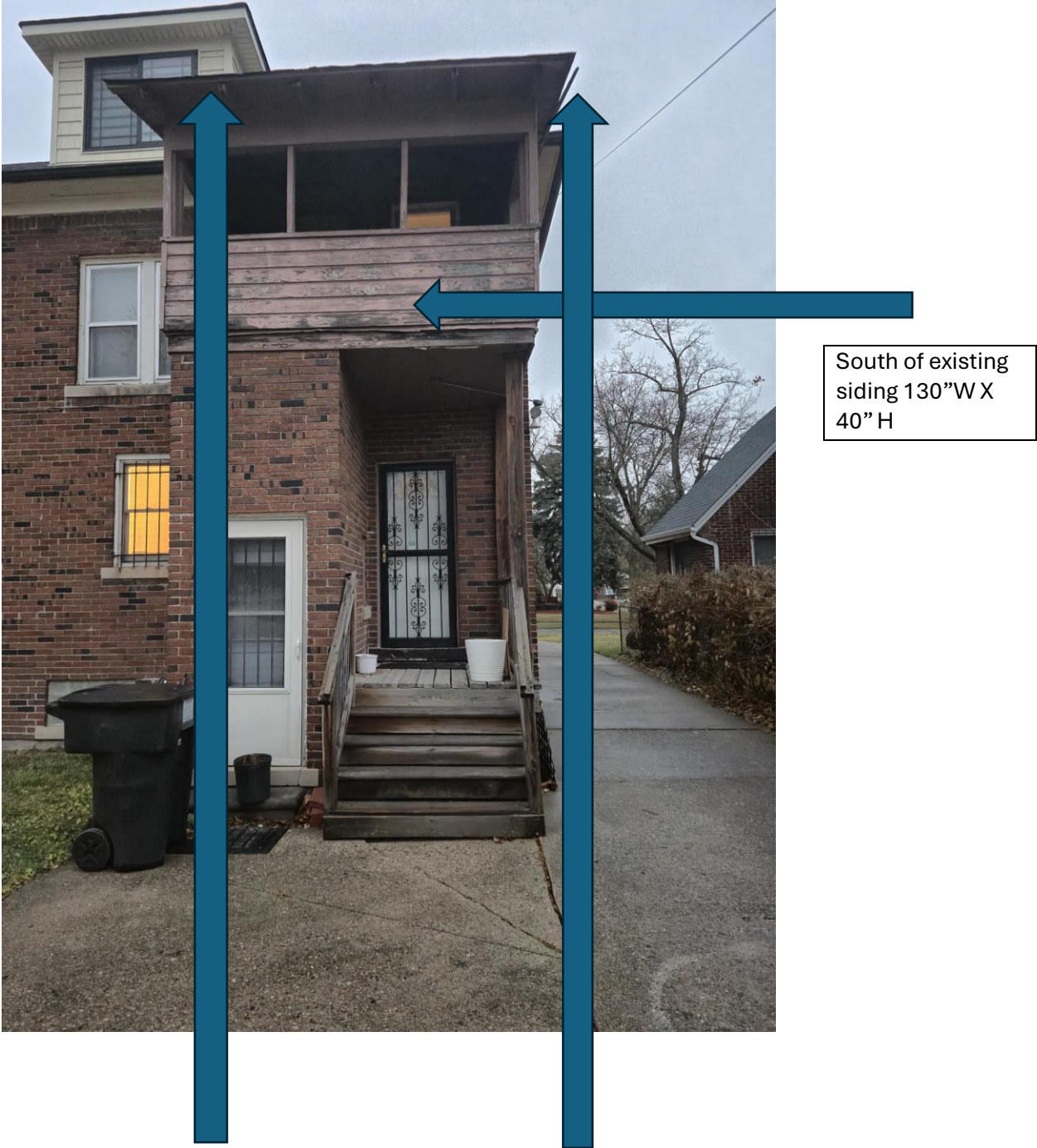
South Overhang (left arrow) is 20" and east/west overhang (right arrow) is 8" each side
