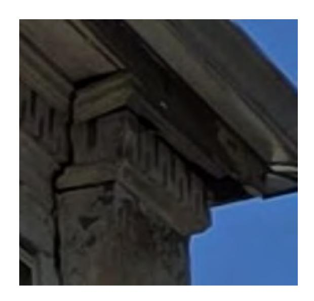
West elevation: Observed separation at the extension joint resulting from foundation instability
