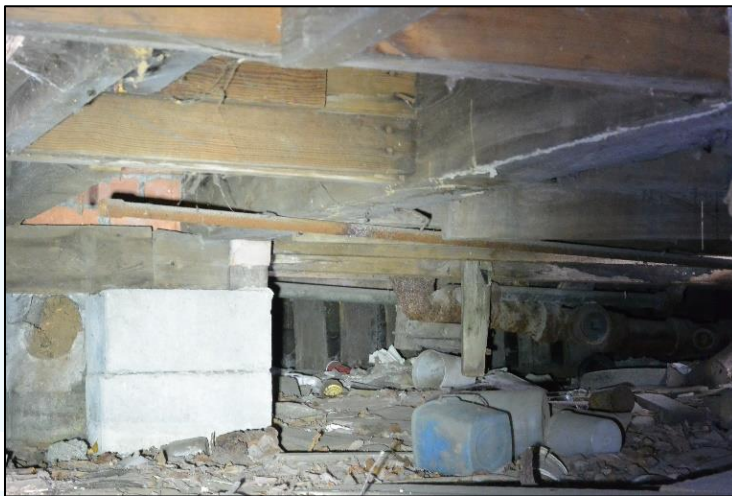
PHOTO NO. 12: Crawl space.
