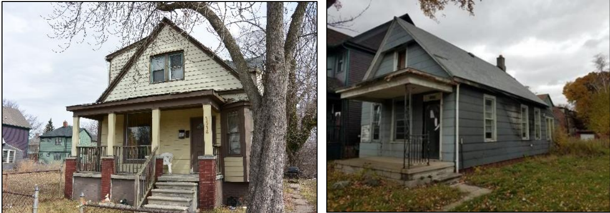
PHOTO NO. 1: Residential structures at 1514 (left) and 1532 (right) Van Dyke St, Detroit, Michigan. (Front entrances, west elevations, face Van Dyke St.)
