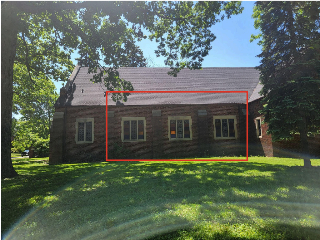
North Elevation of windows
