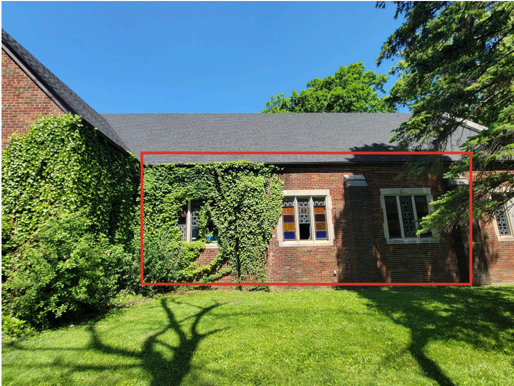
South Elevation of windows
