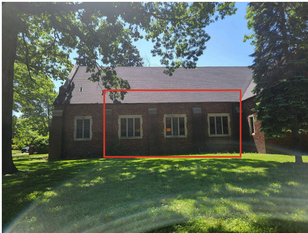
North Elevation of windows
