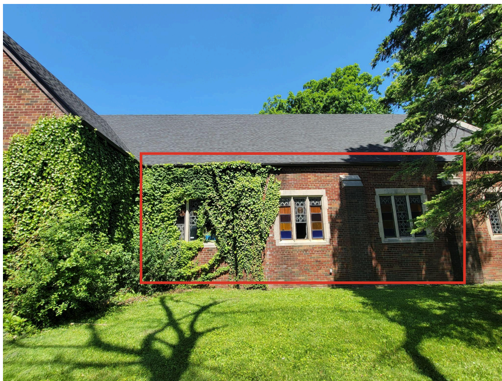
South Elevation of windows
