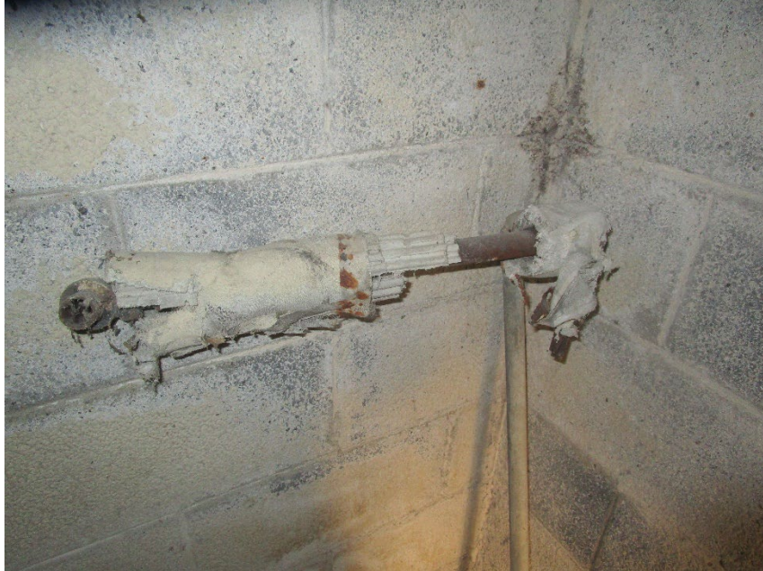
Asbestos-containing pipe insulation.
