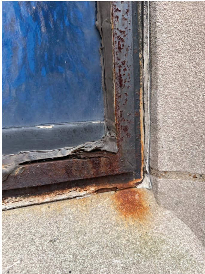
EXISTING EXTERIOR FRAME/CAULK CONDITIONS (TYP.)
