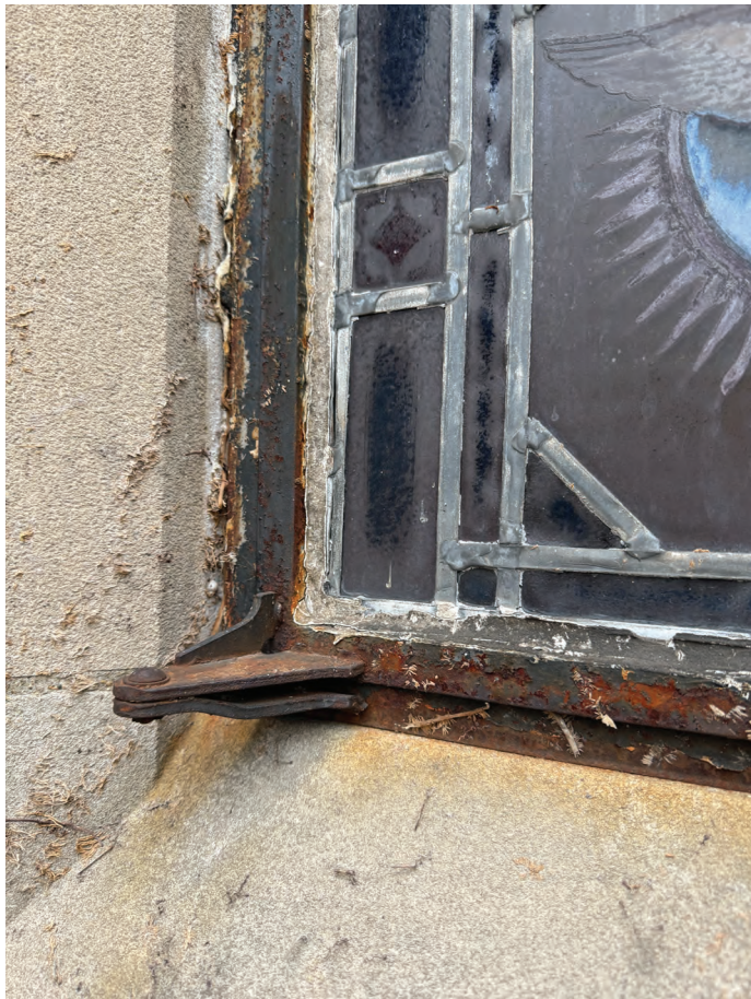
EXISTING EXTERIOR FRAME/CAULK CONDITIONS (TYP.)
