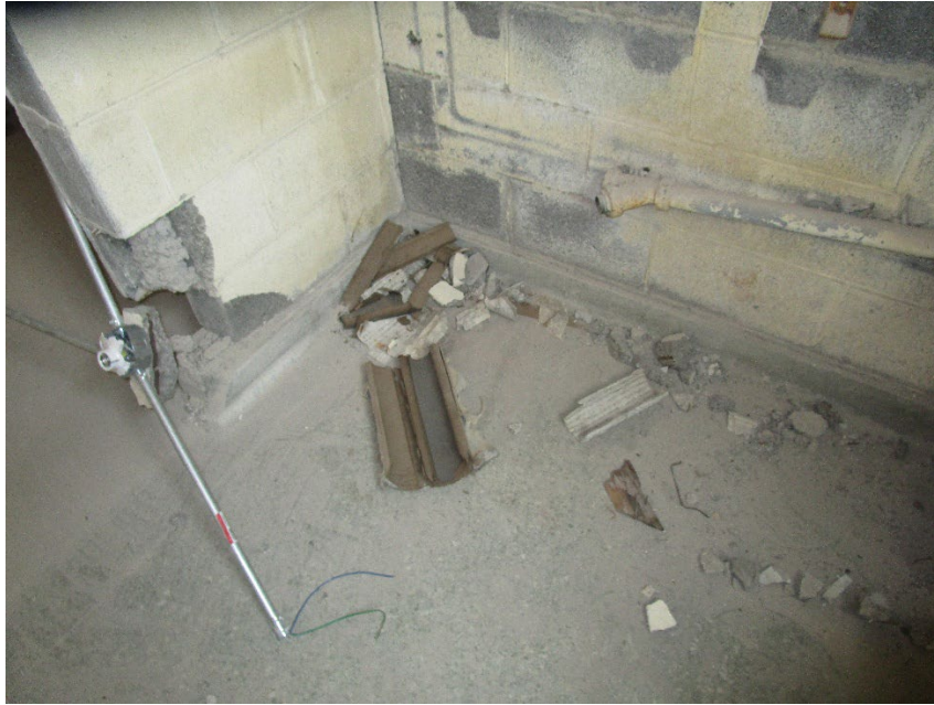
Asbestos-containing pipe insulation.
