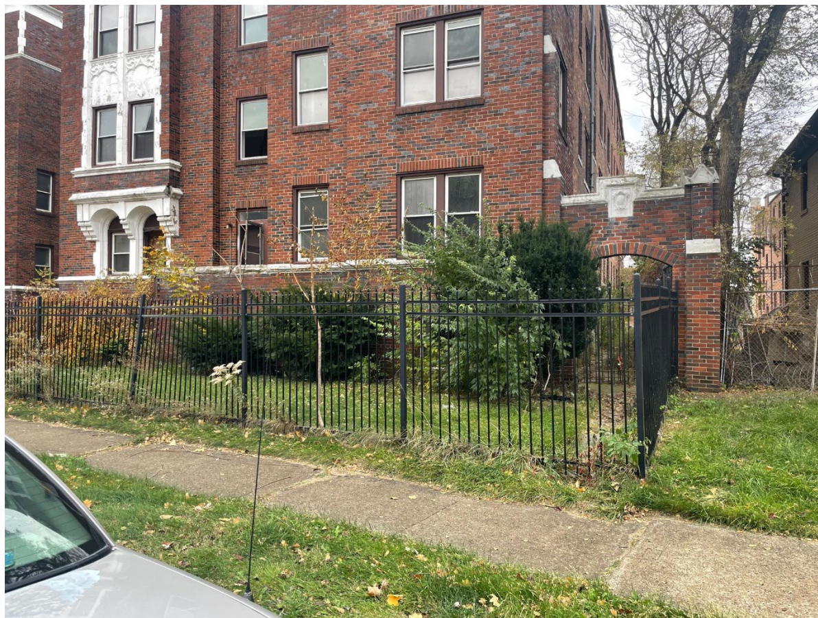
Photo 3: View of existing adjacent property fence at 725 Whitmore
