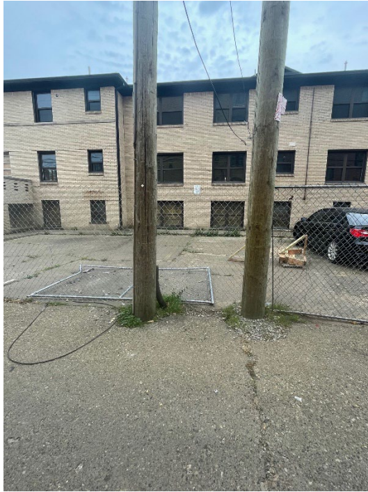
Photo 1: Looking at building from south alley
