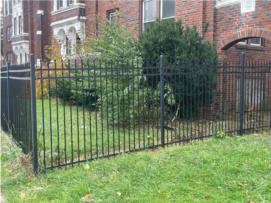
Photo 2: View of existing adjacent property fence at 725 Whitmore
