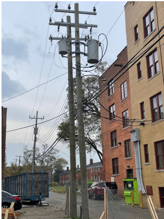
Photo 2: Looking at existing utility poles along alley from Third Avenue
