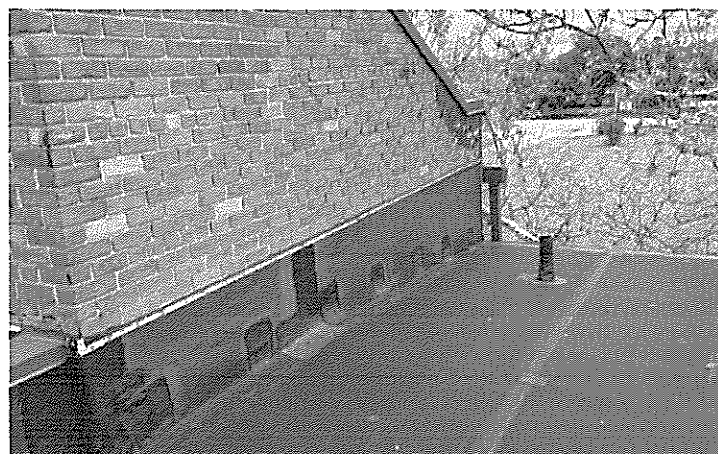
OVERALL VIEW SLOPES TO GUTTER
