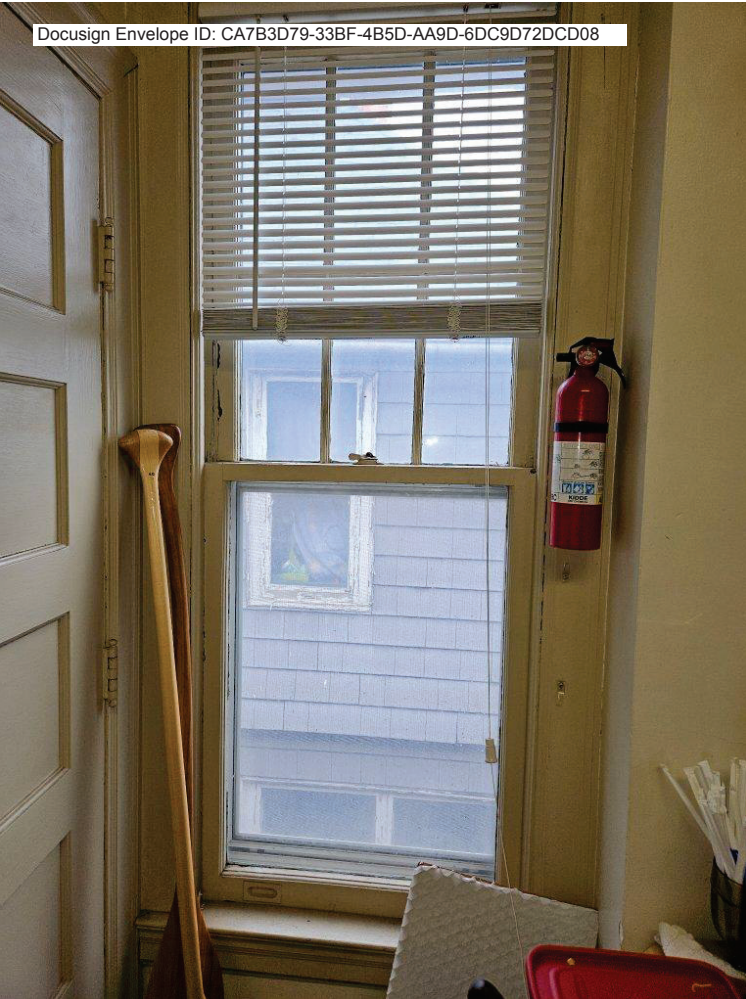
Unit 201 (kitchen) Interior / Exterior New grilles on interior only (3w x 2h) to match existing grille pattern
