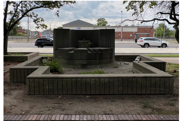
Water Fountain Restoration
