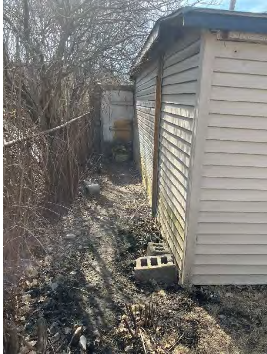
Existing photo – east side
