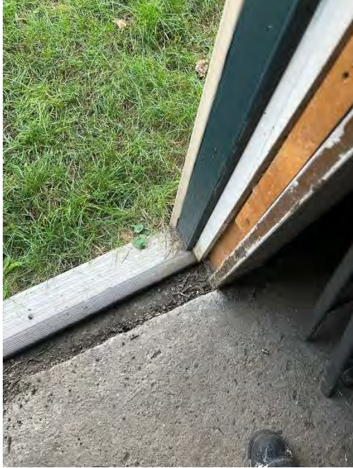
Level of exterior grade compared to slab
