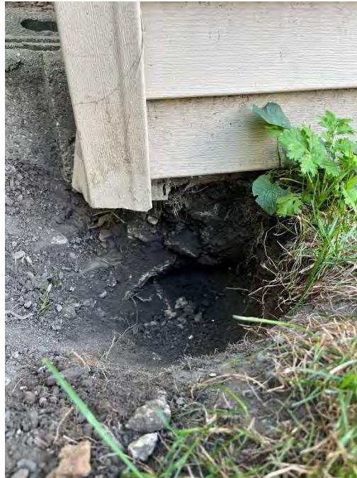
Test pit showing bottom of slab +/- 8" below
