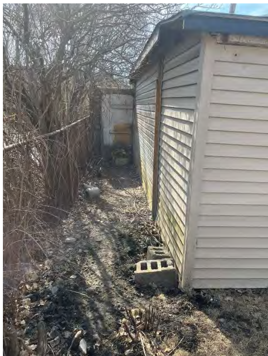
Existing photo – east side
