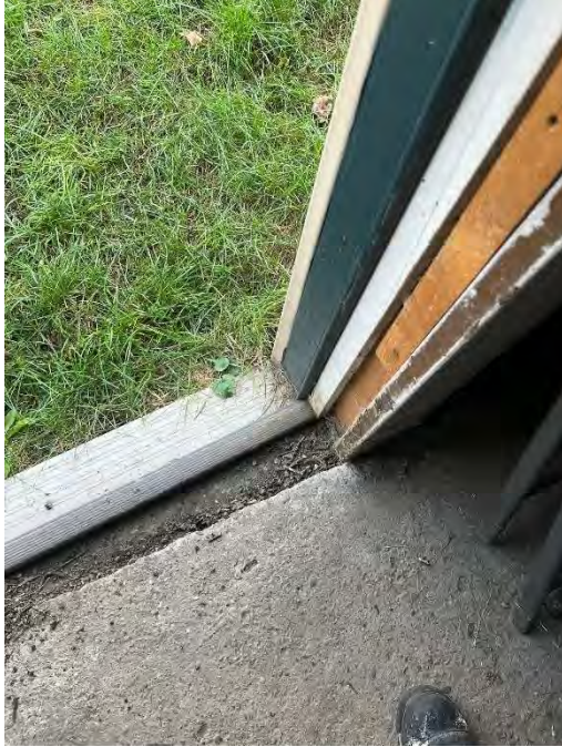
Level of exterior grade compared to slab
