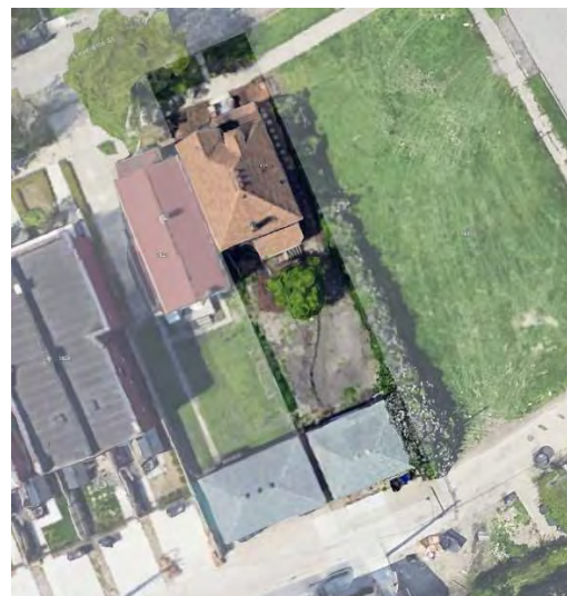
Primary Structure and Garage
