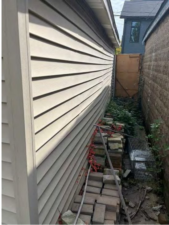
Existing photo – west side
