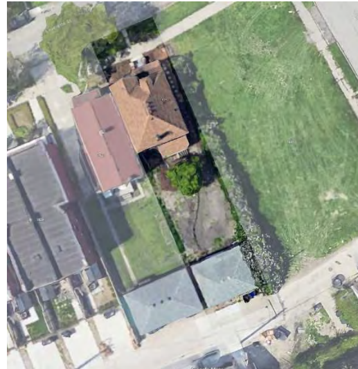
Primary Structure and Garage
