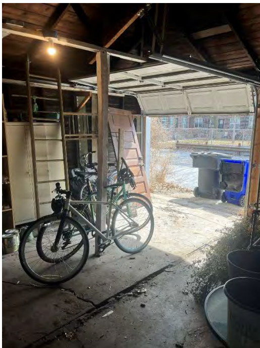
Temporary column installed to support roof
