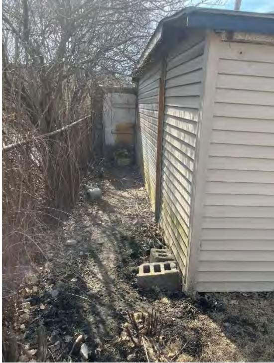
Existing photo – east side
