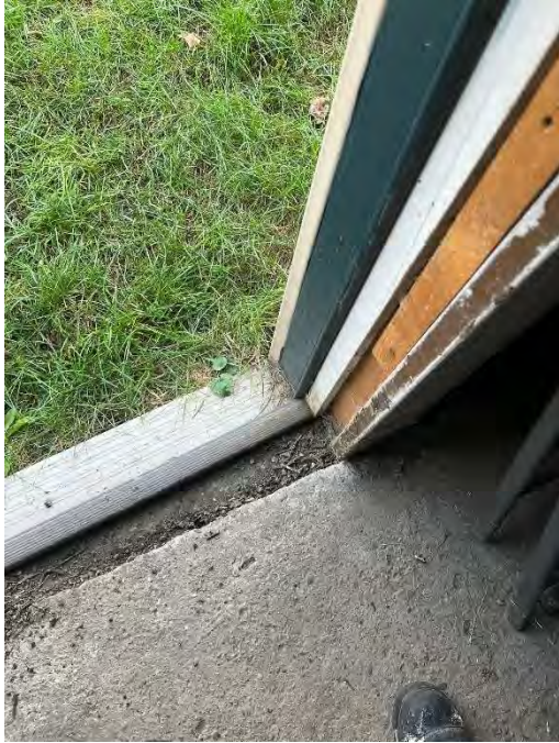
Level of exterior grade compared to slab
