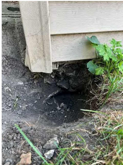
Test pit showing bottom of slab +/- 8" below
