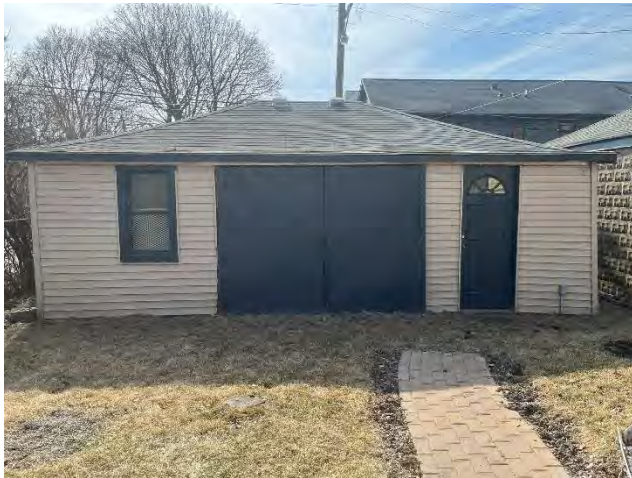
Existing photo - north, rear yard side
