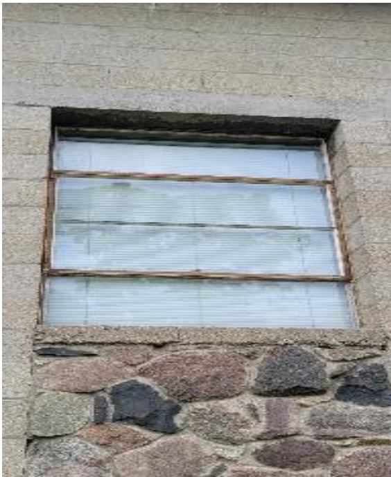
Window # W1.2 Area: OFFICE 212 Size: ~36 x 58 Sill: Int 5" sill
