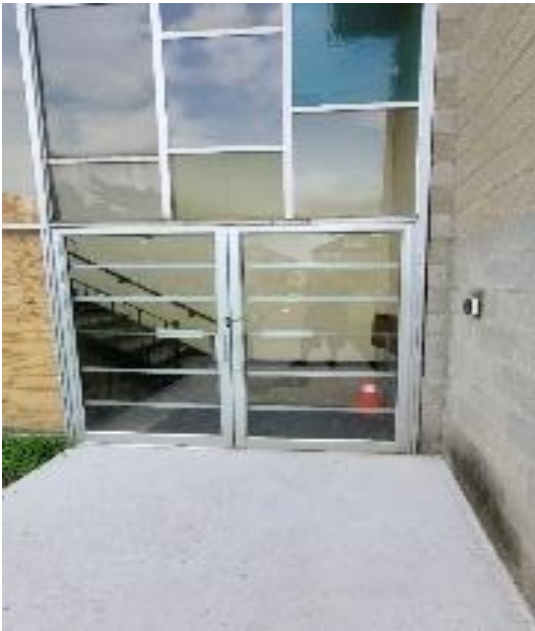
Window #: W7.2 Area: ENTRY/ STAIRS Size: 38 x 12 Sill: 5" double sill
