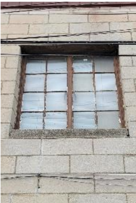
Window #: W5.6 Area: Gathering Space Size (H x W): ~40 x 56 Sill/ Mullion details: Mullions 1 ½" x ¼"; 4" double sill
