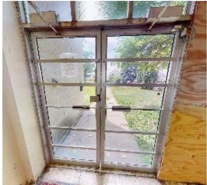
Window #: W7.2 Area: ENTRY/ STAIRS Size: 38 x 12 Sill: 5" double sill
