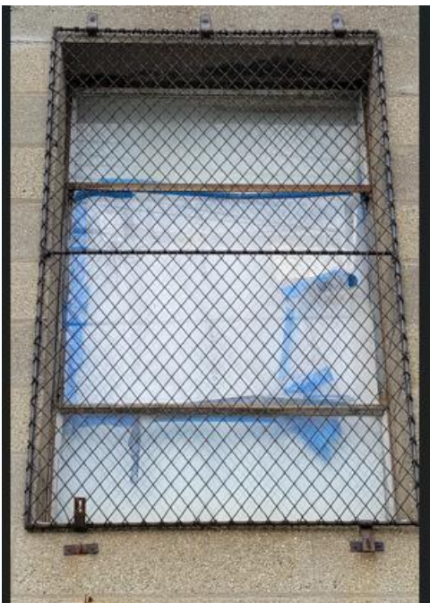
Window # W2.3 Area: OFFICE 217 Size: 66 x 54 Int 5" sill
