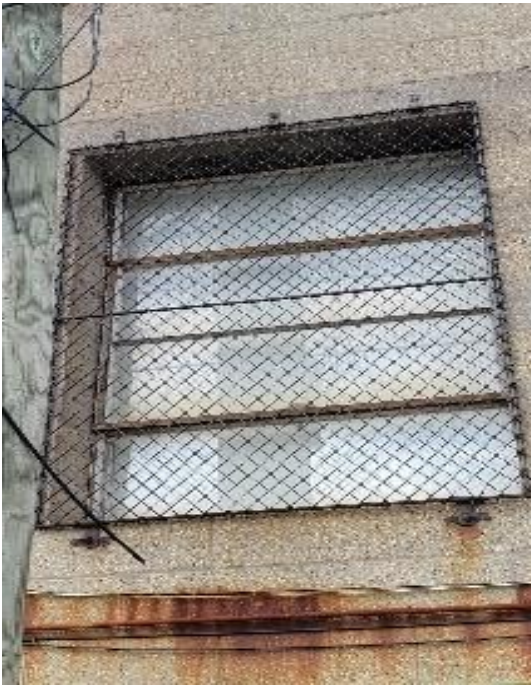
Window #: W5.5 Area: Storage Size (H x W): ~40 x 56 Sill/ Mullion details: Mullions 1 ½" x ¼"; 4" double sill
