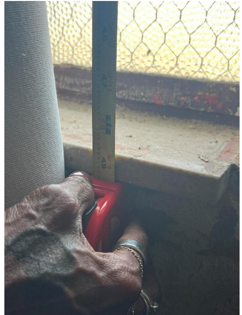
Window #: W5.5 Area: Storage Size (H x W): ~40 x 56 Sill/ Mullion details: Mullions 1 ½" x ¼"; 4" double sill
