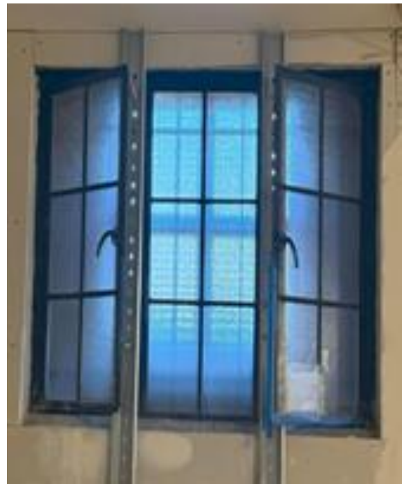
Window #: W5.6 Area: Gathering Space Size (H x W): ~40 x 56 Sill/ Mullion details: Mullions 1 ½" x ¼"; 4" double sill
