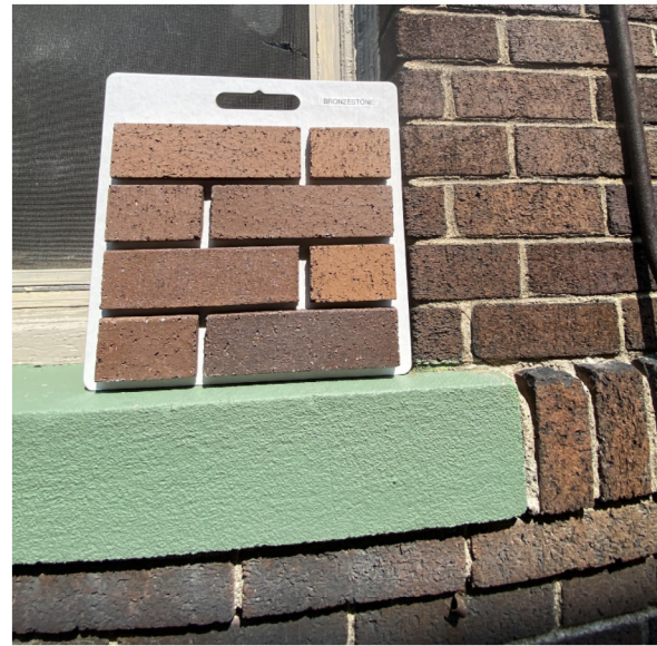
INFILL BRICK TO MATCH EXISTING INTERSTATE BRICK - BRONZESTONE & WALNUT BLEND - SHOWN IN SAMPLE BOARDS
