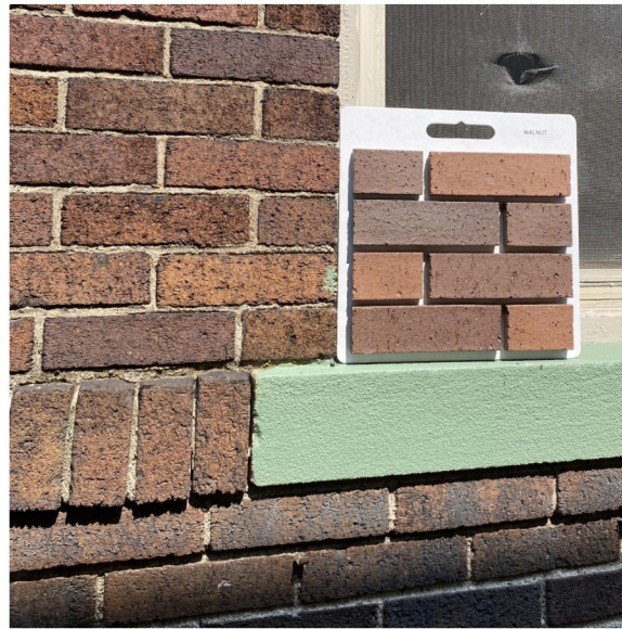
INFILL BRICK TO MATCH EXISTING INTERSTATE BRICK - BRONZESTONE & WALNUT BLEND - SHOWN IN SAMPLE BOARDS
