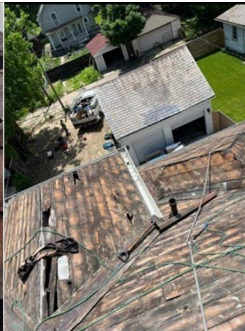
Wood damage underneath previous slate
