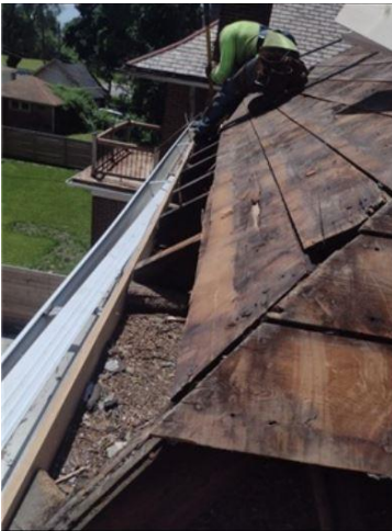
Replacing damaged wood
