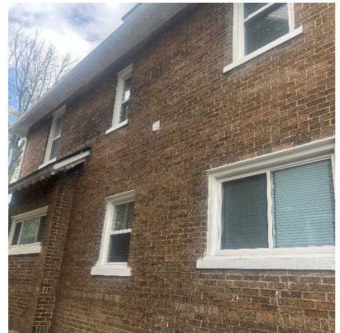
Site Photo 3, by Applicant: (west) side elevation showing replaced vinyl windows.
