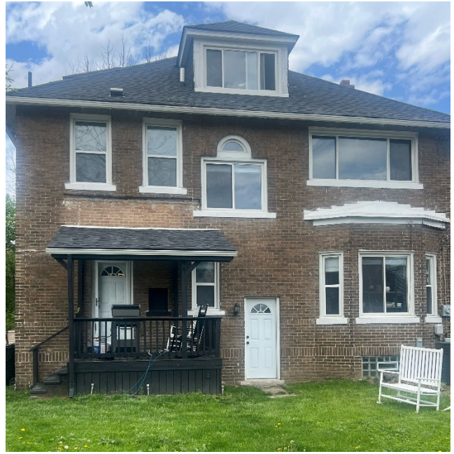
Site Photo 2, by Applicant: (South) rear side elevation showing replaced vinyl windows, altered rear porch and replaced rear door.
