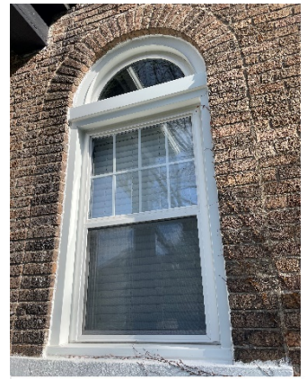
Site Photo 4, by Staff April 19, 2024: (North) front elevation showing detail of thick, vinyl coil stock around brick mold and seam, and color tinted transom, proposed
