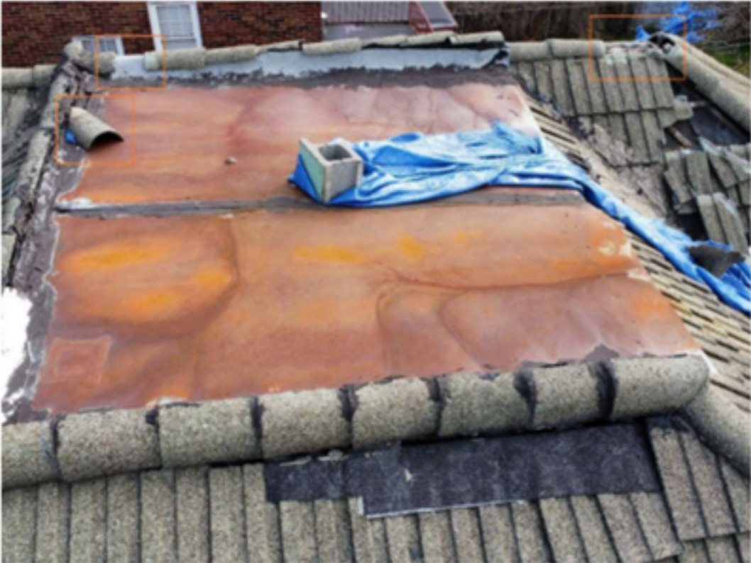
Photograph 17: View of missing and displaced ridge tiles.
