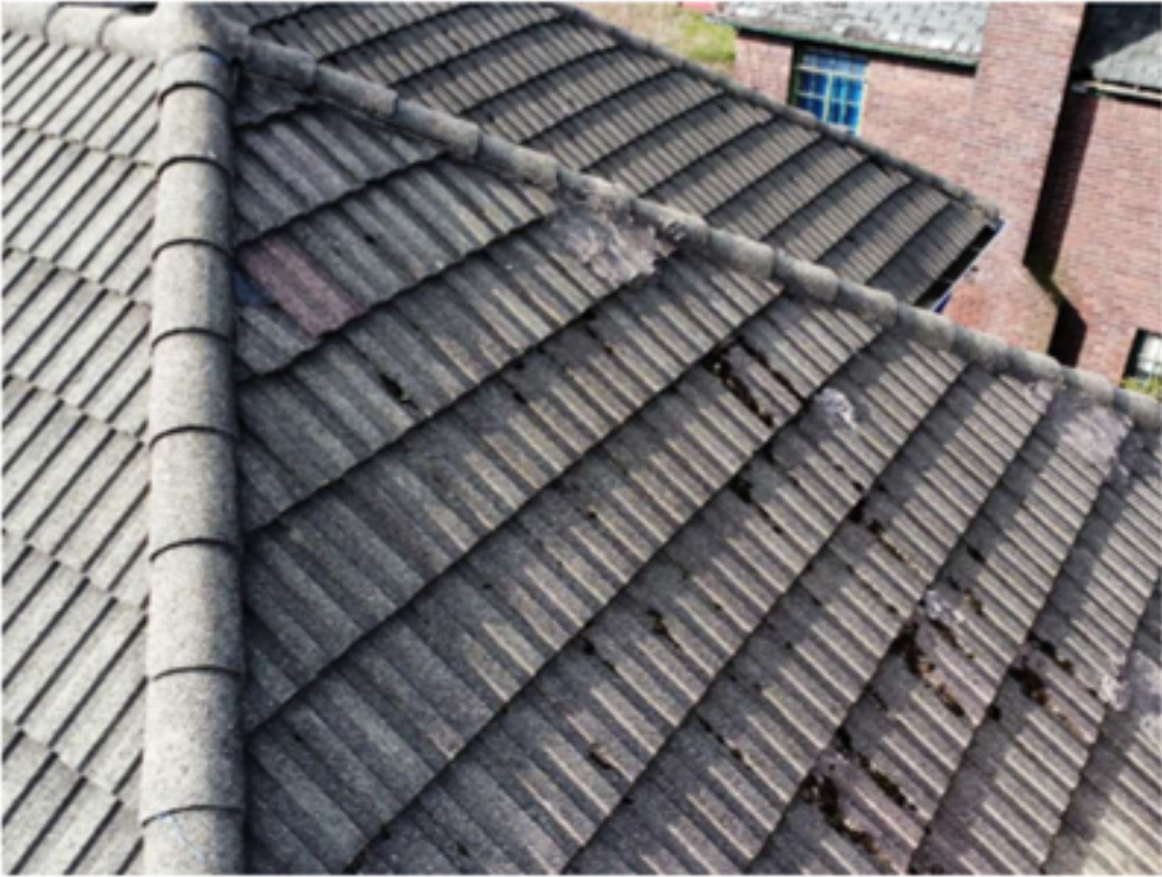
Photograph 7: View of historical repairs.
