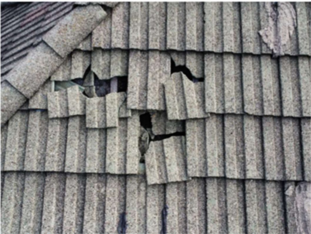
Photograph 14: View of cracked roof tiles on roof slope N.
