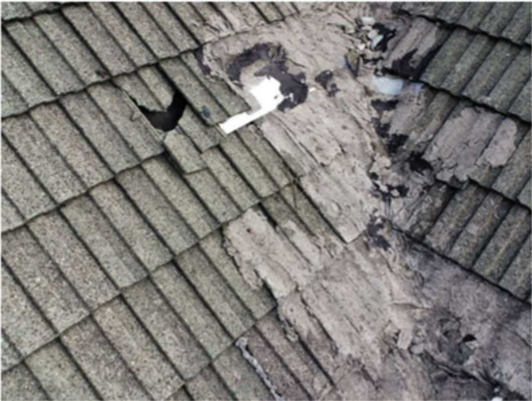
Photograph 11: View of historical repairs.
