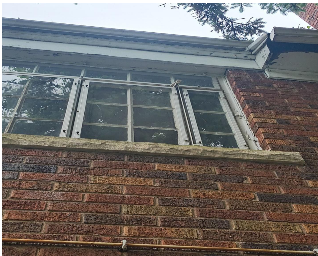
Photos of the rotten wood.
