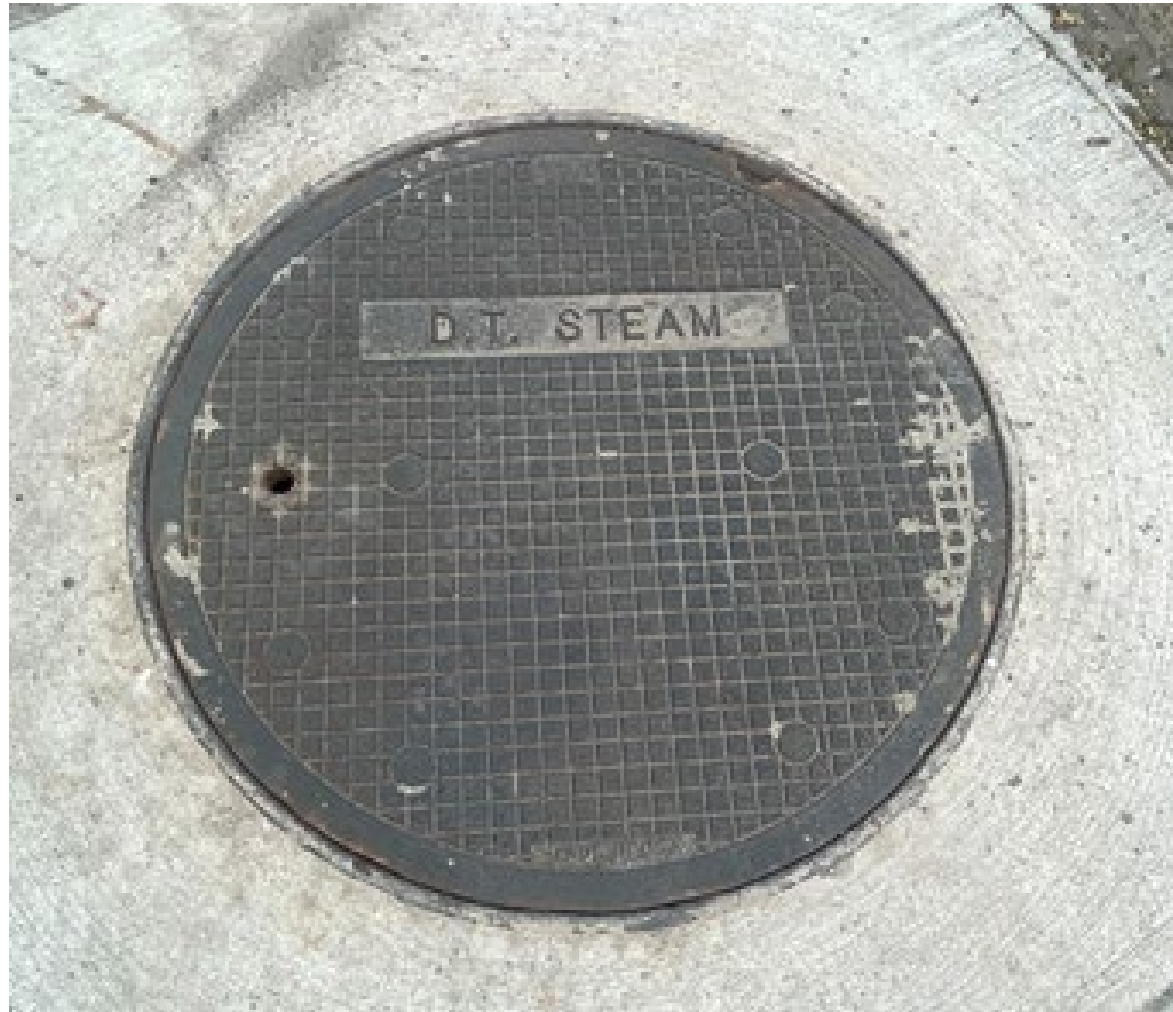
Detroit Thermal cast iron manhole frame and cover
