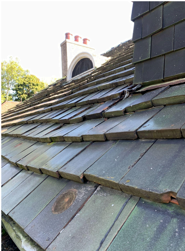
Damaged tile to east of front double dormer and view of barrel window
