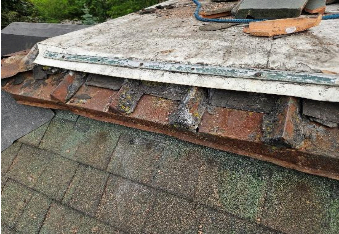
Tin flat roof coping rusted, asphalt shingles where tile once was
