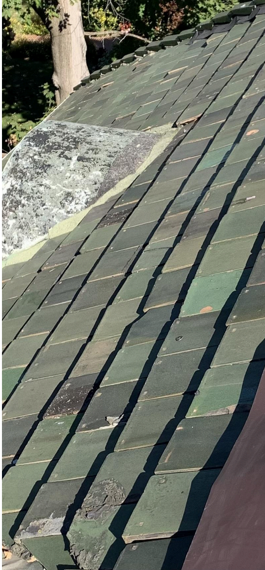
Damaged tile and barrel arch window on north side facing east. Coping from flat roof extended with brown aluminum.
