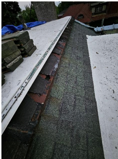
broken tiles in front of shed dormer. Rusted flat roof combing.
