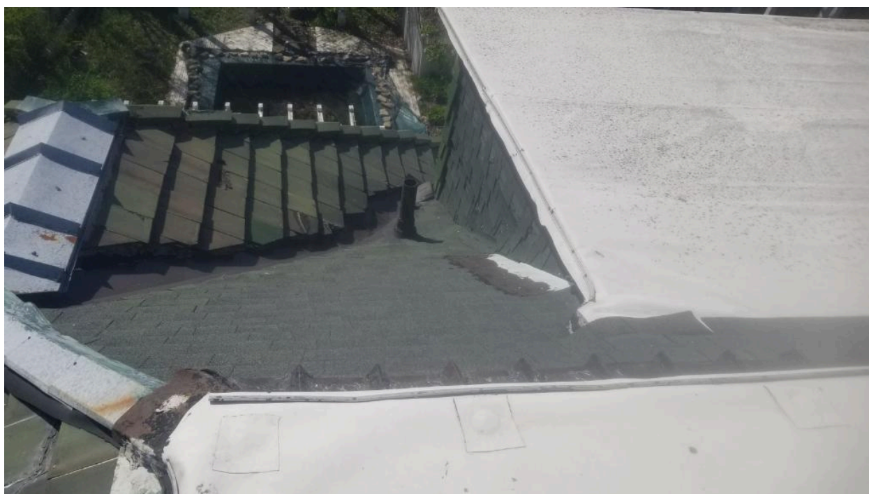
East side of south facing shed dormer . Roof and siding are shingled where roof and siding tile once were.
