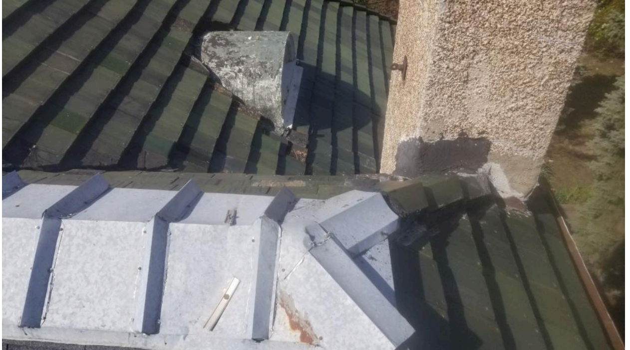
Damaged tile to east of front double dormer and view of barrel window
