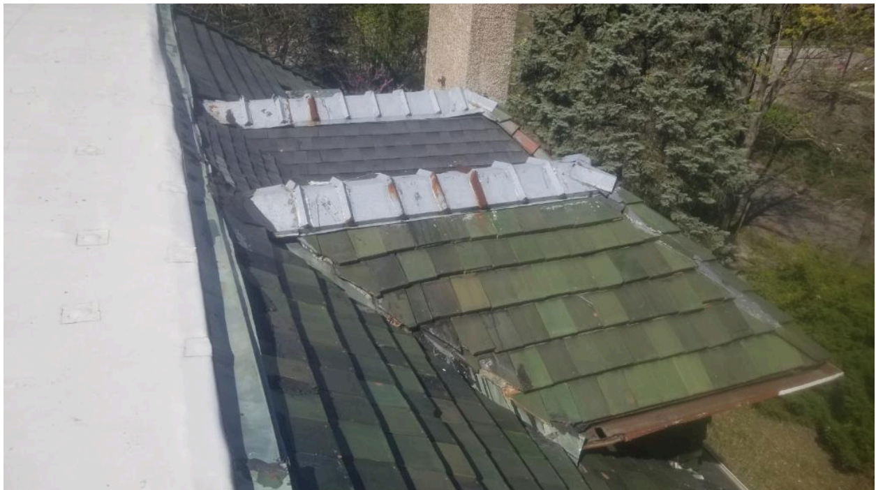
Damaged tile, rusted gutter, damaged flashing on east side of front double dormer
