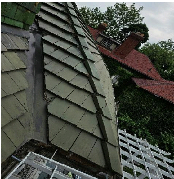
Hip tiles broken and cemented to roof tiles
