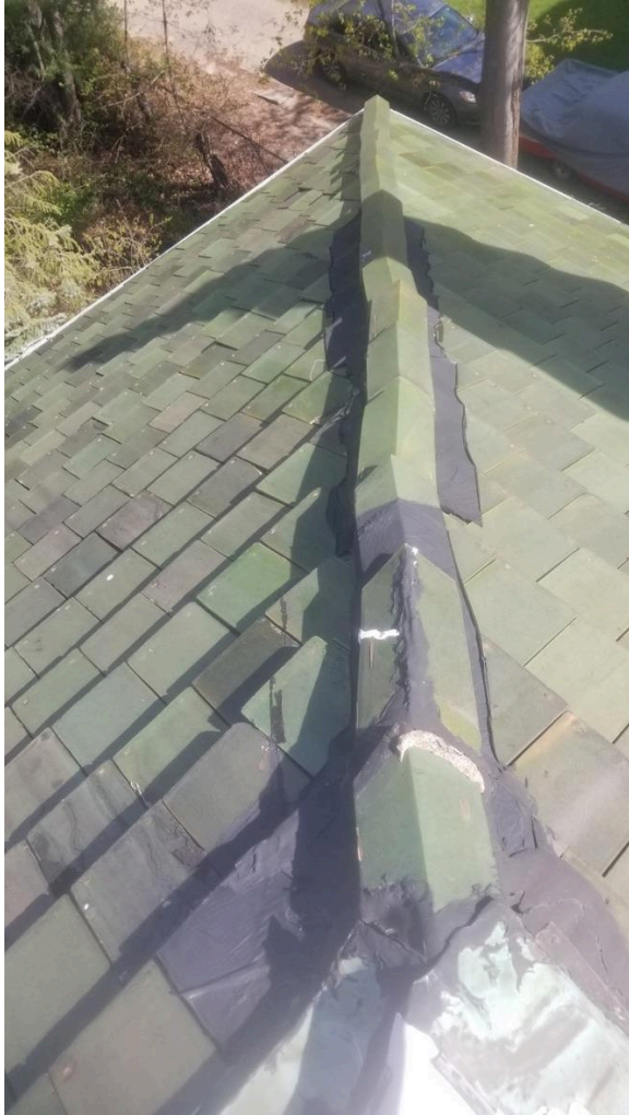
North east hip and surrounding tiles show damage and repair by tar and ice and water shield.
