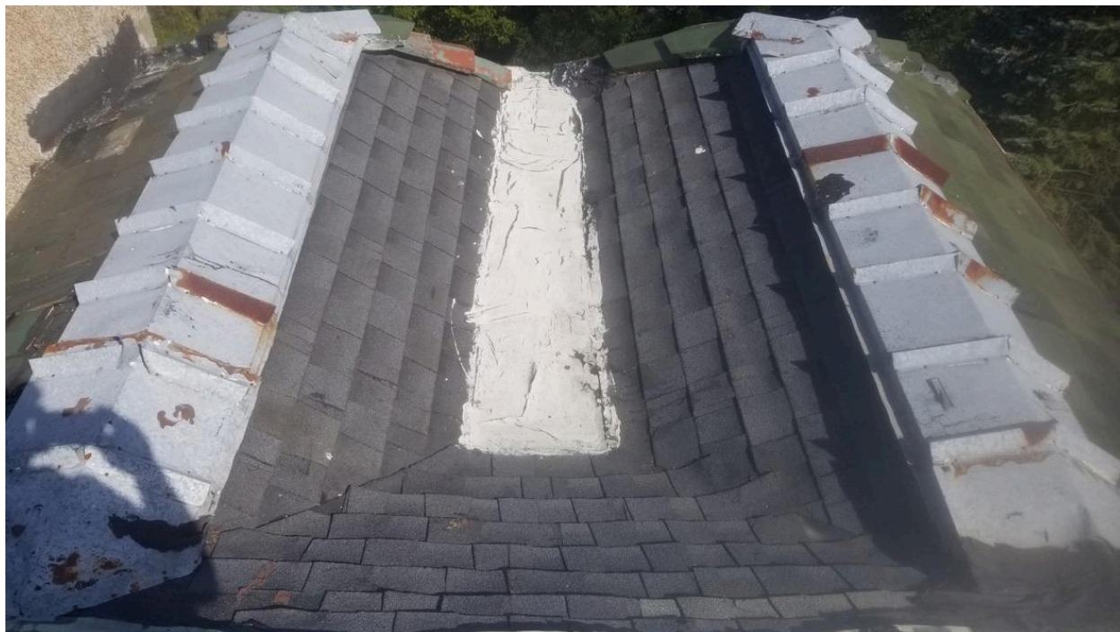
Front double hip dormers have been repaired with asphalt shingles, metal ridge caps, elastomeric coating and red clay tiles that were painted to match but now show red
