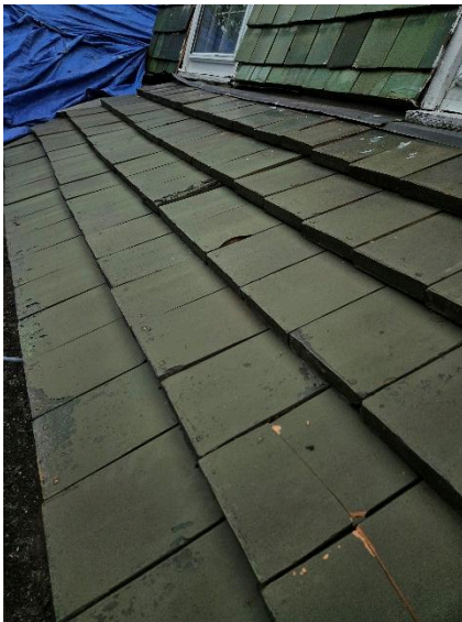
broken tiles in front of shed dormer. Rusted flat roof combing.
