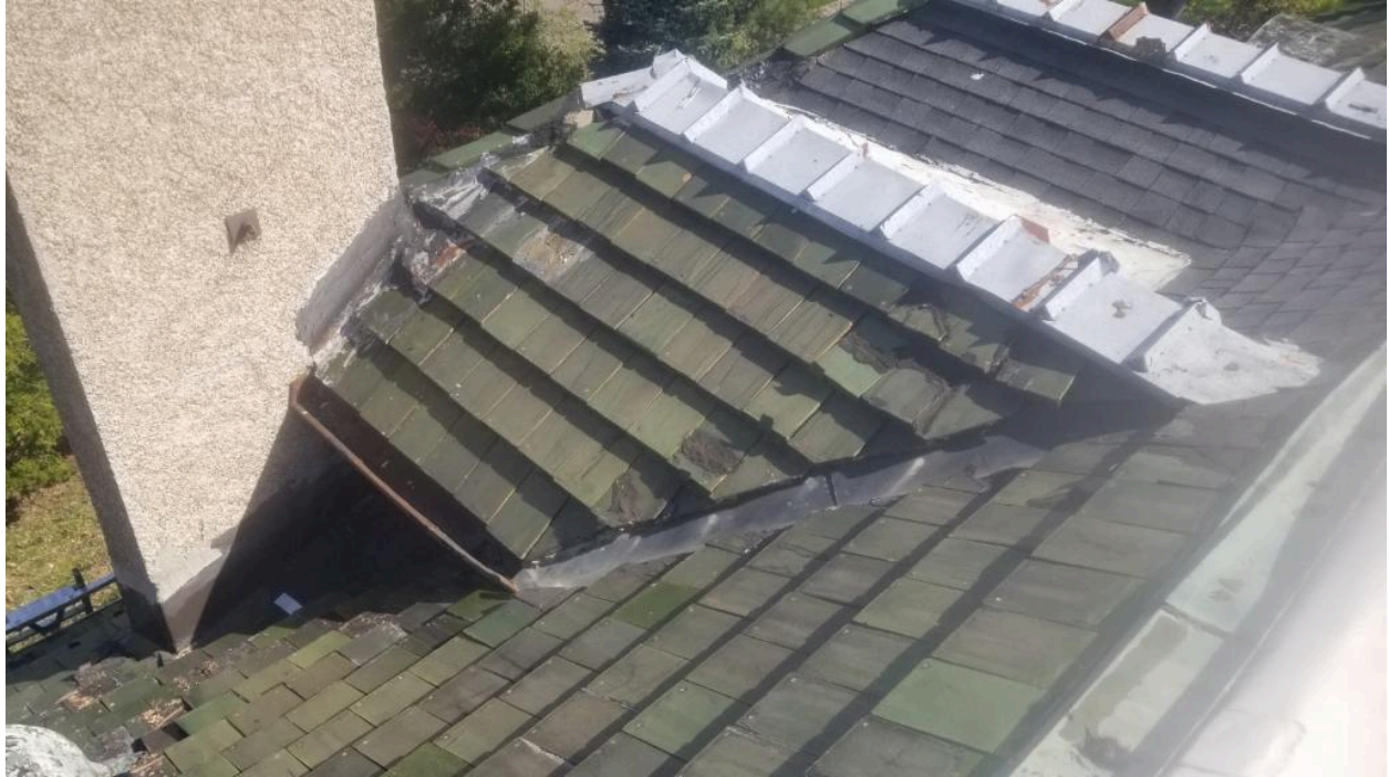
Faulty flashing & valley, rusted gutter, many broken tiles behind the front chimney west side of double dormer
