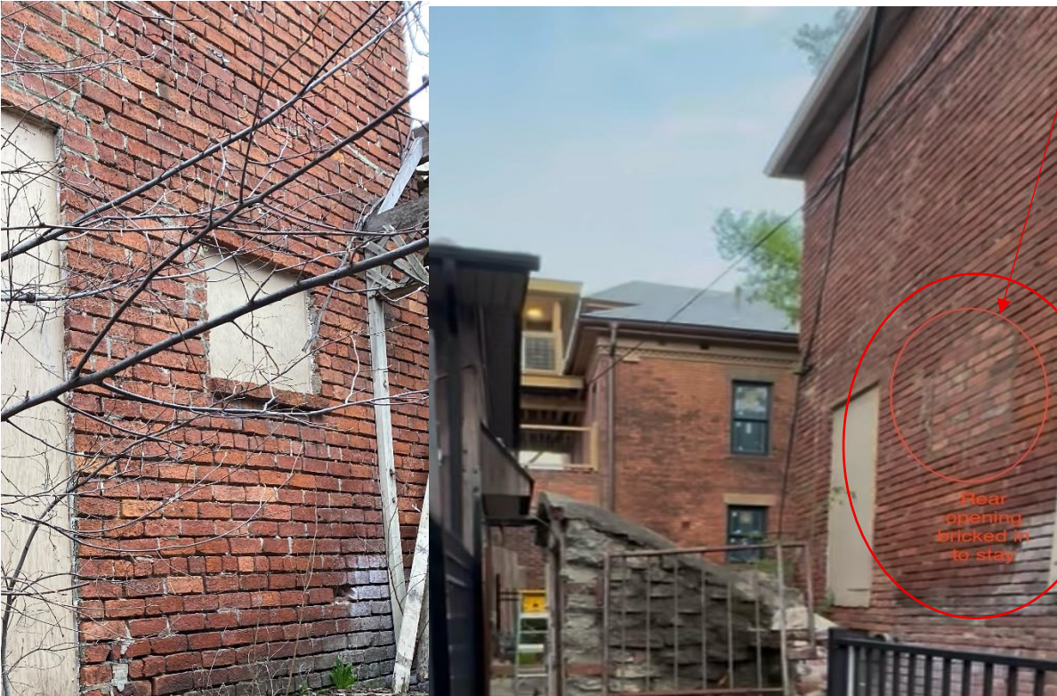
Bricked in opening South Face
