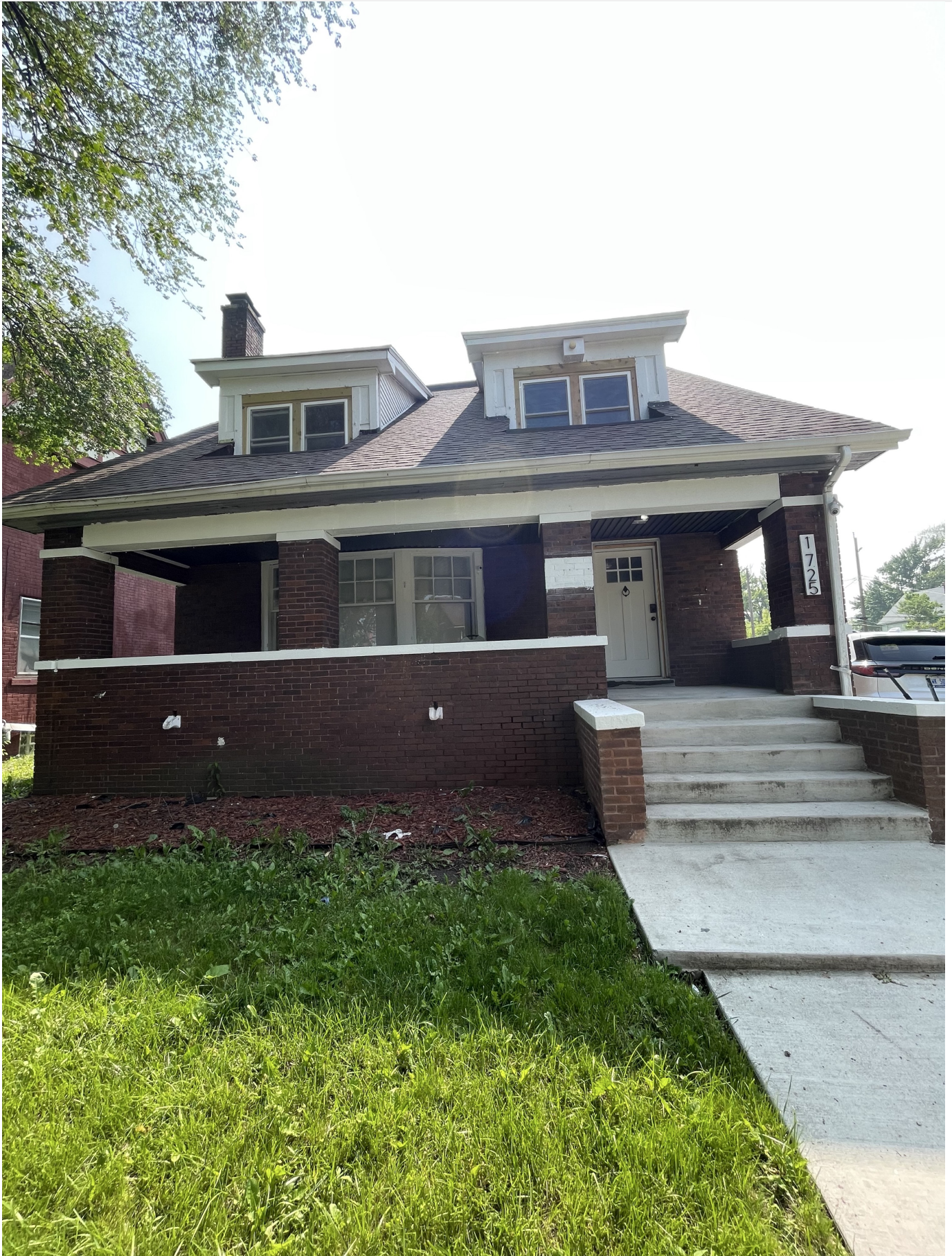
Photo 3 - Front Elevation with New Top Windows (30"x55")
