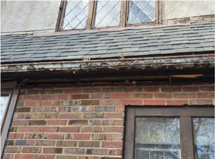
FASCIA/TRIM/GUTTER REPAIRS
