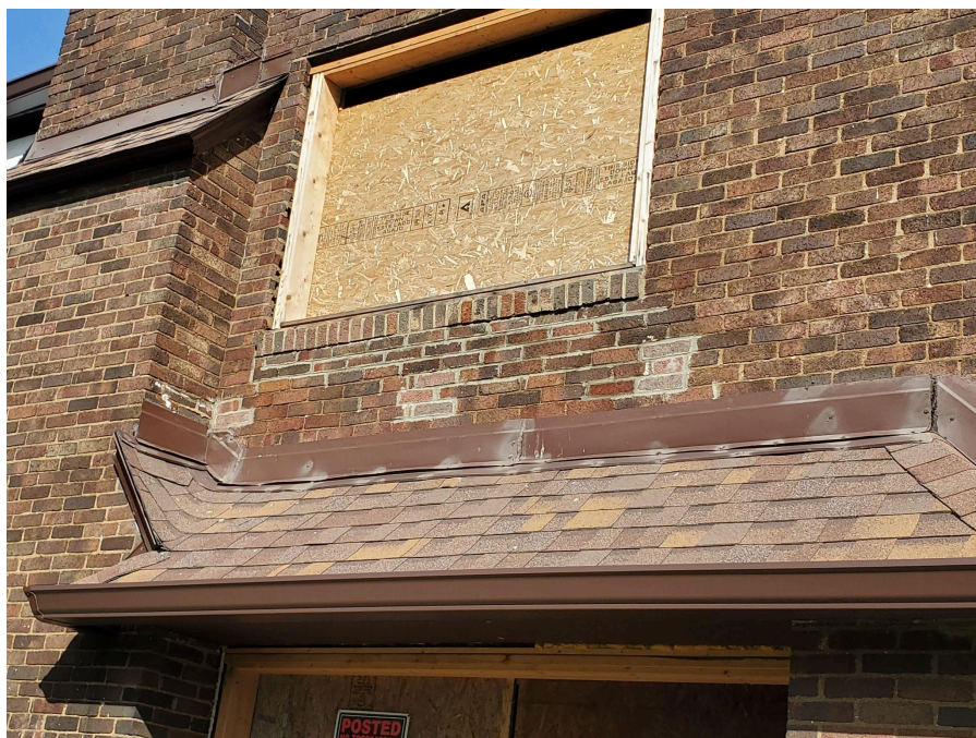
South Elevation, Brick Tuckpointing/Repair Required (typical detail) (cont'd)
