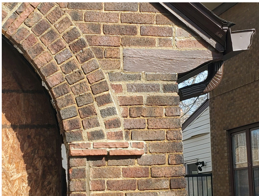
South Elevation, Brick Tuckpointing/Repair Required (typical detail)
