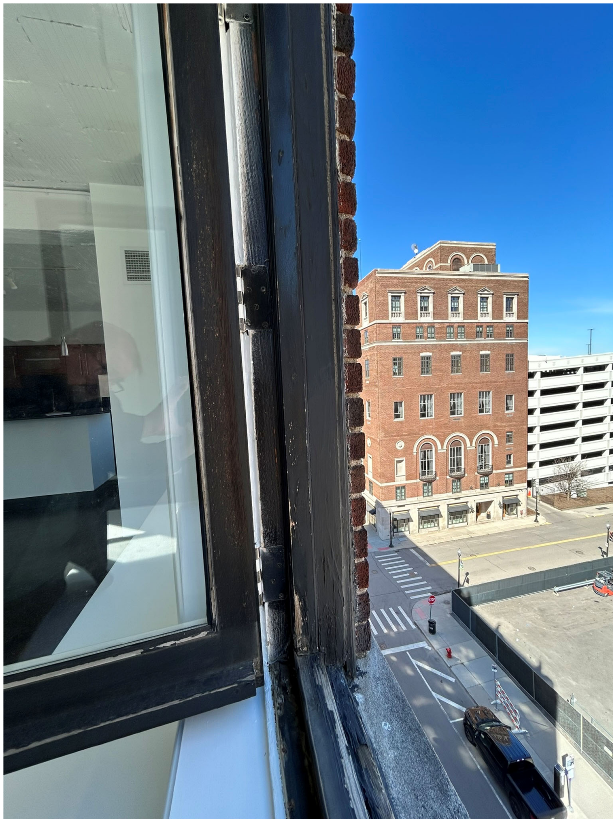
View of existing widow jamb and sash
