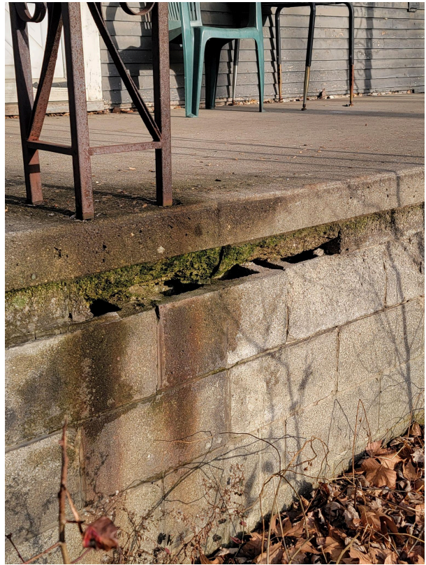
Typ. Damage to Front Porch
