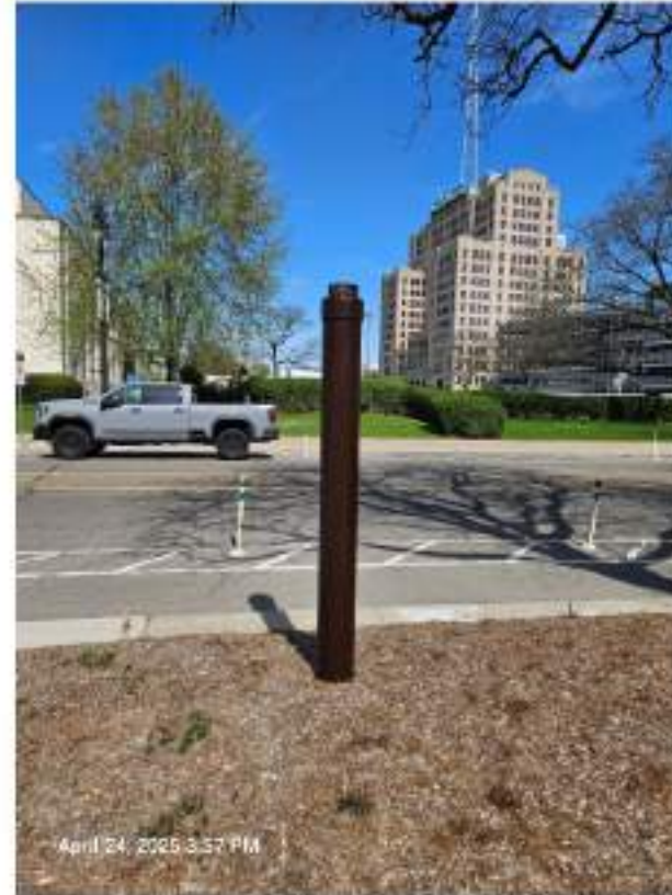
Example Detroit Thermal Venting Installation
