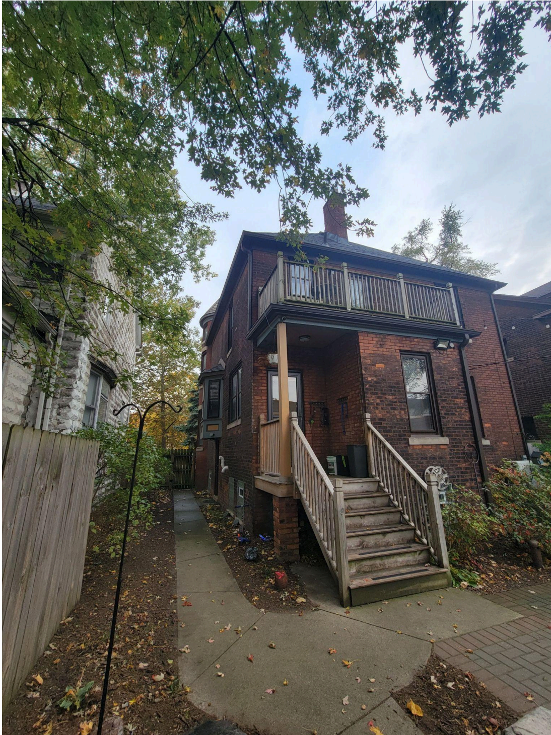
East/Partial South View
