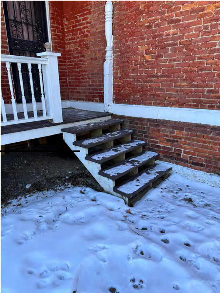
These steps are not original or historic. They are painted, pressure treated, exterior grade 2x members
